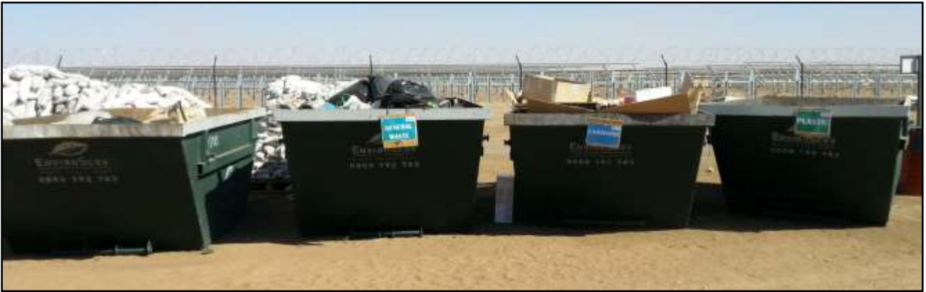
Image 2: Example of marked recycling skips within a site camp
