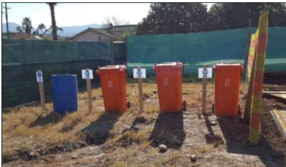
Image 1: Example of marked recycling bins within a site camp
