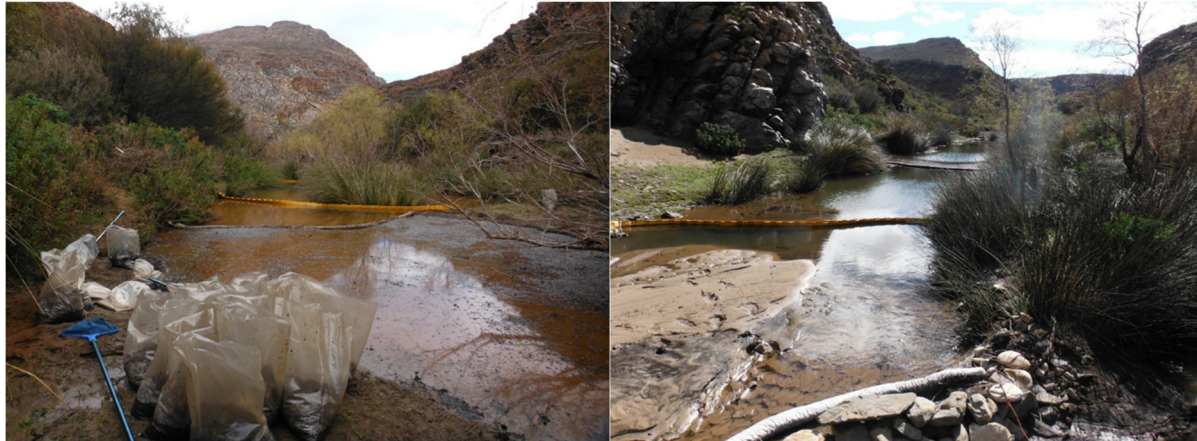
Figure 6: Containment berms and clean-up of contaminated soil (left) and furthest downstream containment berm (right)
