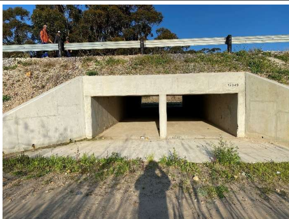
Box culvert 12349 as seen from the west of the road towards the east (upstream).
