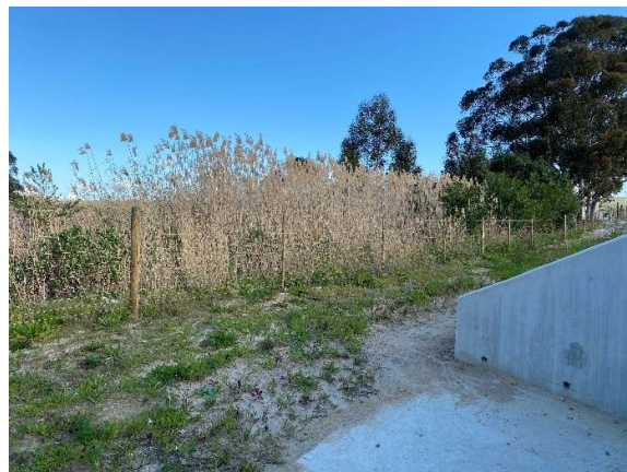
Upstream towards the east as seen from box culvert 12349.
