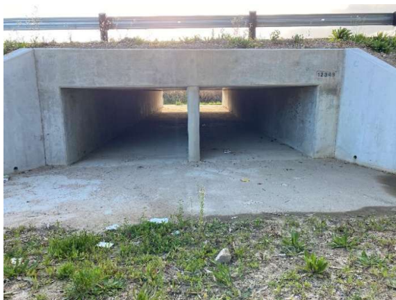
Box culvert 12349 as seen from the east towards the west (downstream).
