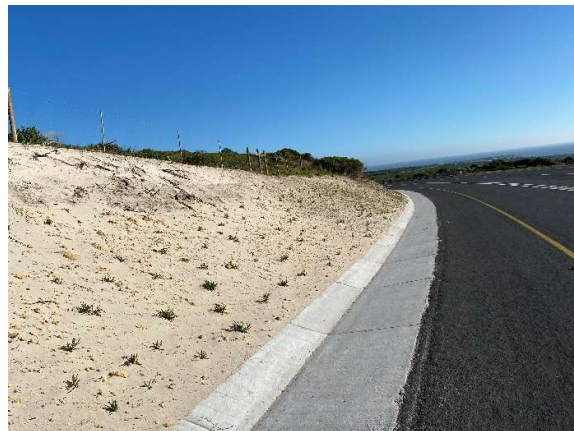
Completed planting and rehab along the sandy exposed slopes as seen towards the south.
