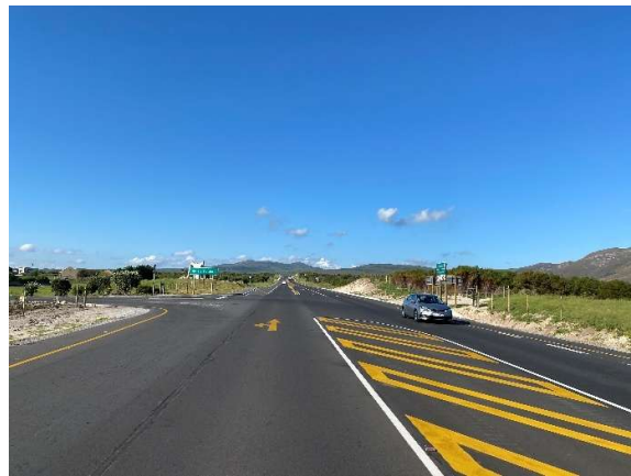
The upgraded intersection at the De Kelders turnoff at km 40.
