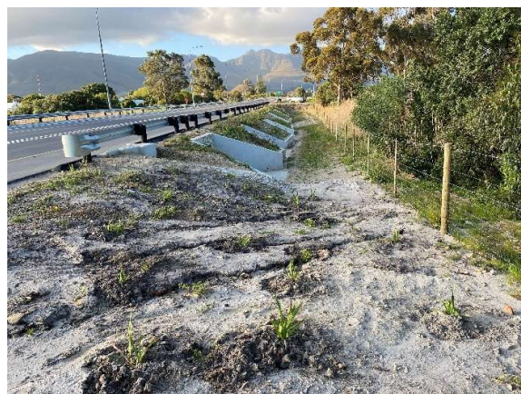
Completed landscaping along the road shoulder towards the south of the completed box culverts at km24.
