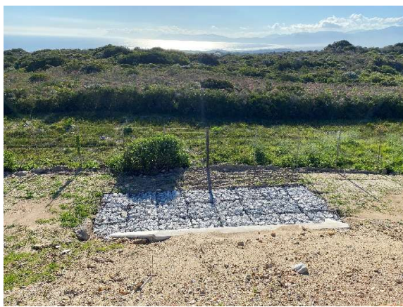
Completed culvert with headwall and reno mattress downstream at km 36.
