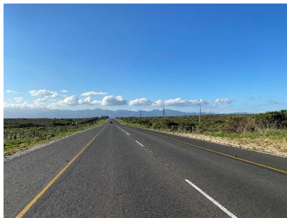
Completed road surface near km 33 seen towards the north.
