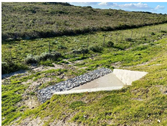
Completed culvert with headwall and mattress downstream at km 35 as seen from the road shoulder towards the northwest.
