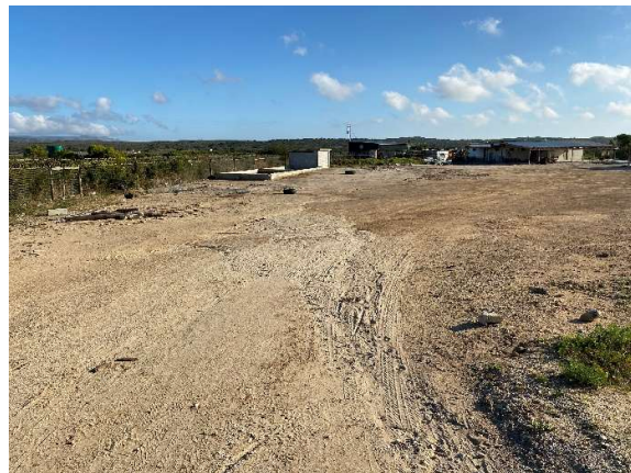
The condition of the site camp. Some infrastructure improvements were retained on request of the landowner.
