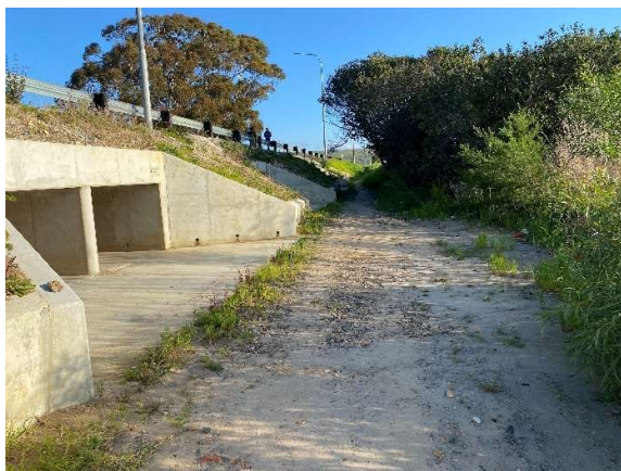
Box culvert 12350 as seen from the west of the road towards the south.
