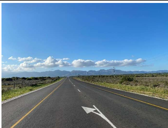
Completed road surface near km 29 seen towards the north.
