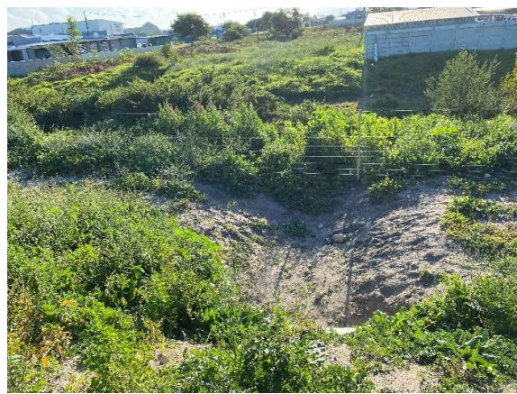
Pipe culvert with headwall completed along the west of the road at km25 as seen towards the west.
