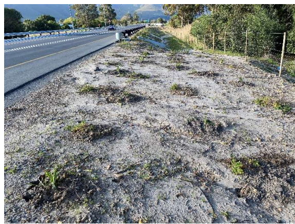
Completed rehabilitation along the eastern road shoulder at km24.
