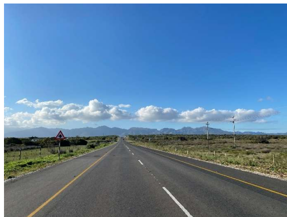
Completed road surface near km 28 seen towards the north.
