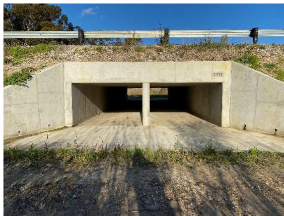
Box culvert 12350 as seen from the west of the road towards the east (upstream).
