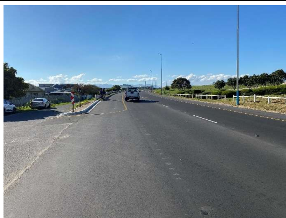
Near the end of the contract at the entrance into Gansbaai at km 43.
