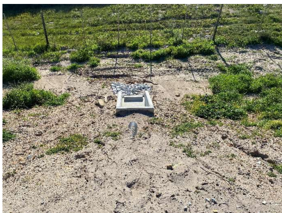
Completed culvert outlet with litter trap and mattress downstream at km 36.
