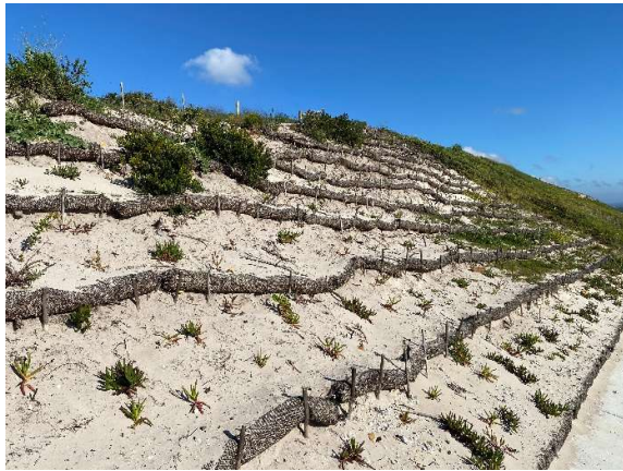
Completed large scale rehabilitation at the larger and steeper cuttings along the R43 at km 3.
