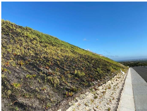
Completed large scale rehabilitation at the larger and steeper cuttings along the R43.
