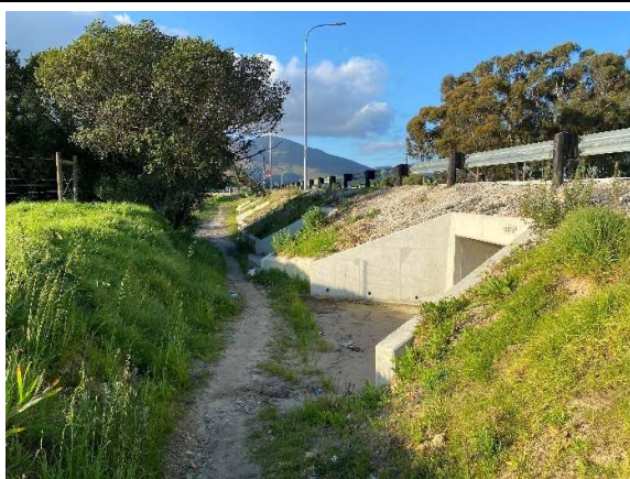
Along the west of the completed box culverts at km24 as seen towards the north.
