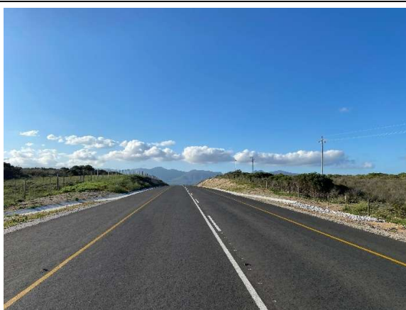
Completed road surface near km 30 seen towards the north.
