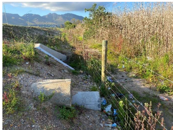
Pipe culvert with headwall completed and another pipe culvert retained along the east of the road at km25 as seen towards the north.
