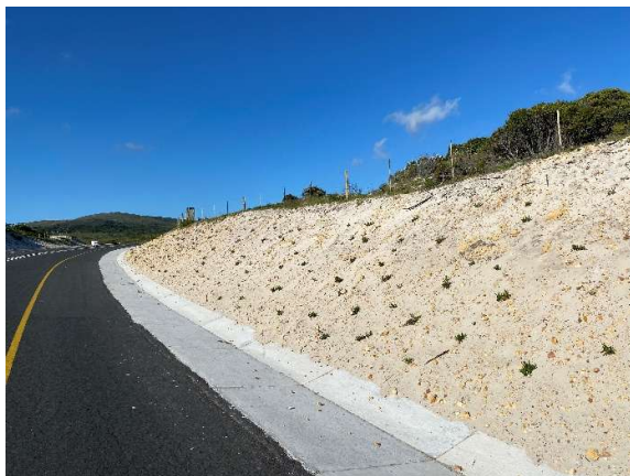
Completed planting and rehab along the sandy exposed slopes as seen towards the north.
