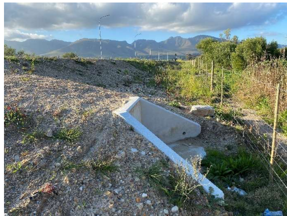
Pipe culvert with headwall completed along the east of the road at km25 as seen towards the north.
