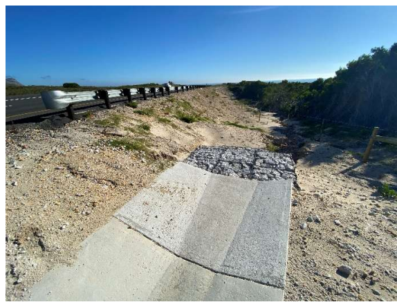
Completed sidedrain channel outlets @km 37 with gabions at the outlet for energy dissipation to prevent erosion.
