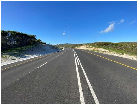
Completed road surface near km 37 seen towards the north.
