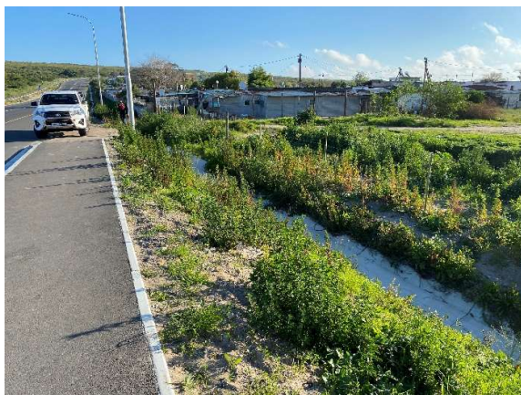
Side drains completed along the west of the road at km25.
