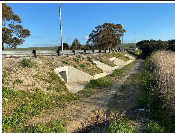
Along the west of the completed box culverts at km24 as seen towards the south.
