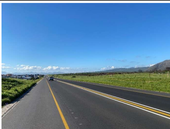
Completed road surface near km 42 seen towards the north.
