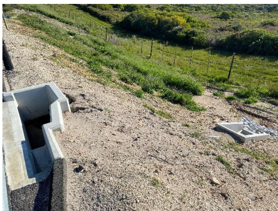
Road shoulder catchment inlet with culvert outlet downstream at km 36.
