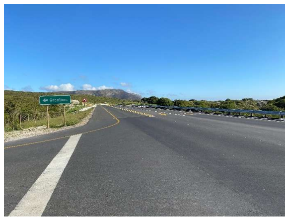
Completed upgraded intersection with dedicated turn lanes at the Grootbos Nature Reserve at km 36.
