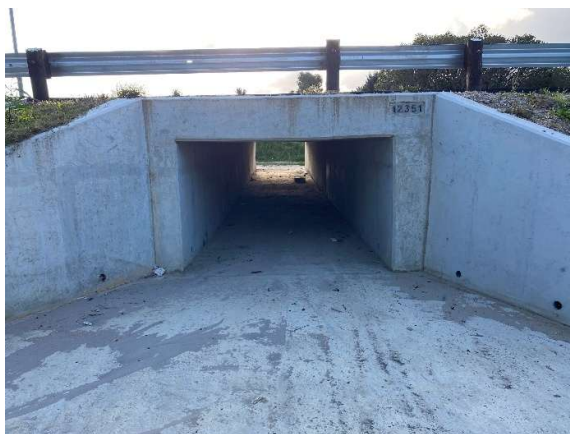
Box culvert 12351 as seen from the east towards the west (downstream).
