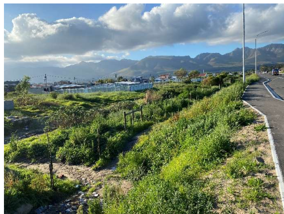
Pipe culvert with headwall completed along the west of the road at km25 as seen towards the north.
