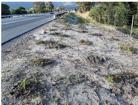
Completed landscaping along the road shoulder towards the south of the completed box culverts at km24.
