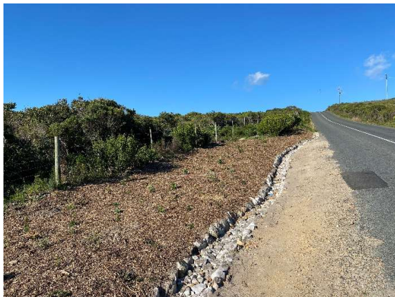
Completed planting and rehab at the Grootbos turnoff complete with stone pitched stormwater drainage.
