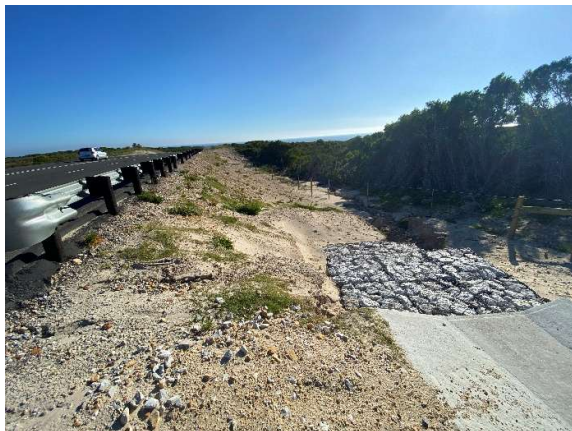
Completed sidedrain channel outlets @km 37 with gabions at the outlet for energy dissipation to prevent erosion.
