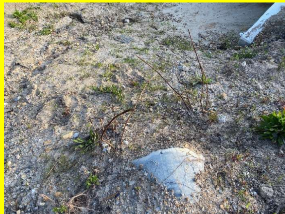
Some steel reinforcement along the east of the new box culverts which need to be removed.
