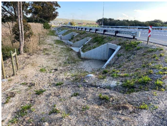
The current condition along the eastern upstream end of the completed box culverts at Km 24 as seen towards the south.
