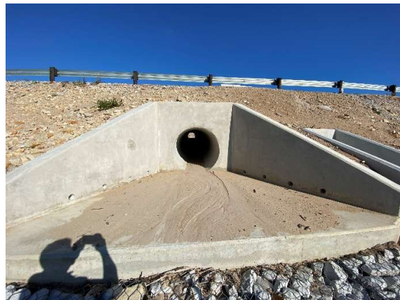
Completed culvert outlet with wingwall and mattress downstream at km 37.84
