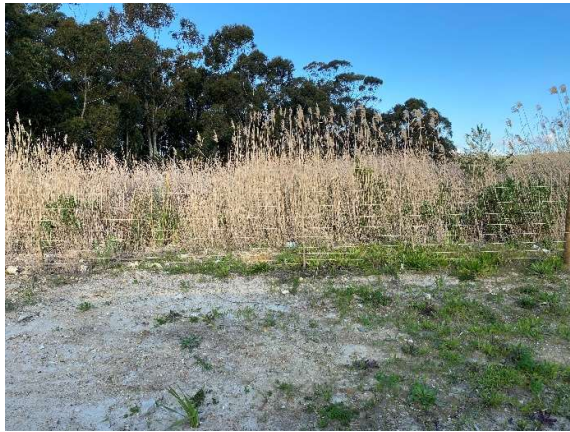
Upstream towards the east as seen from box culvert 12350.
