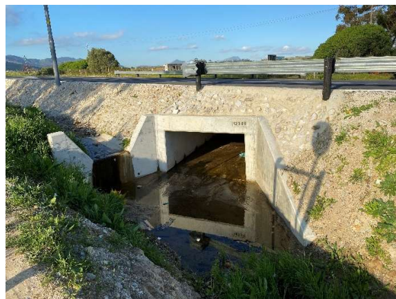
Box culvert 12340 along the west of the road as seen towards the north at km24.
