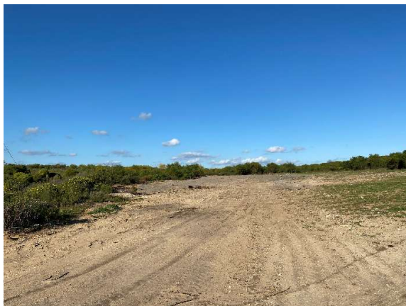
Stockpile area 2, at approximately km 27.5 where all stockpiled material has been removed and the area ripped.
