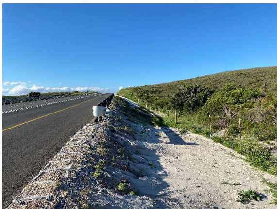
Completed culvert with headwall upstream at km 36 as seen towards the north.
