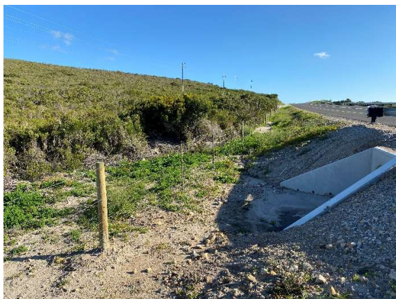
Completed culvert with headwall upstream at km 35 as seen towards the south.
