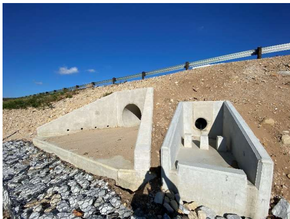
Completed culvert outlet with wingwall and mattress and litter trap downstream at km 37.84.
