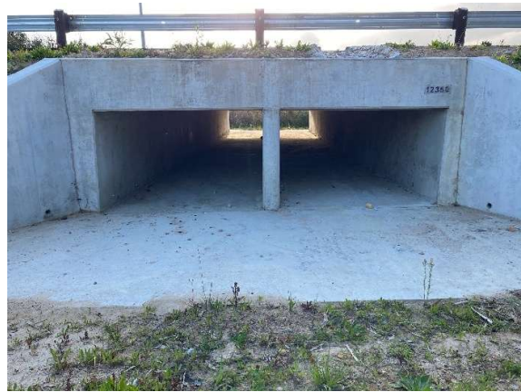
Box culvert 12350 as seen from the east towards the west (downstream).
