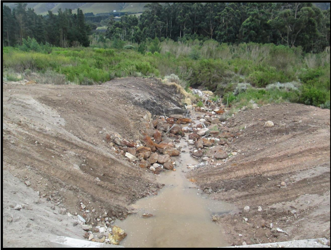
Figure 24: Culvert Rehabilitation carried out by GNEC.
