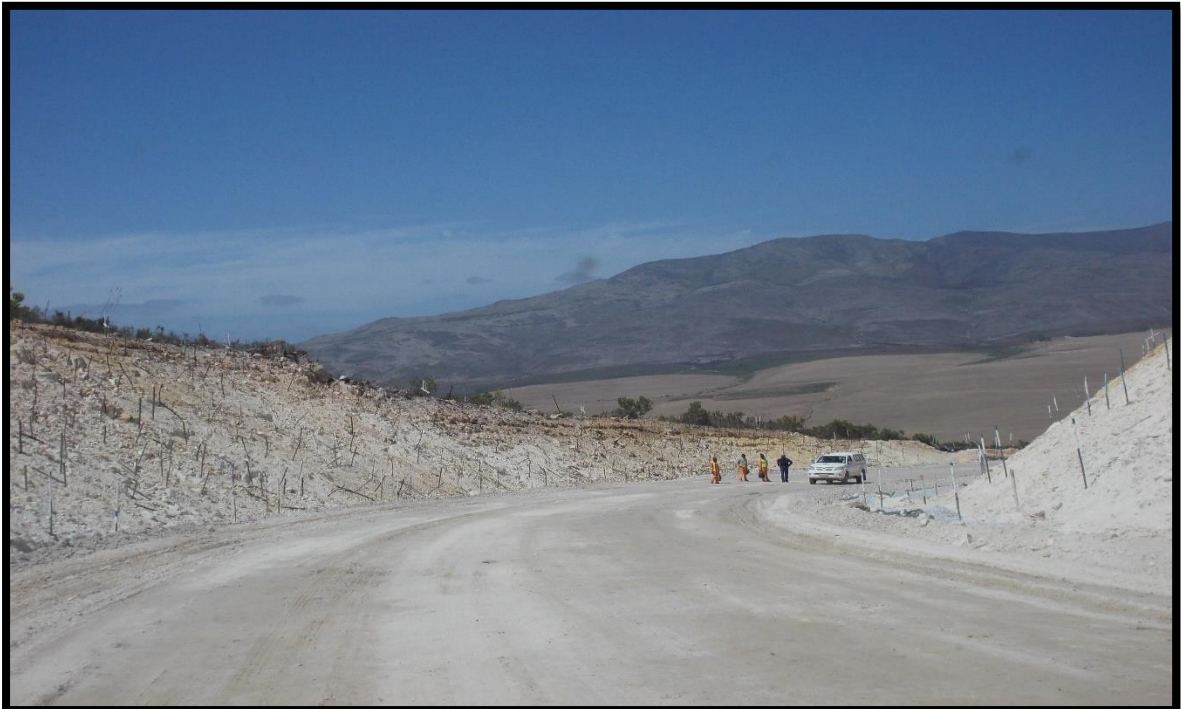
Figure 34: Embankment Rehabilitation carried out by GNEC.
