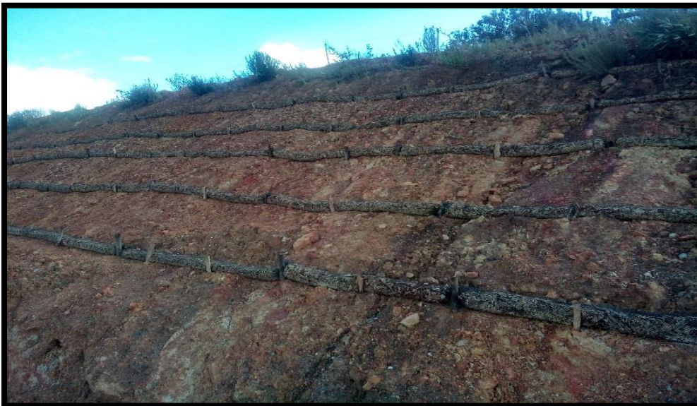
Figure 12: Example of horizontal terracing with biodegradable sausages to reduce down slope erosion.
