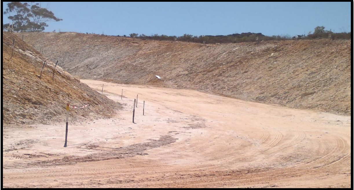
Figure 33: Embankment Rehabilitation carried out by GNEC.
