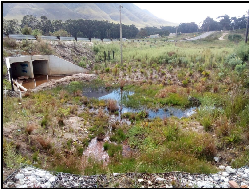
Figure 17: Culvert Rehabilitation carried out by GNEC.
