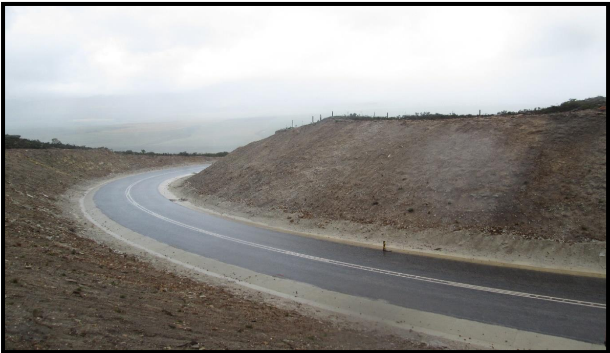
Figure 36: Embankment Rehabilitation carried out by GNEC.
