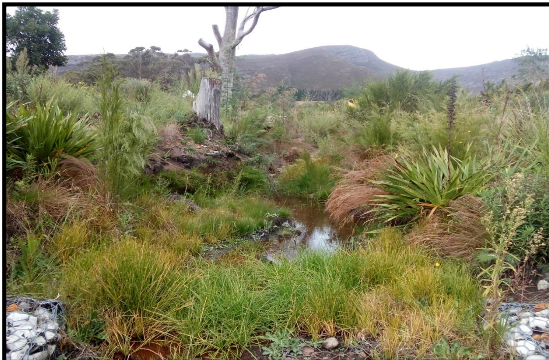
Figure 20: Culvert Rehabilitation carried out by GNEC.
