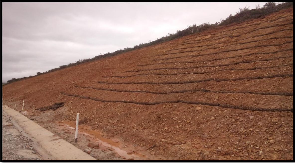
Figure 39: Embankment Rehabilitation carried out by GNEC.
