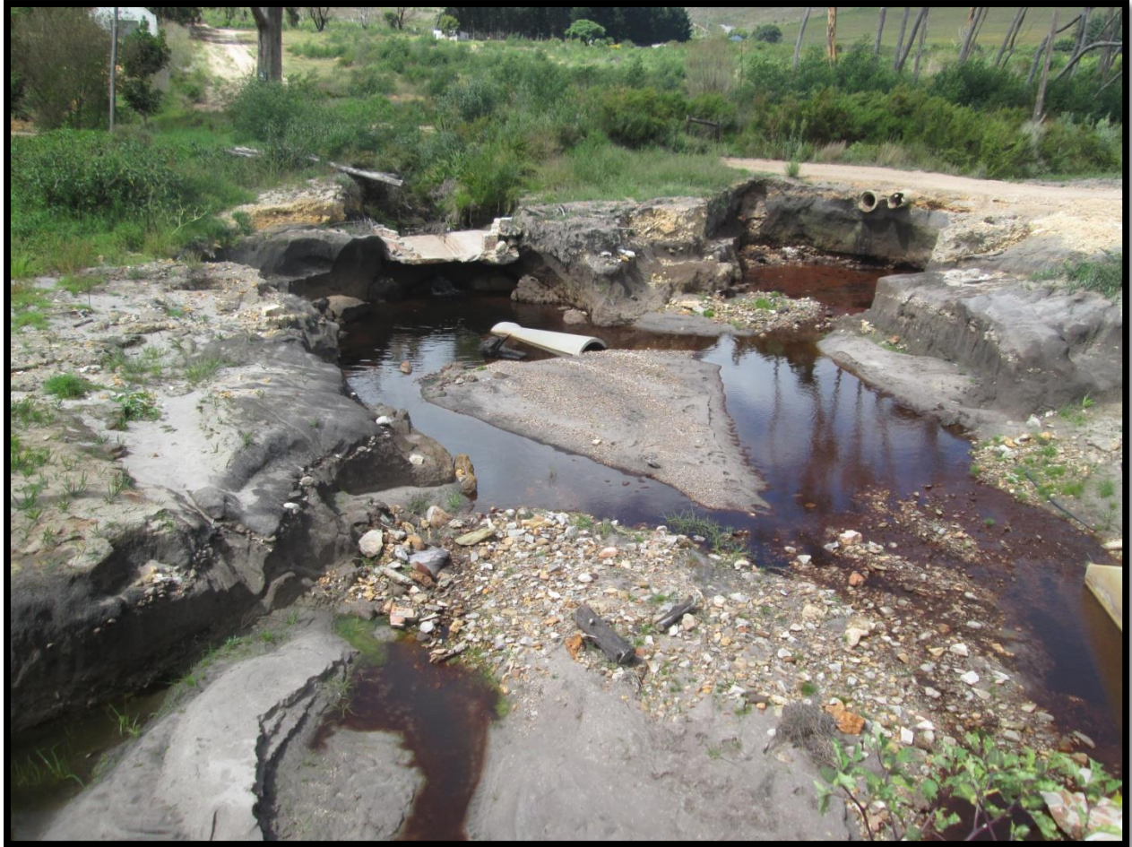
Figure 14: Culvert Rehabilitation carried out by GNEC.
