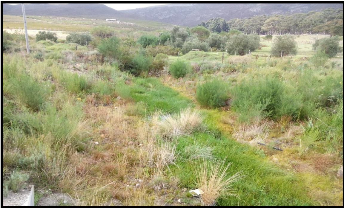
Figure 26: Culvert Rehabilitation carried out by GNEC.
