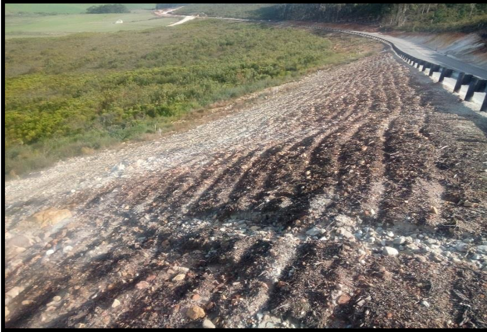
Figure 11: Example of horizontal terracing to reduce down slope erosion.
