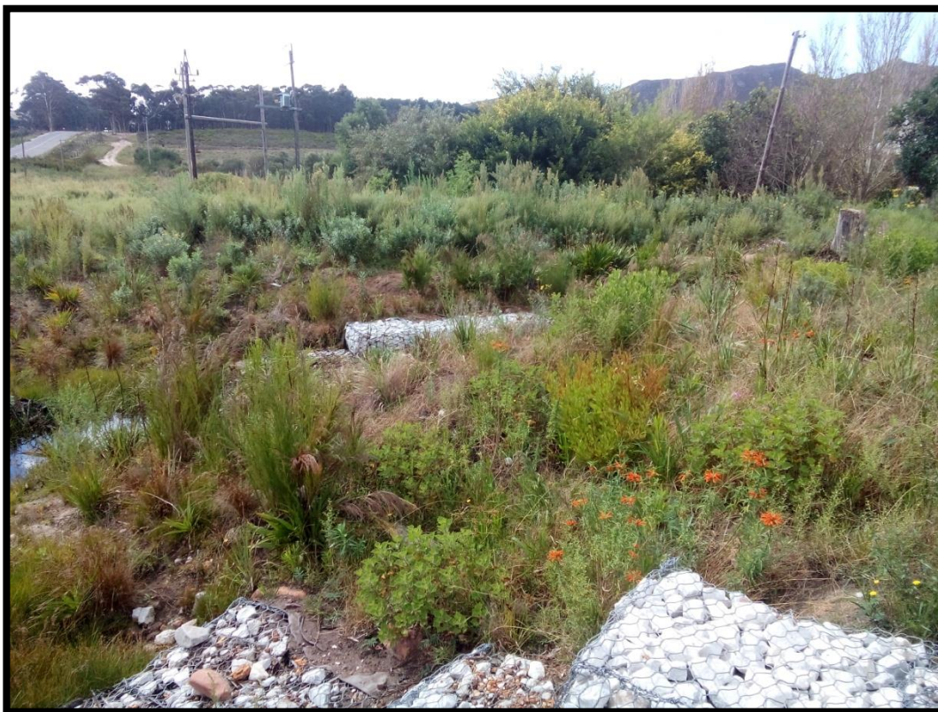
Figure 18: Culvert Rehabilitation carried out by GNEC.
