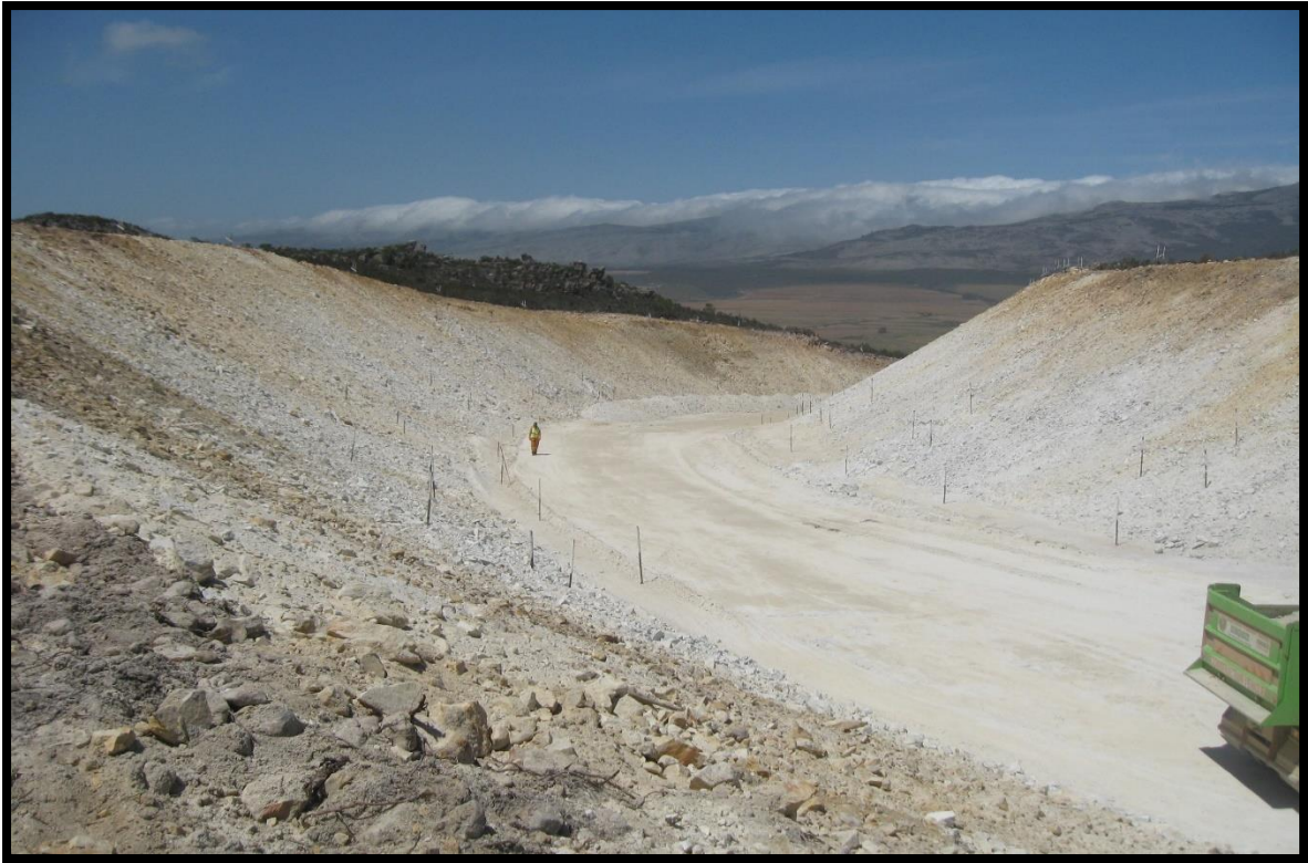
Figure 35: Embankment Rehabilitation carried out by GNEC.
