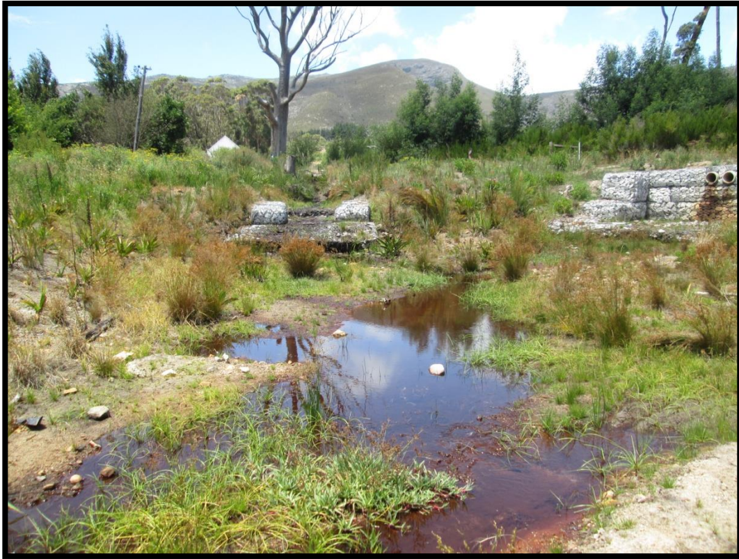
Figure 15: Culvert Rehabilitation carried out by GNEC.
