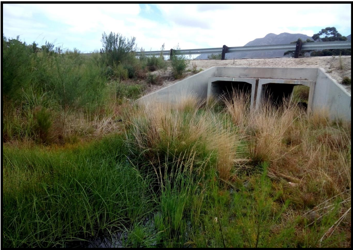
Figure 30: Culvert Rehabilitation carried out by GNEC.
