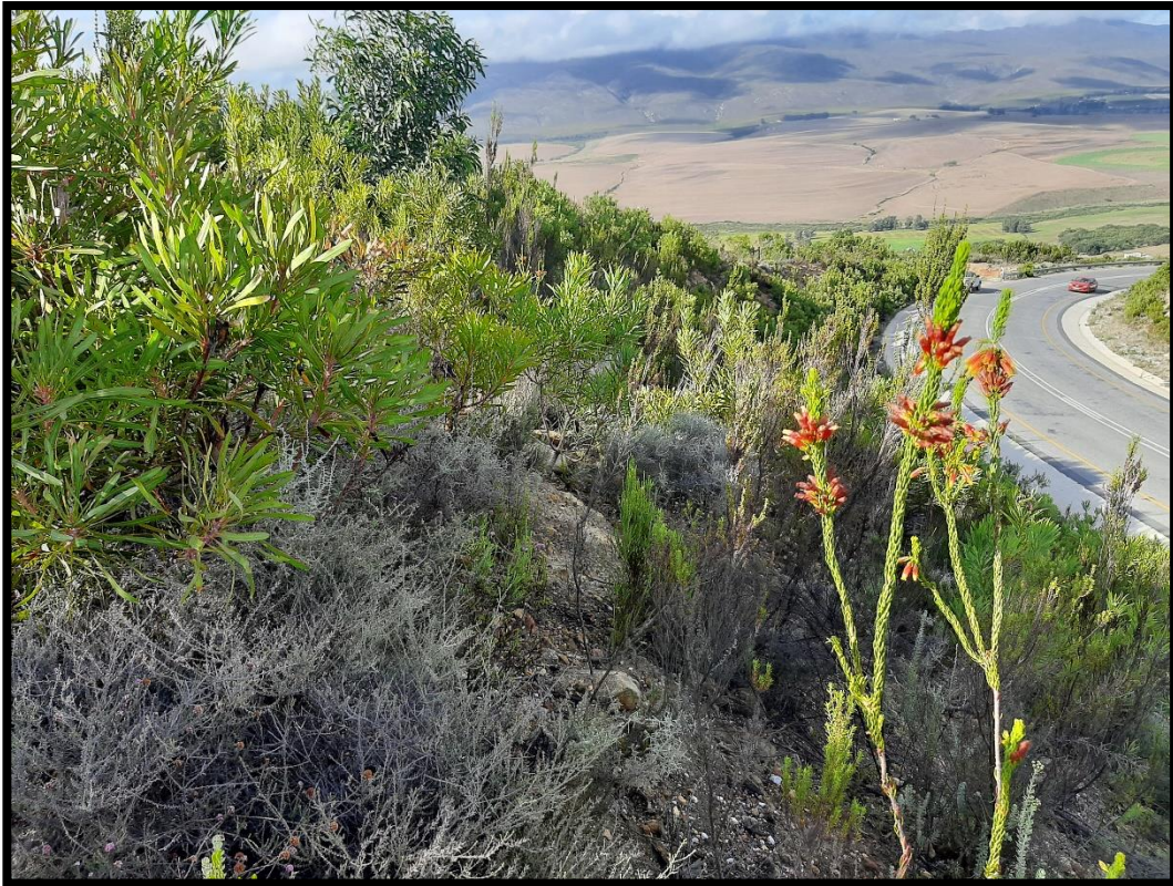
Figure 44: Embankment Rehabilitation carried out by GNEC.
