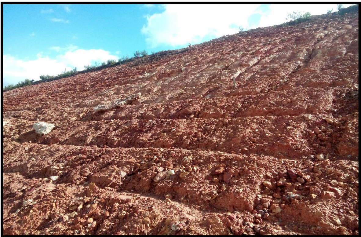
Figure 38: Embankment Rehabilitation carried out by GNEC.
