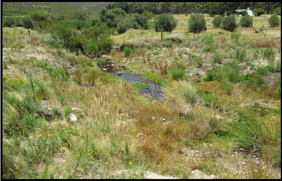
Figure 25: Culvert Rehabilitation carried out by GNEC.
