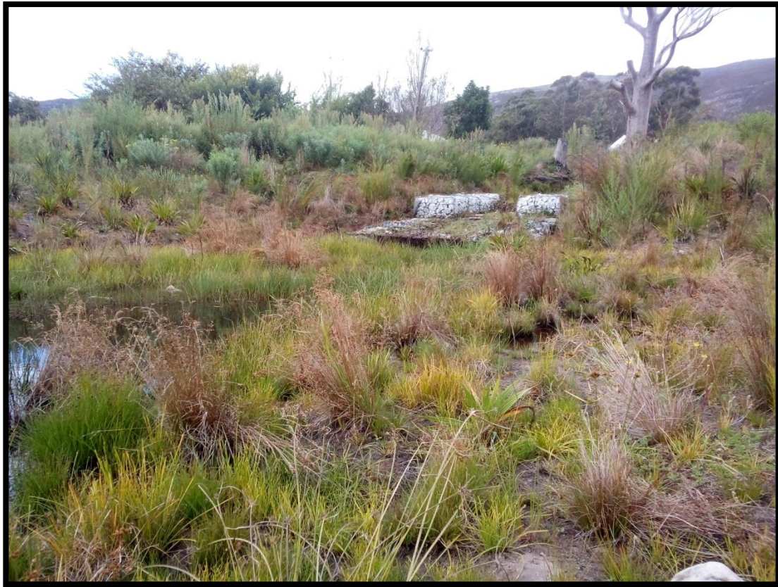
Figure 21: Culvert Rehabilitation carried out by GNEC.
