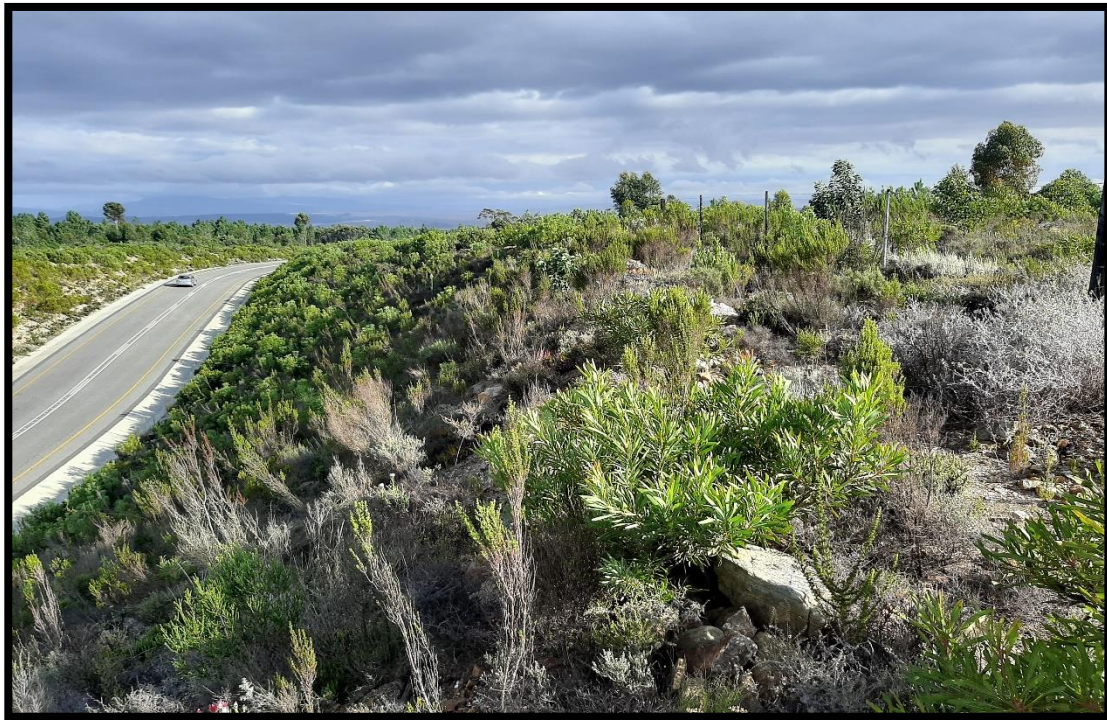
Figure 40: Embankment Rehabilitation carried out by GNEC.
