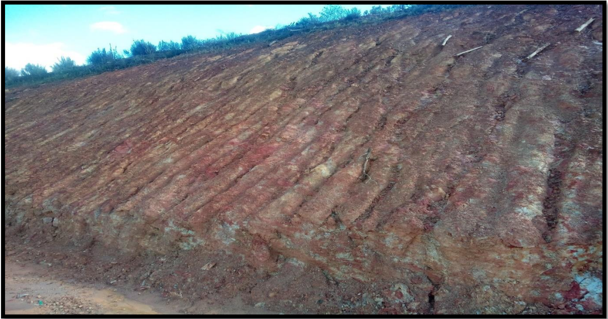
Figure 37: Embankment Rehabilitation carried out by GNEC.
