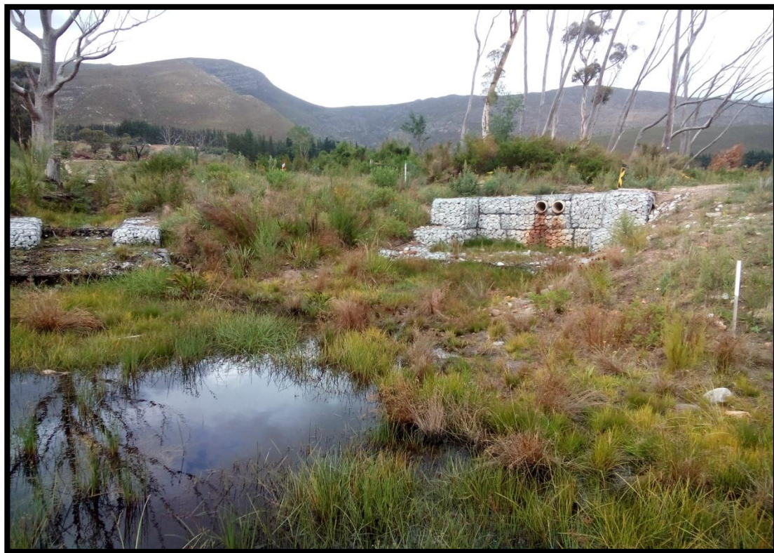
Figure 22: Culvert Rehabilitation carried out by GNEC.
