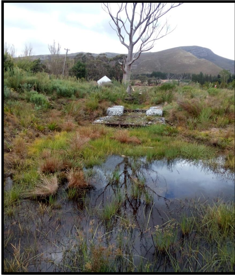
Figure 23: Culvert Rehabilitation carried out by GNEC.
