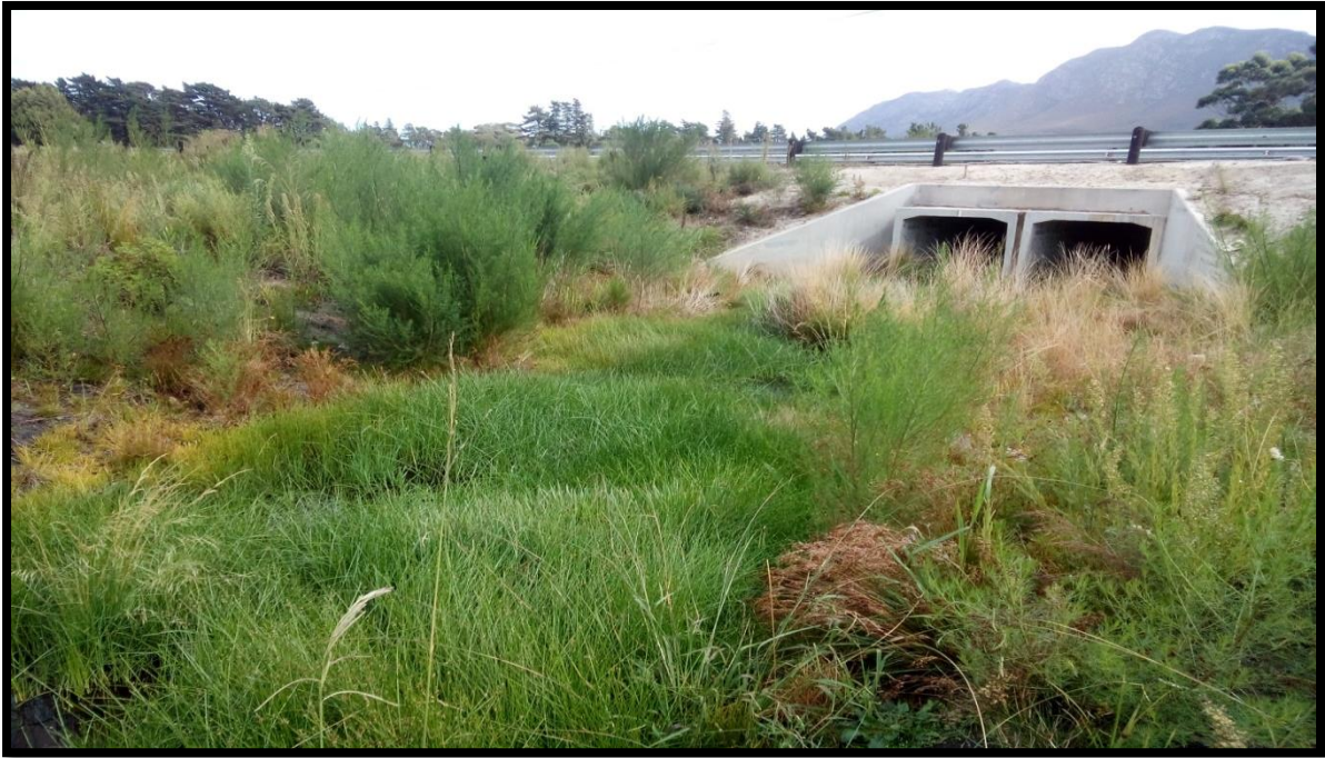
Figure 31: Culvert Rehabilitation carried out by GNEC.
