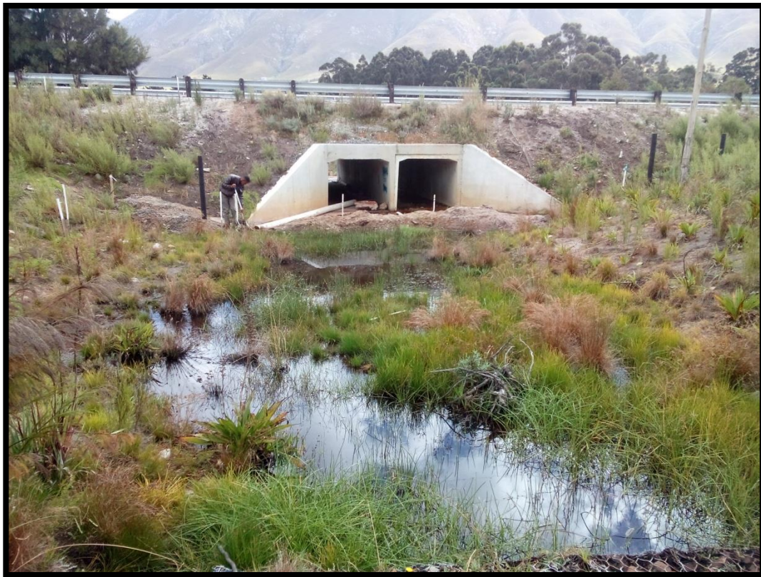
Figure 19: Culvert Rehabilitation carried out by GNEC.
