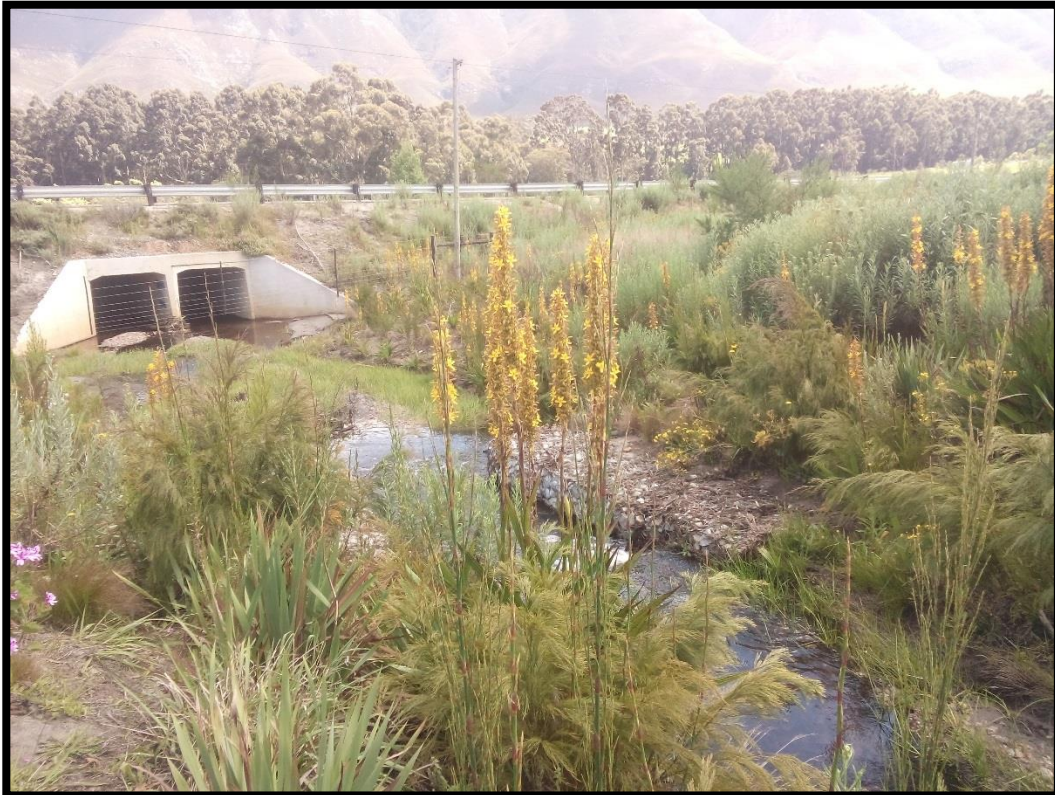
Figure 16: Culvert Rehabilitation carried out by GNEC.
