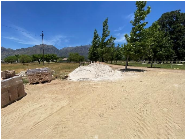
Stockpile area adjacent to the current works area towards the south of the facility.
