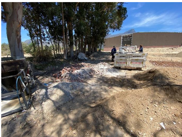
Builders rubble and waste material being loaded onto mobile skip for transportation.
