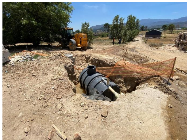
An underground sewage tank being installed immediately north of the existing facility.
