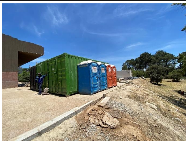
Chemical toilets available adjacent to the current works area.
