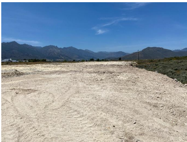
Excavated material spoil used as platform for approved future PV plant towards the northeast of the site.
