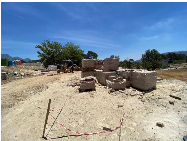
Construction laydown area adjacent Wetland B.
