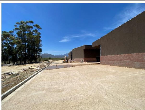
The completed extended facility as seen along its northern boundary in an eastern direction.
