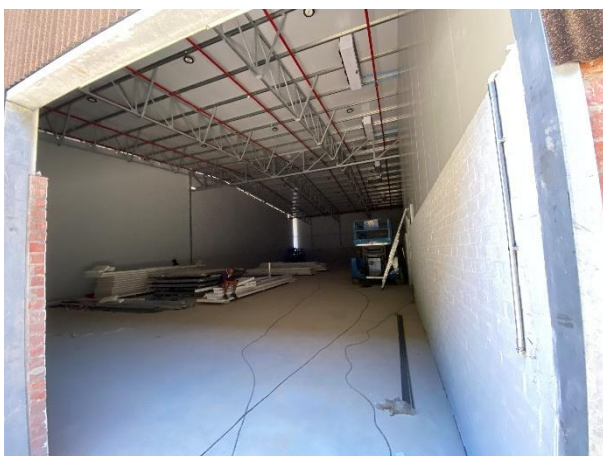
Internal section of the newly built sparkling wine facility, indicating finalised structural elements.
