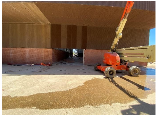
A picture demonstrating the completed extension of the existing facility.
