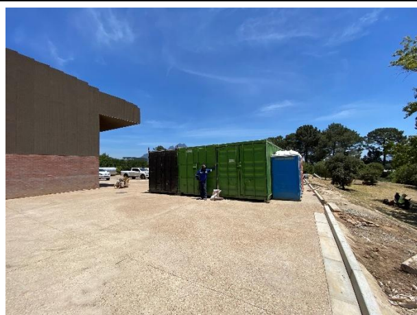
Storage container adjacent to the existing facility.
