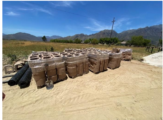
Stockpile area adjacent to the current works area.
