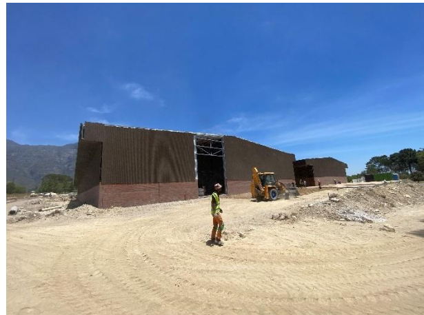
Construction progress of the facility adjacent to the new facility seen towards the southwest.
