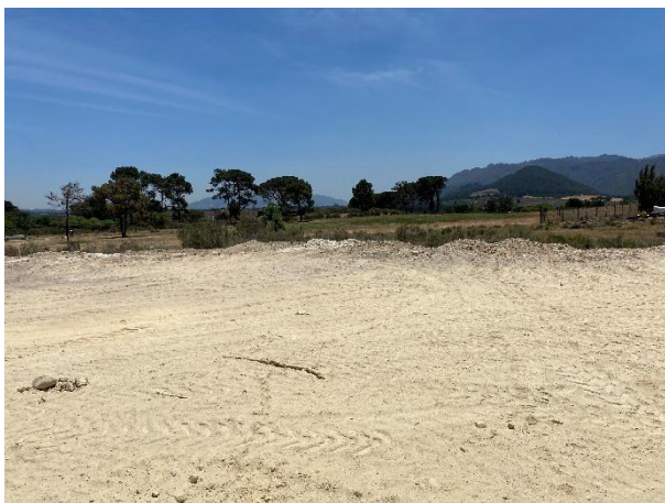
Construction access roads along the remnant fynbos section.
