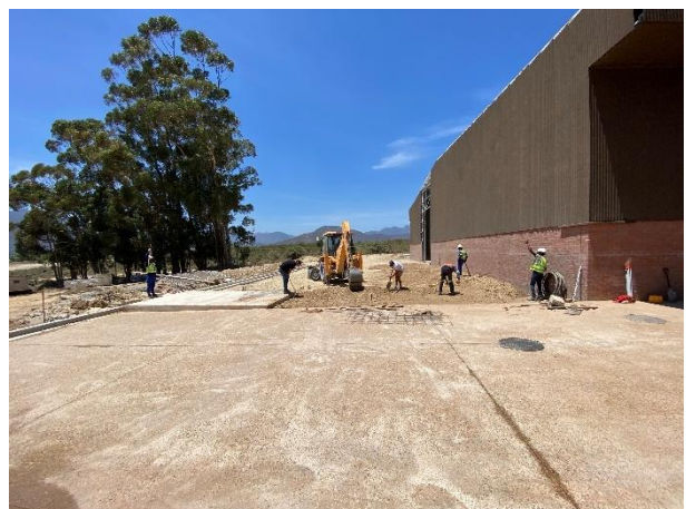
Current construction activities underway along the completed northern boundary of the facility.
