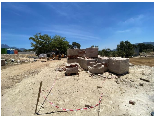
Construction laydown area adjacent Wetland B.
