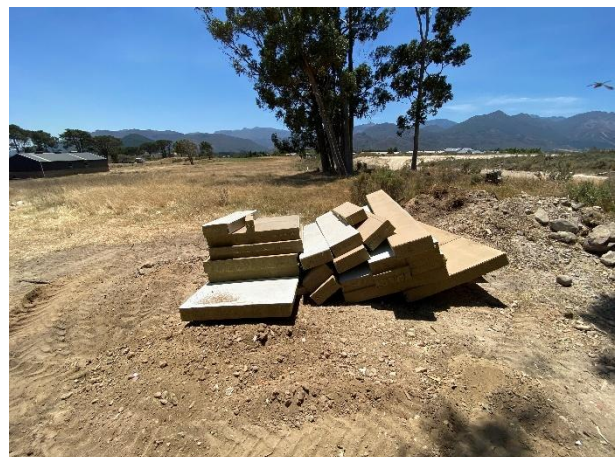
Material laydown area with Wetland B to the back of picture.
