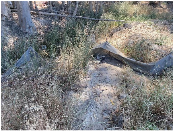
Silt fence installed along the Eucalyptus trees where a drainage line is in place adjacent Wetland B.
