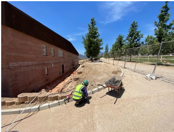
South of the newly constructed facility as seen towards the east. All tree lines have been retained.
