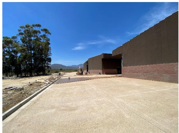
The completed extended facility as seen along its northern boundary in an eastern direction.
