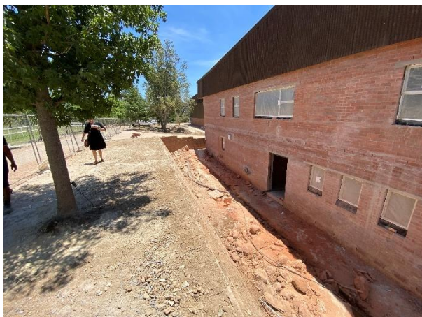
South of the newly constructed facility as seen towards the west. All tree lines have been retained.
