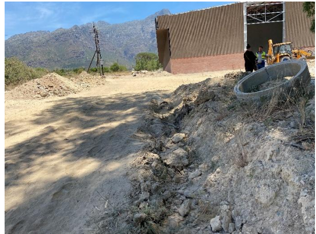
Along the Eucalyptus trees where a drainage line is in place as seen towards the south.
