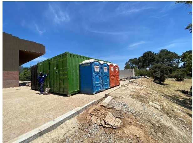
Chemical toilets available adjacent to the current works area.
