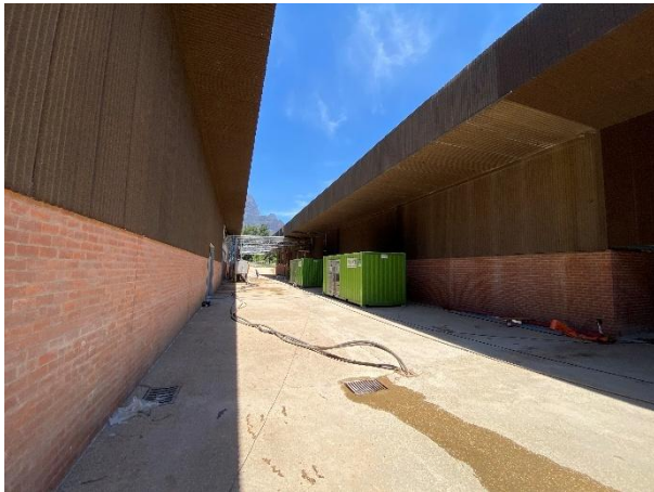
The walkthrough area between the two buildings, with the existing to the right and the new to the left.
