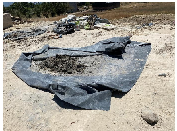
Cement batching taking place on an impermeable surface.
