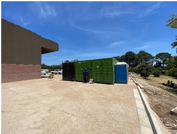
Storage container adjacent to the existing facility.
