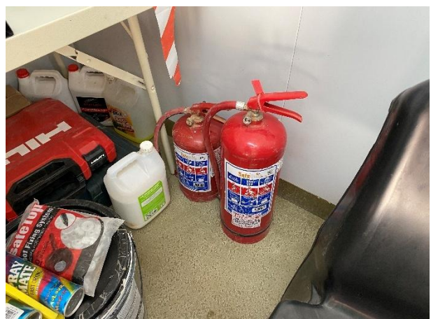
Appropriate firefighting equipment within the site office.
