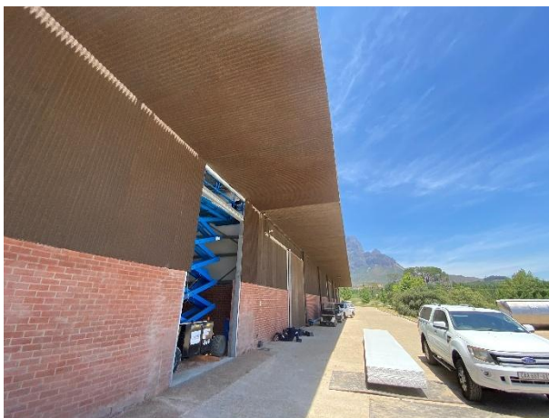
A picture demonstrating the completed extension of the existing facility as seen towards the south.
