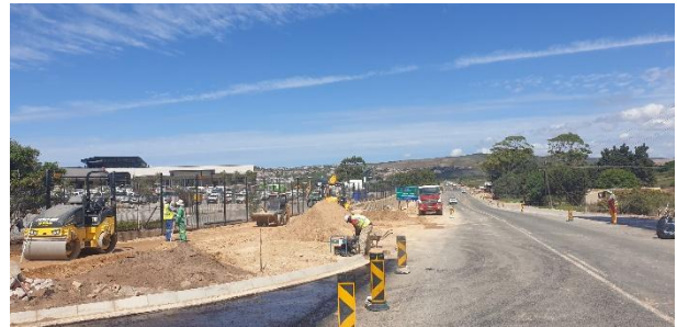
R102 being upgraded as per the municipal planning conditions for the construction of the Garden Walk Mall.
