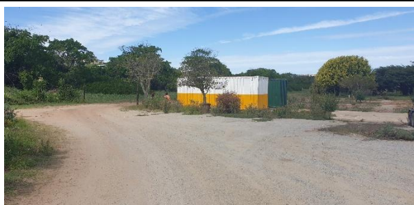
Site camp establishment within the previous Swans Nursery footprint.
