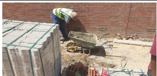
Final construction in progress along the R102.
