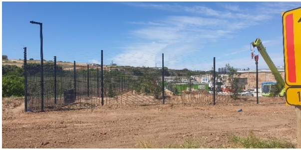
Retaining wall constructed along RE/219 boundary following unlawful clearing.
