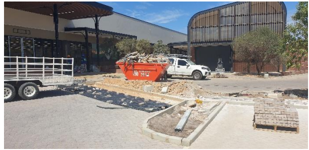
Skip in place near paving and cement works.
