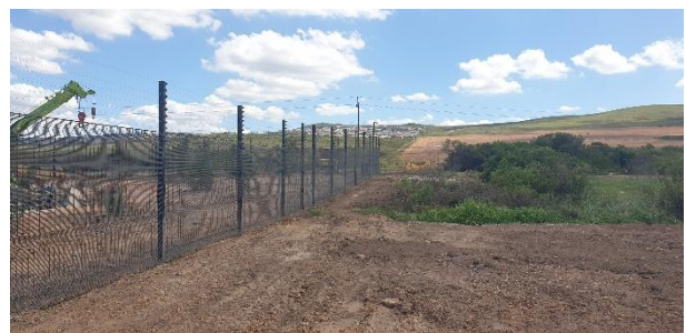
Previous site camp location within RE/219. Borderline shown to the West.
