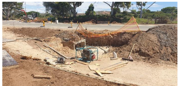
Stormwater system being installed as part of the R102 upgrade.
