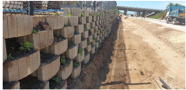
Landscaped retaining wall along the entrance of the site.
