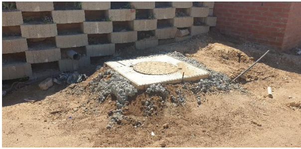
Completed stormwater services adjacent to the entrance of the site.
