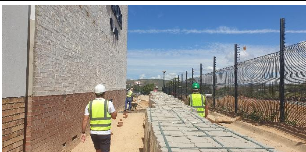
Construction boundary along the R102.
