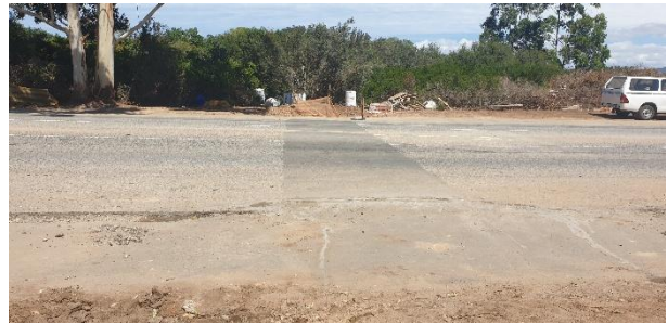
Stormwater services adjacent to the entrance of the site being installed.
