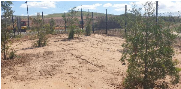
Rehabilitation Phase 3 in progress along the RE/219 boundary, on top of the retention wall.
