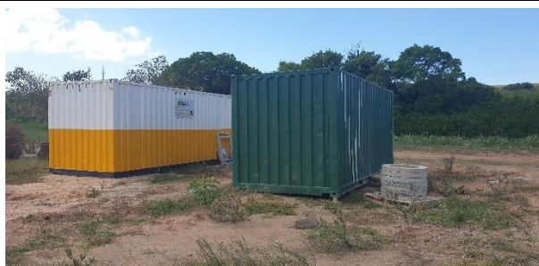
Storage containers located within the newly established site camp.
