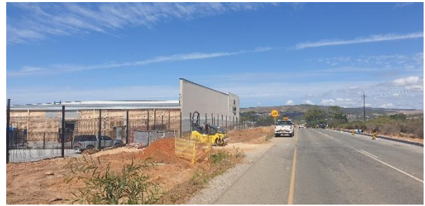
R102 being upgraded as per the municipal planning conditions for the construction of the Garden Walk Mall.
