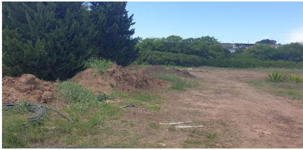
Remaining topsoil stockpiles at the site camp for rehabilitation.
