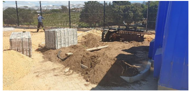
Ground preparation and material handling for paving and drainage works.
