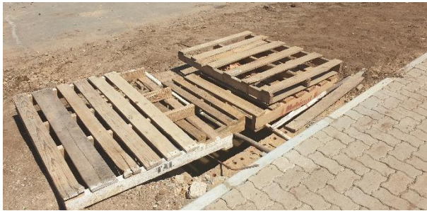
Stormwater services adjacent to the entrance of the site being installed.
