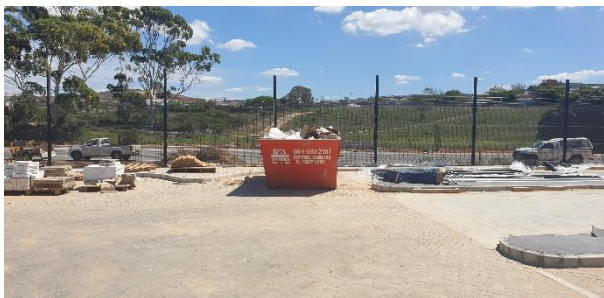
Skip available along the parking area of the construction area.
