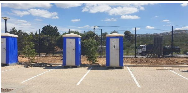
Chemical toilets available along the parking area of the Garden Walk Mall construction area.
