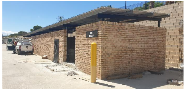
Delivery refuse yard.
