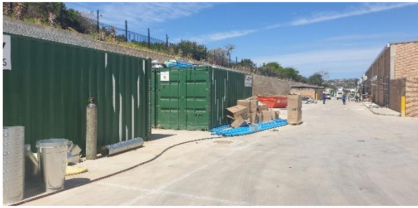
Service yard and delivery area constructed for retail tenant logistics.
