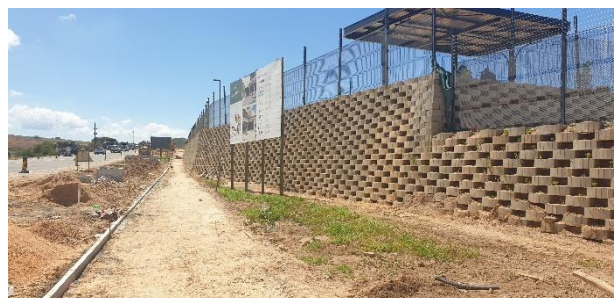
Landscaped retaining wall along the R102 boundary of the site.
