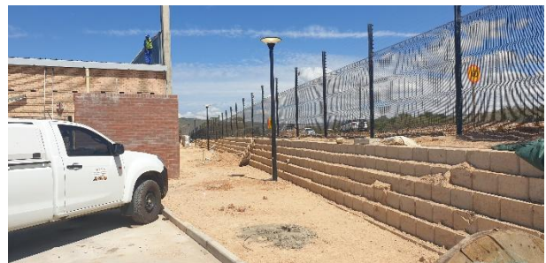
Construction boundary along the R102.
