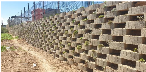
Landscaped retaining wall along the R102 boundary of the site.
