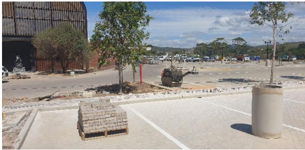
Bin in place near paving and cement works.
