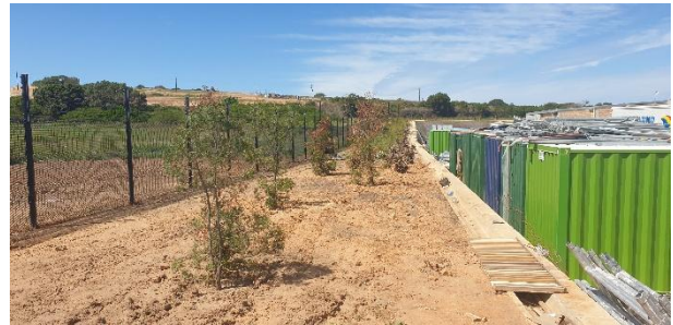
Rehabilitation Phase 3 in progress along the RE/219 boundary, on top of the retention wall.
