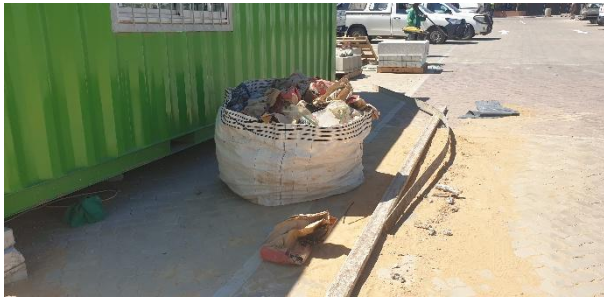
Empty cement bags collected for disposal.
