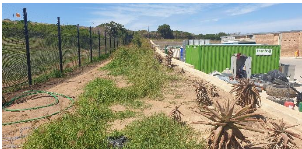
Rehabilitation Phase 1 in progress along the RE/219 boundary, on top of the retention wall.
