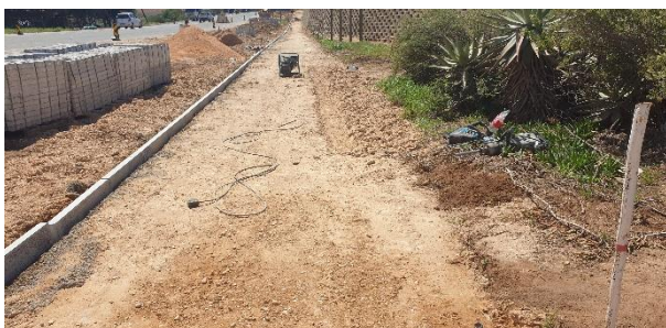
View of the constructed side path along the R102.
