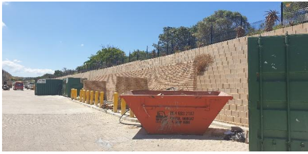
Eastern boundary (N2) retaining wall berm with transplanted indigenous trees.
