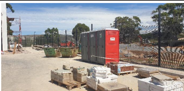
Chemical toilets available along the parking area of the construction area.
