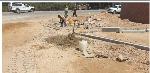
Construction of the entrance of the mall, paving, and cement works in progress.
