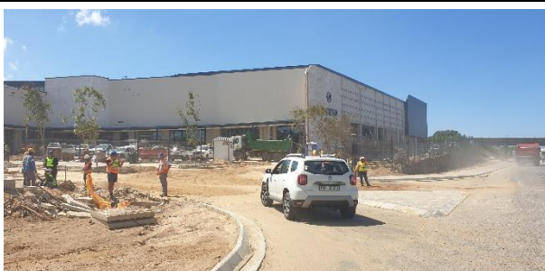
Entrance of the Garden Walk Mall along Monte Christo Rd.
