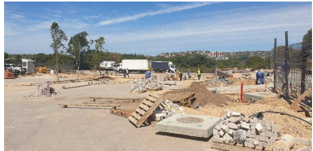
Construction of the entrance of the mall, paving, and cement works in progress.
