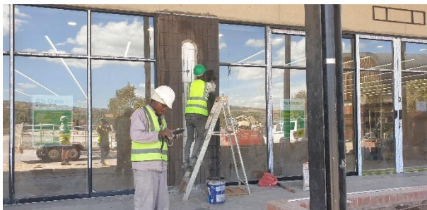
Paving and cement works in progress.
