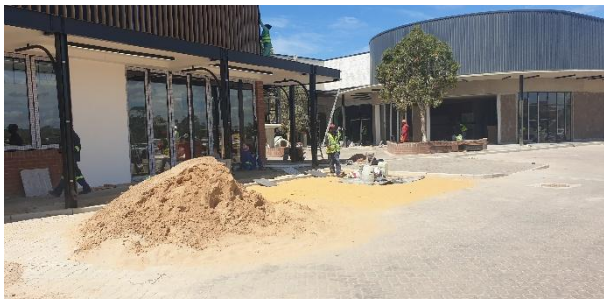
Building sand stockpile adjacent to ongoing paving and masonry activities.
