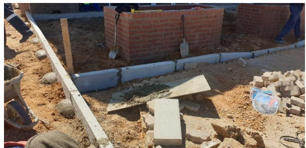
Installing paving blocks as part of a hard-surfaced area.
