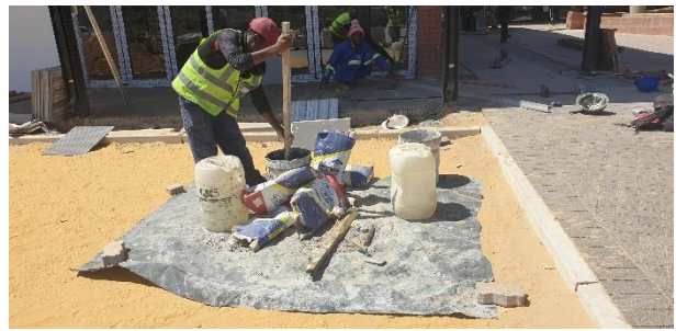
Preparing mortar on-site for ongoing paving or masonry activities.
