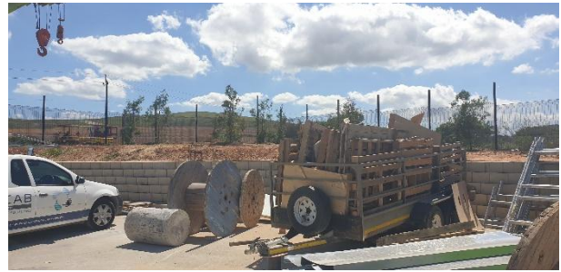
Storage and laydown area along the RE/219 boundary and retention wall being rehabilitated.
