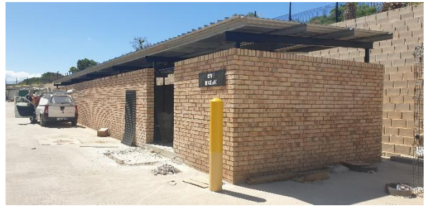
Delivery refuse yard.
