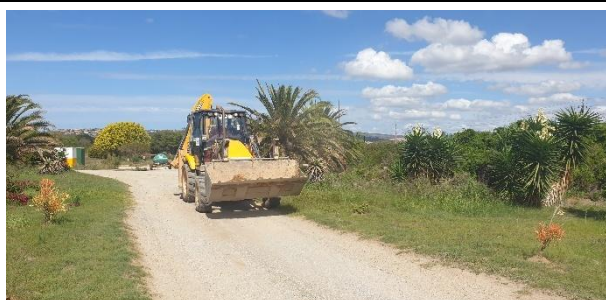
Construction machinery making use of existing hall roads.
