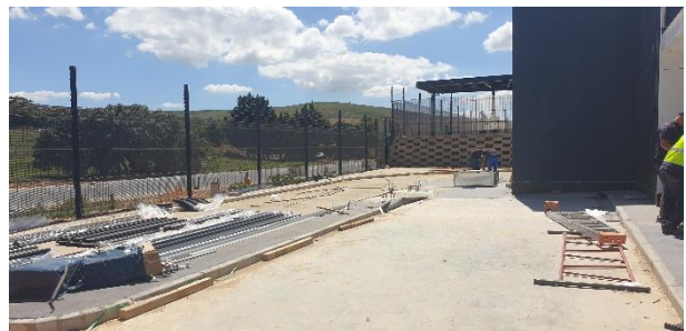
Laydown area adjacent to Burger King.
