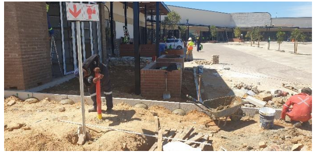
Installing paving blocks as part of a hard-surfaced area.
