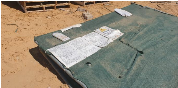
Green shade cloth screening that was installed around the perimeter of the mall building.
