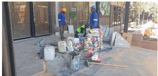
Paving and cement works in progress.
