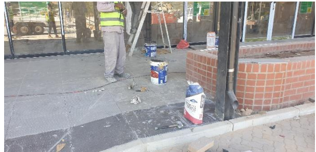
Paving and cement works in progress.
