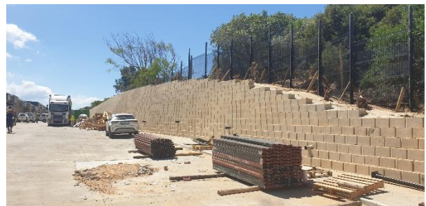
Eastern boundary (N2) retaining wall berm with transplanted indigenous trees.
