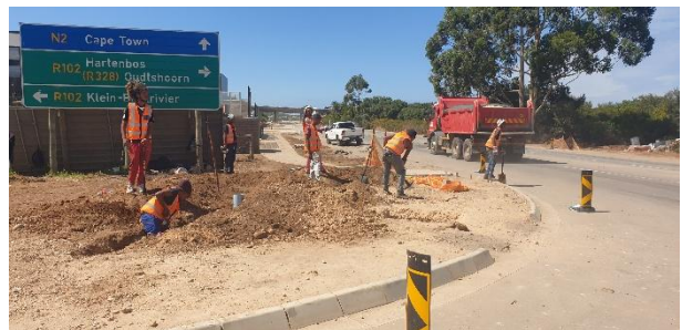
Stormwater services being installed along the entrance of the Garden Walk Mall along Monte Christo Rd.
