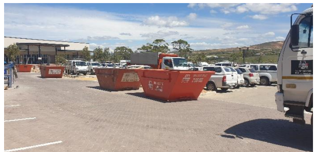
Skips available along the parking area of the Garden Walk Mall construction area.
