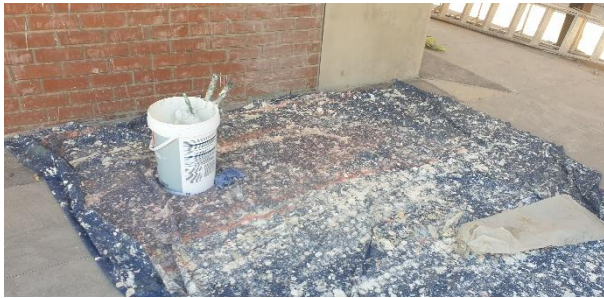
Painting works in progress on the exterior façade of the mall.
