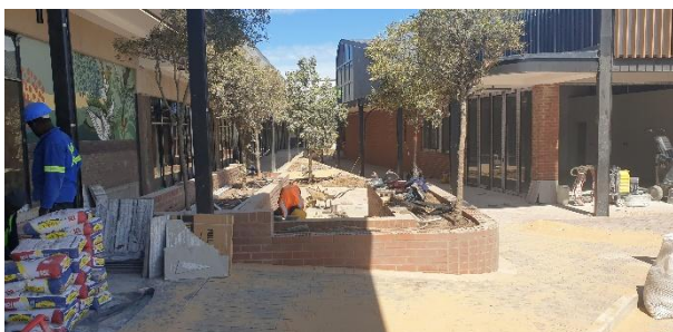
Paving and cement works in progress.
