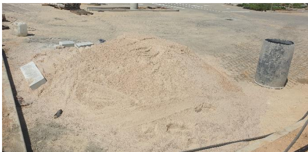
Building sand stockpile and bin in place near paving works within the parking area.
