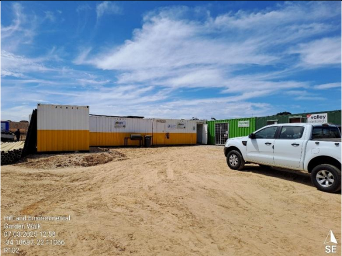
Earthworks contractor site camp
