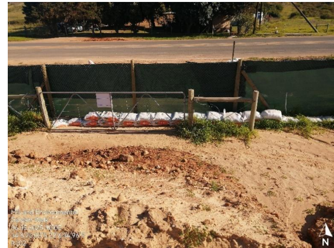
Additional sandbags were placed at the low point (old access point)
