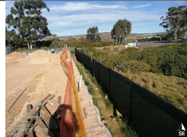
No stormwater runoff issues outside the demarcation noted.
