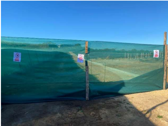
Photo of the rehabilitation area above the retaining wall – where work and access has been restricted.
