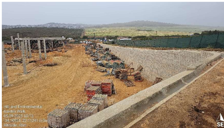
Photo of the area below the retaining wall where a S24G rectification application will be made to retain the area already cleared of vegetation.
