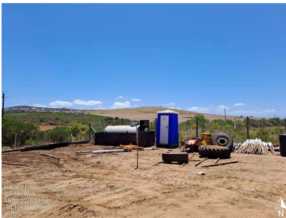
Site camp as it was being set up.
