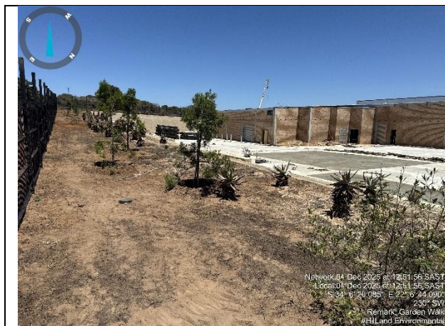
Showing phase 1 rehabilitation.
