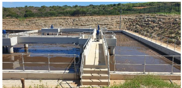
Newly constructed biological reactor.
