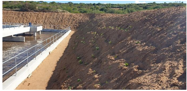
Slopes surrounding the biological reactor being rehabilitated.
