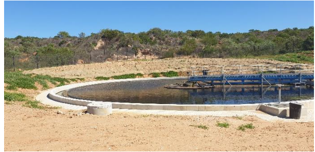
Newly constructed clarifier.
