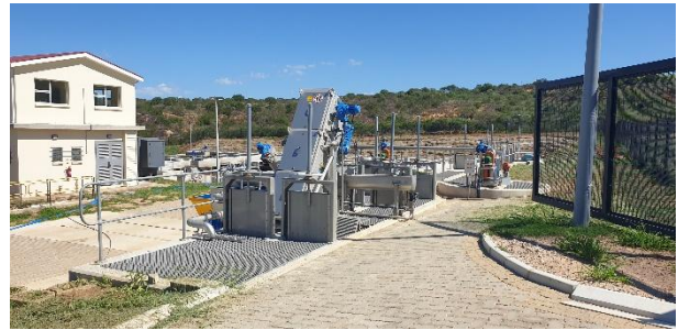
Newly completed inlet works.
