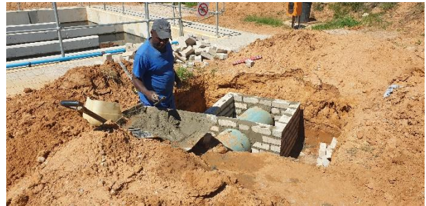
Finishing a brick valve chamber around pipeline valves
