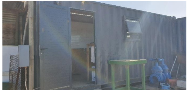
Condition of the site camp.
