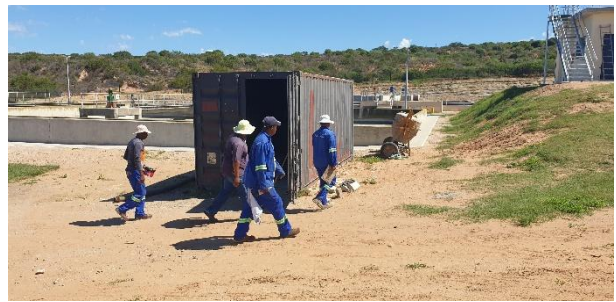
Single container still located on site.
