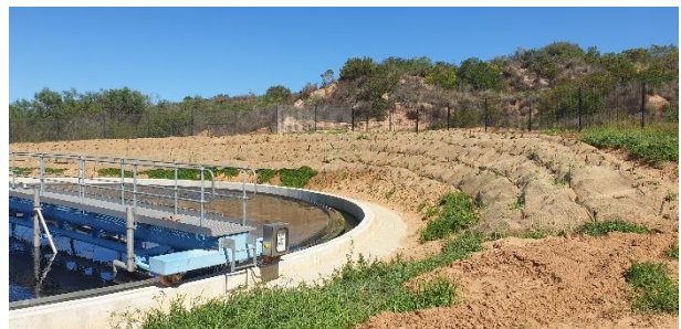
Rehabilitation of the slopes above the newly constructed clarifier.
