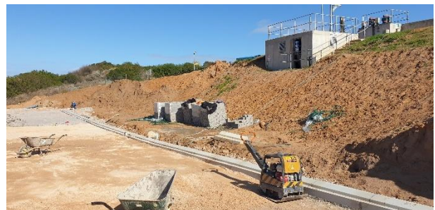
Grading and shaping of the slope adjacent to the Ras Pump Station.
