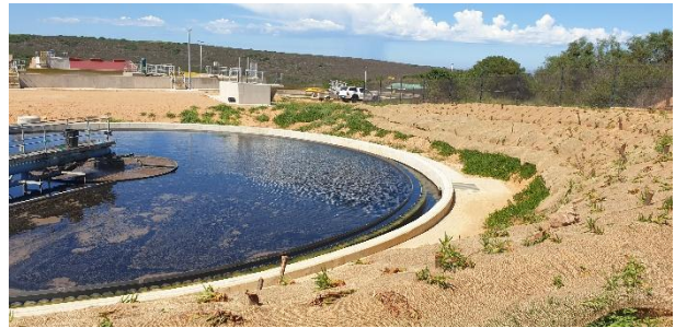
Newly constructed clarifier.
