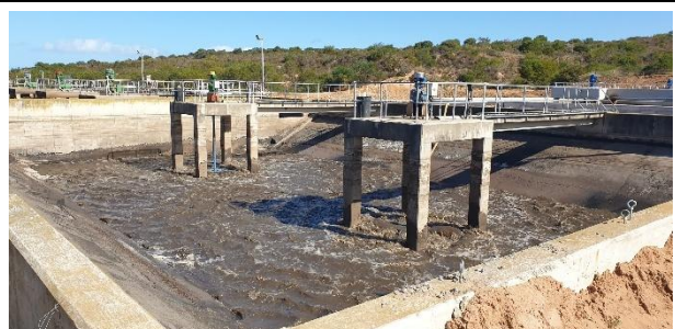
Existing biological reactor being pumped out.
