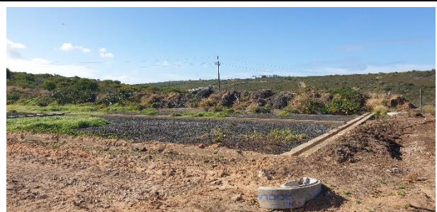
Topsoil stockpiles are placed at the back of the future emergency sludge drying beds
