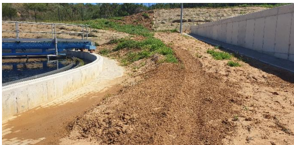
Stormwater/surface water diversion channel created surrounding the newly constructed clarifier.
