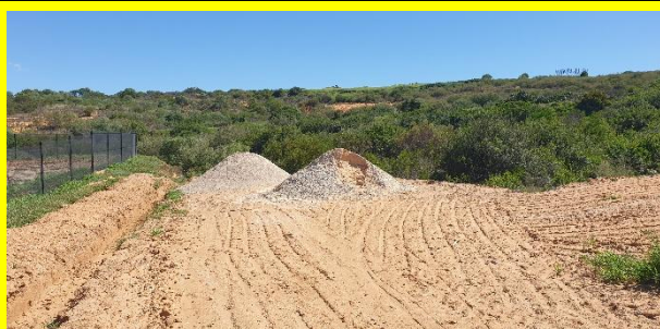
Stockpiles placed adjacent to the suggested parking area at the entrance of the WWTW to be removed.
