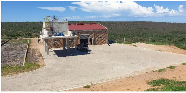
Newly constructed mechanical dewatering facility.
