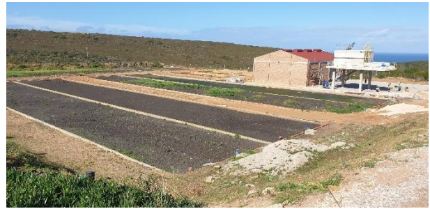
Location of the existing sludge drying beds and future emergency sludge drying beds.
