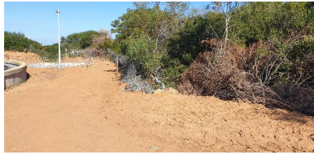
Existing fence to be reinstated.
