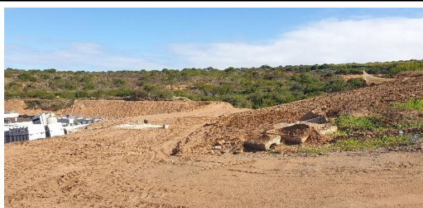
Parking area towards the existing and new inlet works and biological reactor.
