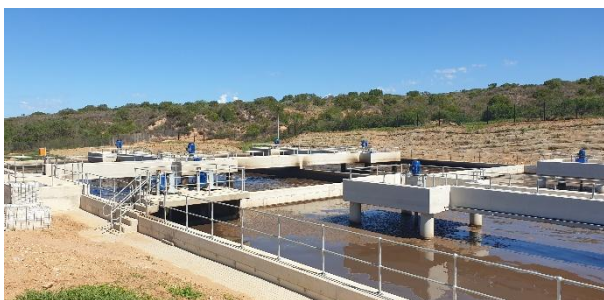
Newly constructed biological reactor.
