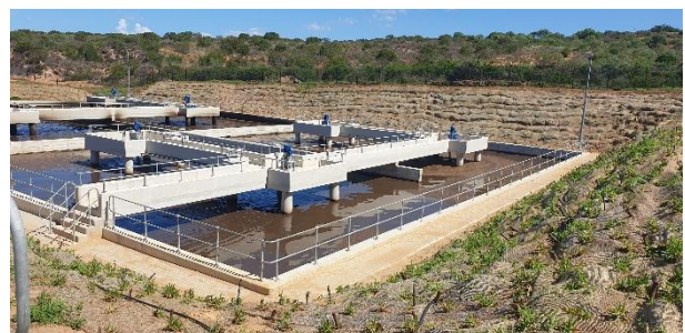
Rehabilitation of the slopes surrounding the newly completed biological reactor.
