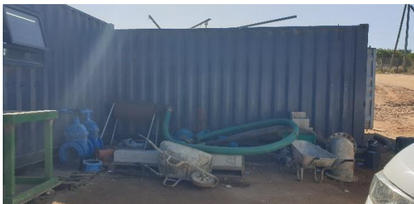
Laydown area adjacent to the site camp.
