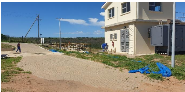
Paving works completed adjacent to the newly constructed inlet works.
