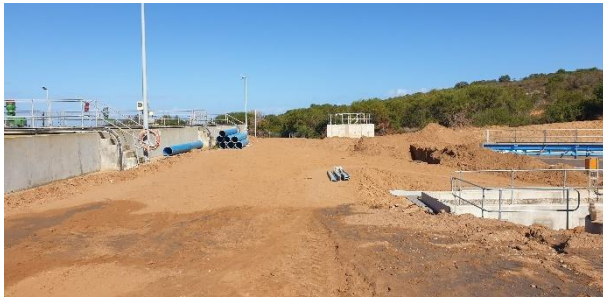
Walkway between the existing and new biological reactor.
