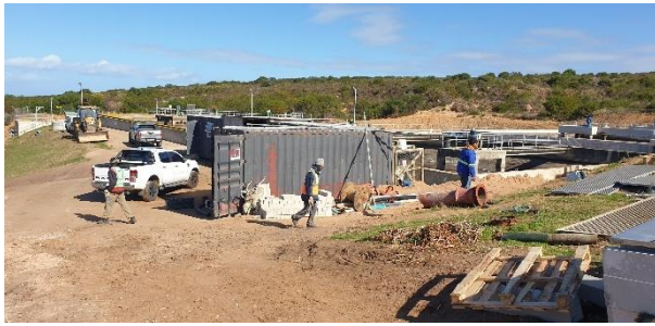
Location of the site camp adjacent to the new office building.
