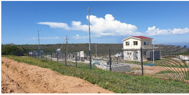
ClearVu Fence installed surrounding the WWTW plant.
