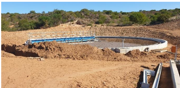
Newly constructed clarifier.
