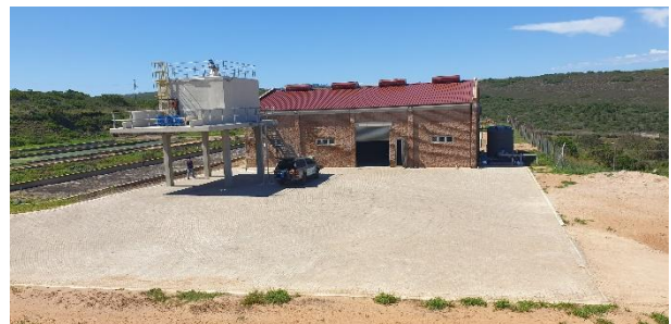
Newly constructed mechanical dewatering facility.
