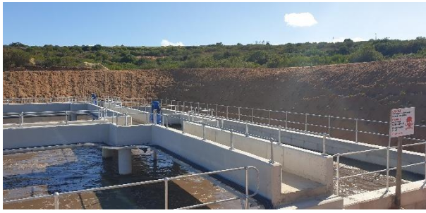
Newly constructed biological reactor.
