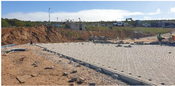
Paving of the ring road along the new mechanical dewatering facility.
