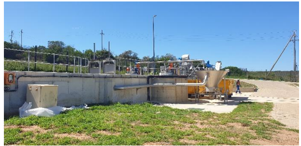
Newly completed inlet works.
