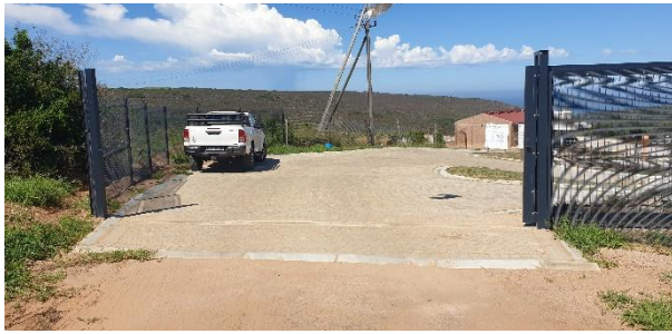
Newly paved access road to the WWTW.
