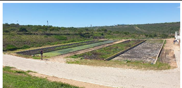
Existing sludge drying beds.
