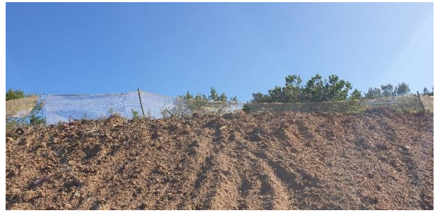
Orange netting is in place along the natural boundary of the new biological reactor and clarifier.
