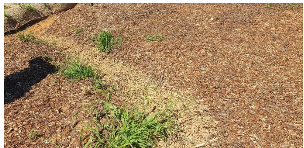
Small stormwater diversion channel created above the newly constructed clarifier.
