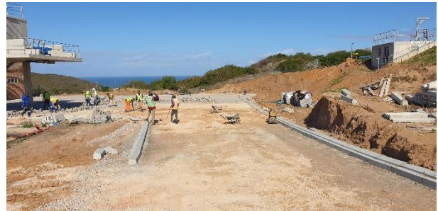
Layering of the ring road, curbs being installed.
