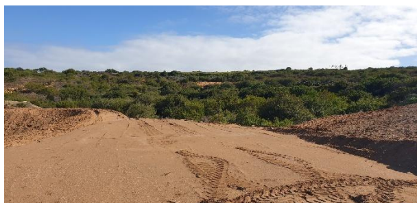
Parking area towards the natural area, and the embankment of the new biological reactor.
