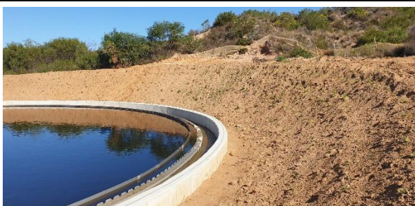
Shaping and grading of the slopes surrounding the clarifier to be rehabilitated.
