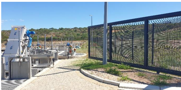
Newly completed inlet works.
