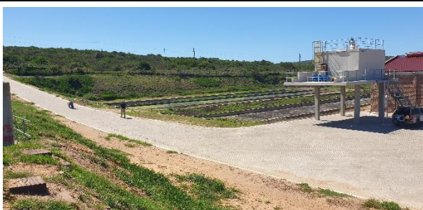
Paving completed of the ring road towards the mechanical dewatering facility.
