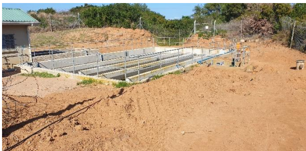
Existing chlorine channel and building on site.
