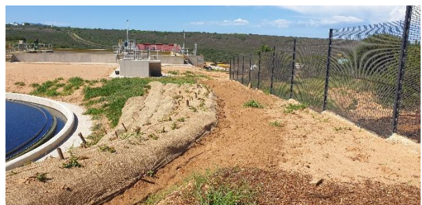
Stormwater/surface water channel surrounding the clarifier.
