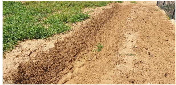
Stormwater/surface water channel surrounding the clarifier.
