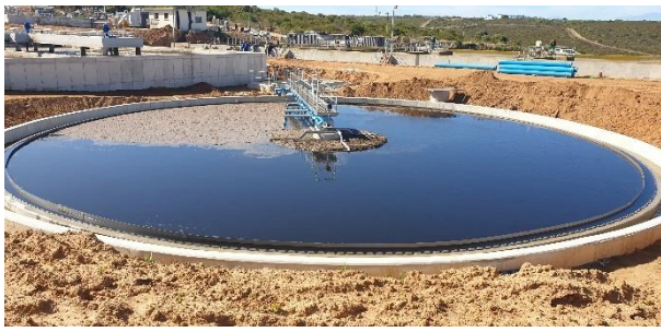
Newly constructed clarifier.
