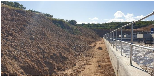
Shaping and grading of the slopes adjacent to the new biological reactor.
