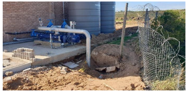
Exiting fence to be reinstated, adjacent to the new mechanical dewatering facility.
