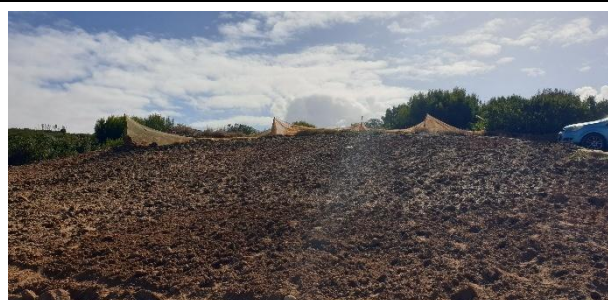
Parking area at the entrance of the WWTW. Stockpiles have been placed there and are busy being shaped.
