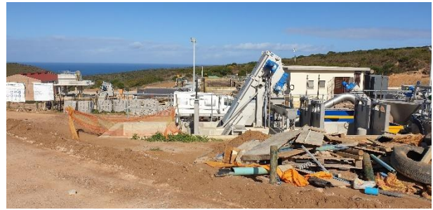
Construction of the new inlet works.
