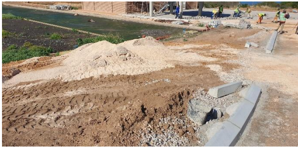
Layering of ring road, curbs being installed.
