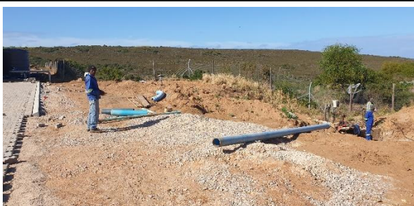
Construction of the new super native pump station.
