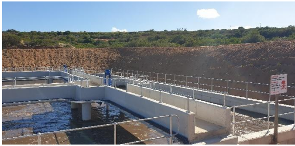
Newly constructed biological reactor.
