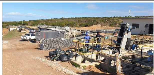
Construction of the new inlet works.
