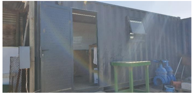
Condition of the site camp.
