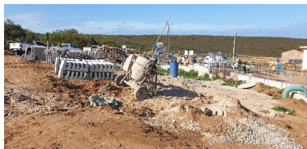
Laydown area located next to the new inlet works.
