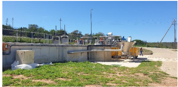
Newly completed inlet works.
