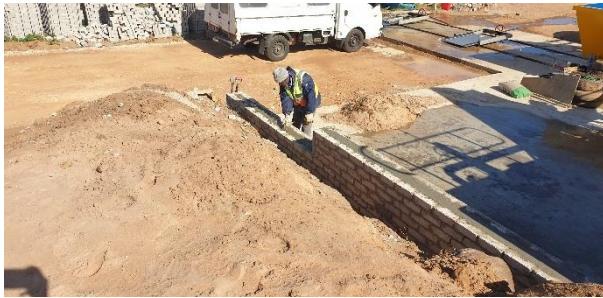
Construction of the new inlet works (cement batching active).
