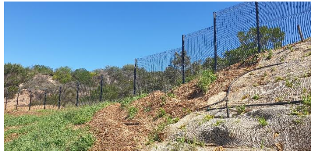
Rehabilitation of the slopes above the newly constructed biological reactor and clarifier.
