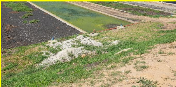
Building material to be removed adjacent to the existing sludge drying beds.
