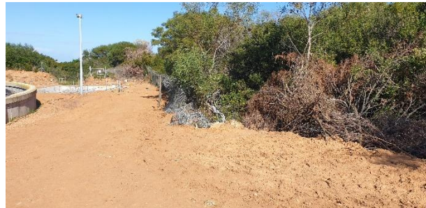
Existing fence to be reinstated.
