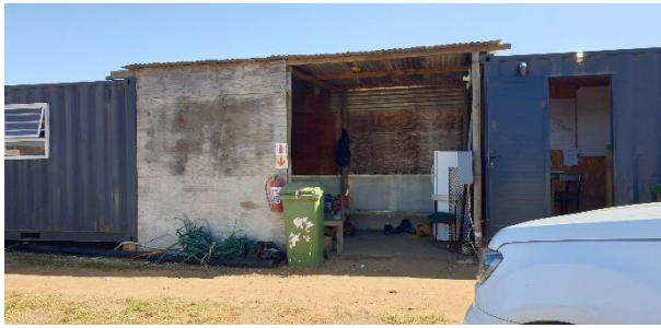
Site camp with waste bin and fire equipment in place.
