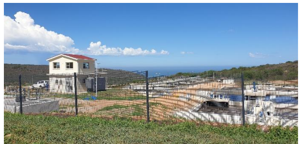
ClearVu Fence installed surrounding the WWTW plant.
