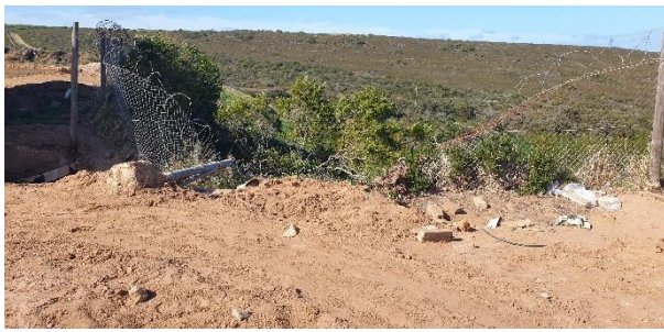
Exiting fence to be reinstated.
