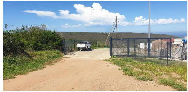
Newly paved access road to the WWTW.
