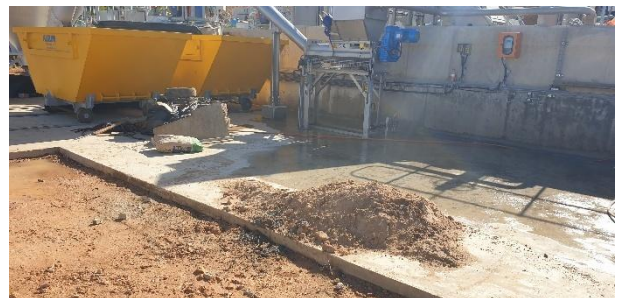
Construction of the new inlet works (cement batching active).
