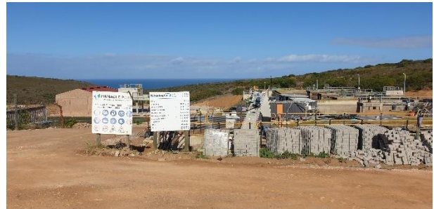
Laydown area and notice boards adjacent to the new inlet works.
