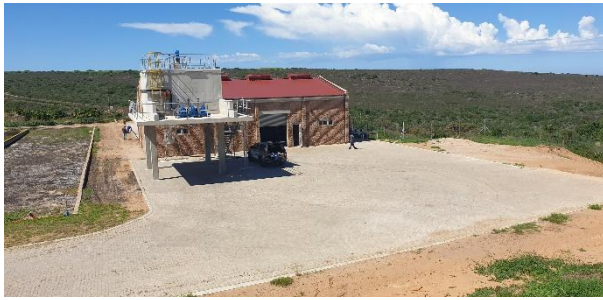
Newly constructed mechanical dewatering facility.
