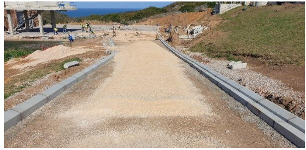
Layering of the ring road, curbing being installed.
