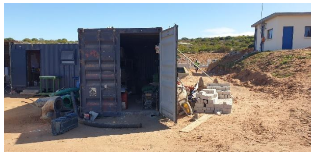
Lockable storage container adjacent to the site camp.
