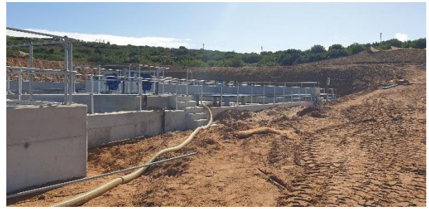
Existing matter within the existing biological reactor being pumped into the new biological reactor.
