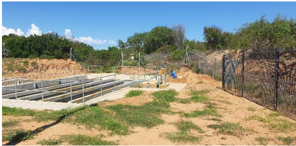
Existing chlorine channel and building on site.
