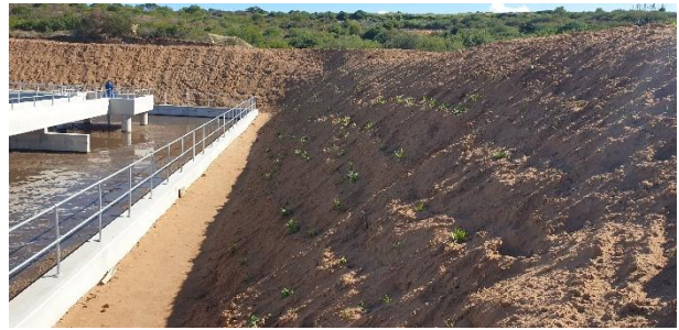
Slopes surrounding the biological reactor being rehabilitated.
