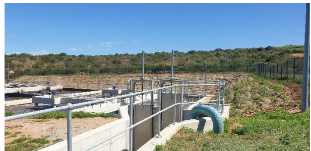
Newly completed inlet works.
