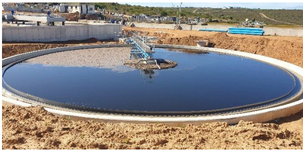
Newly constructed clarifier.
