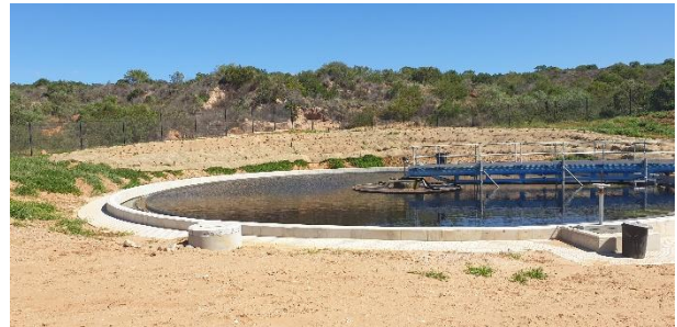
Newly constructed clarifier.
