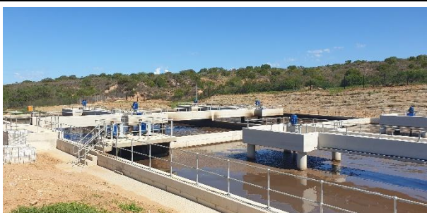
Newly constructed biological reactor.
