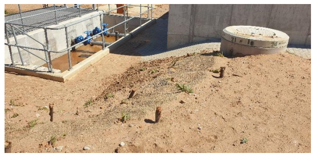
Rehabilitation surrounding the new Ras Pump Station between the new biological reactor and the new clarifier.
