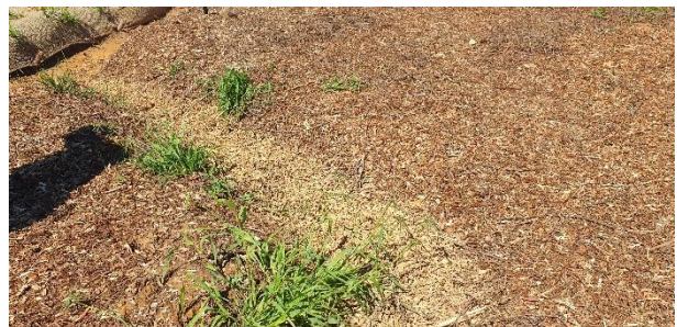
Small stormwater diversion channel created above the newly constructed clarifier.
