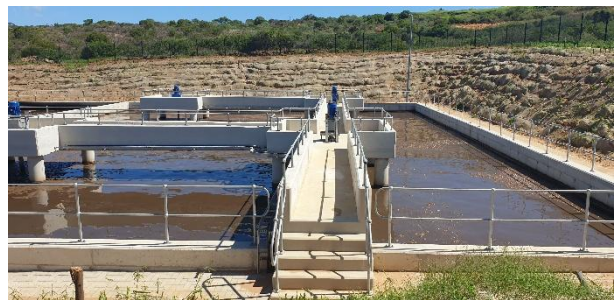
Newly constructed biological reactor.
