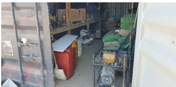
Fuel container and generator in place within the lockable storage container.
