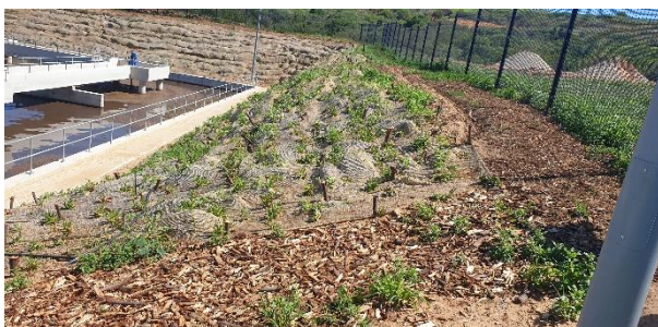
Rehabilitation of the slopes adjacent to the newly completed biological reactor.
