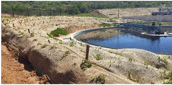
Rehabilitation of the slopes above the newly constructed clarifier.
