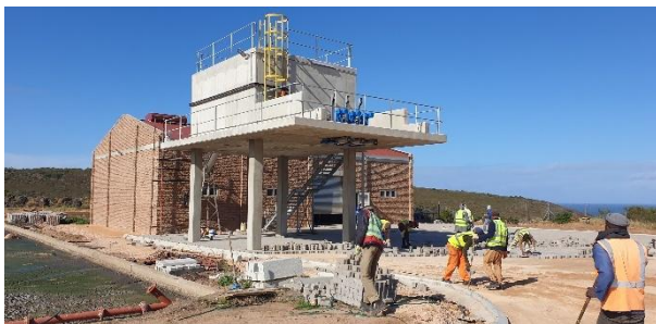
Construction of the new mechanical dewatering facility.
