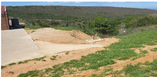
Completed construction of the new super native pump station.
