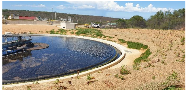
Newly constructed clarifier.
