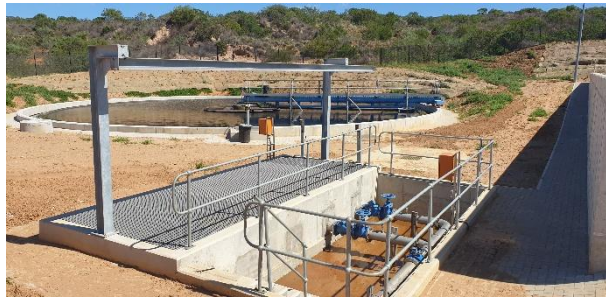
Newly constructed Ras Pump Station between the new biological reactor and the new clarifier.
