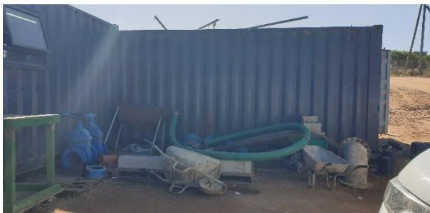
Laydown area adjacent to the site camp.
