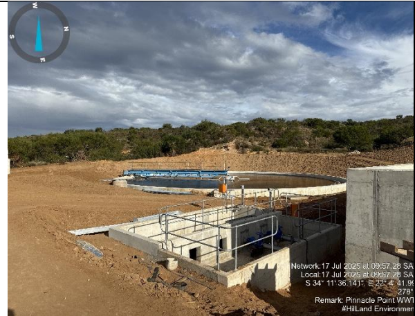
Pumpstation concrete work complete
