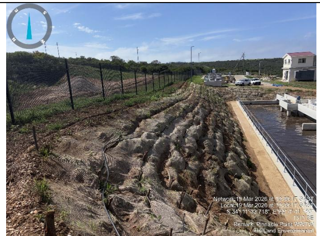
Slope rehabilitation / revegetation and erosion protection
