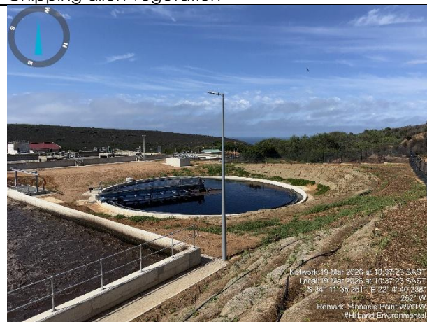
Construction completed - clarifier
