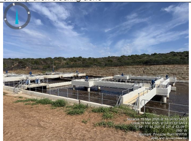
Construction completed – bio-reactor
