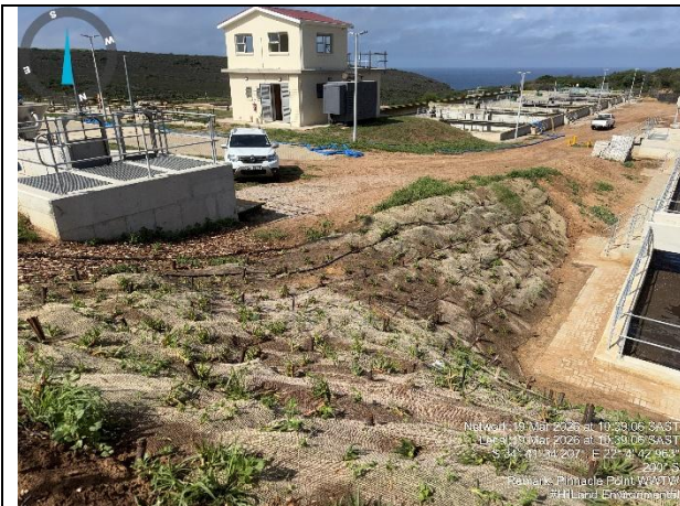
Slope rehabilitation / revegetation and erosion protection
