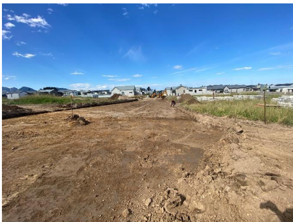
Construction of the main access road adjacent to the Phase 4 frail care development area in progress.
