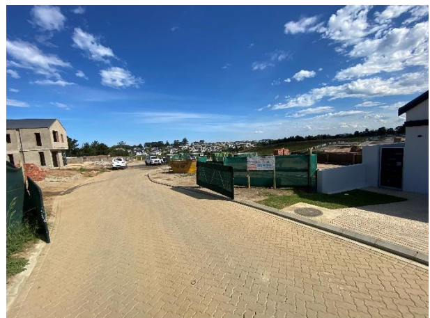
Construction of residence within Phase 3 fully demarcated.
