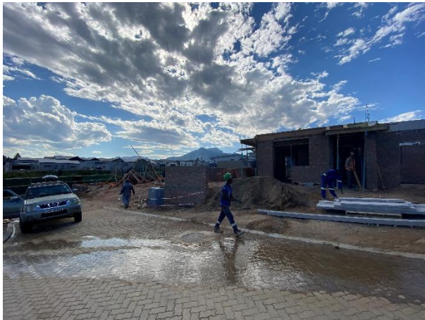
Construction of residences within Phase 3.
