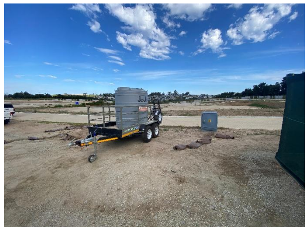
Jojo tank available at the Phase 4 development area for dust suppression.
