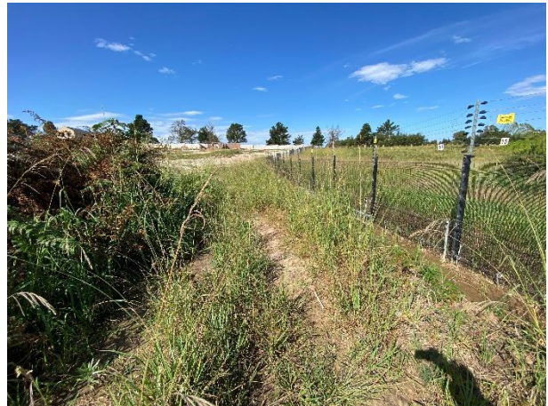
Wetland area fenced off with ClearVu fencing as seen towards the southeast where the road is proposed.
