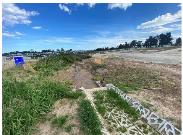
The sewer line and stormwater dissipator towards the south of Phase 4.
