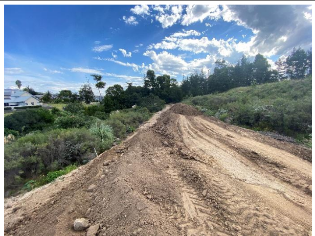
Swale created with rescued topsoil within Phase 5. Swale placement remains within the staked area.
