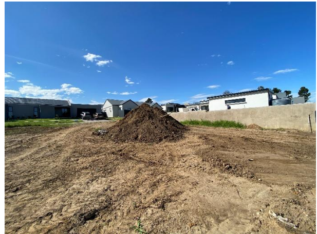
Topsoil stockpile placed within an open erven of Phase 3 as seen towards the north.
