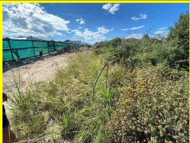
Buffer area along the wetland staked. Spoiled material must be removed.
