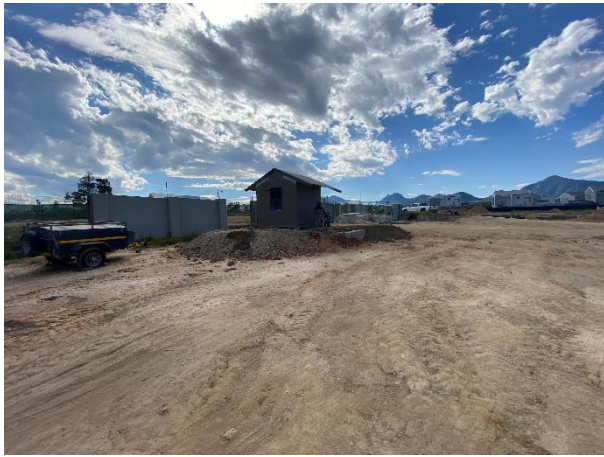
Site office of the frail care development area within Phase 4.
