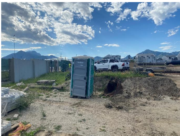
Chemical toilet in place adjacent to the frail care facility development area and main access road being constructed.
