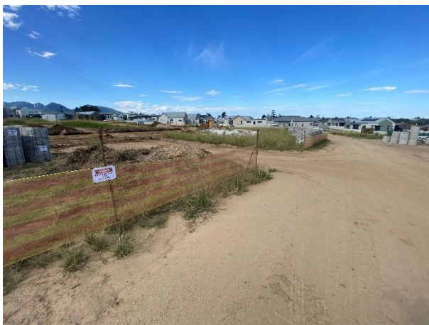
Condition of the frail care development area within Phase 4, pegged and demarcated.
