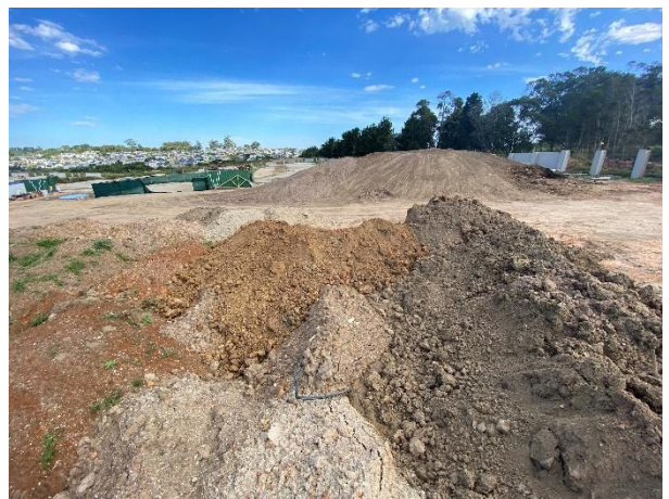
Topsoil and subsoil stockpile area within the Phase 4A and 4B development area. Stockpiles separated.
