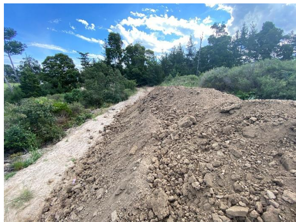
Swale created with rescued topsoil within Phase 5.
