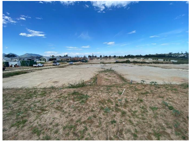
Phase 4A and 4B development area cleared for civil services installation and construction of top structures.
