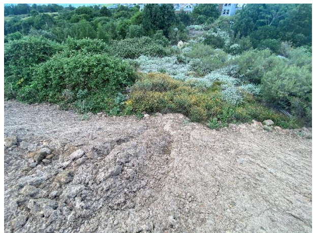
Swale created with rescued topsoil within Phase 5.
