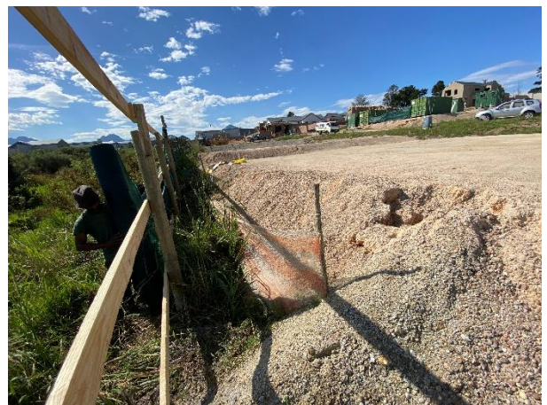
Construction fencing along the wetland buffer being installed.
