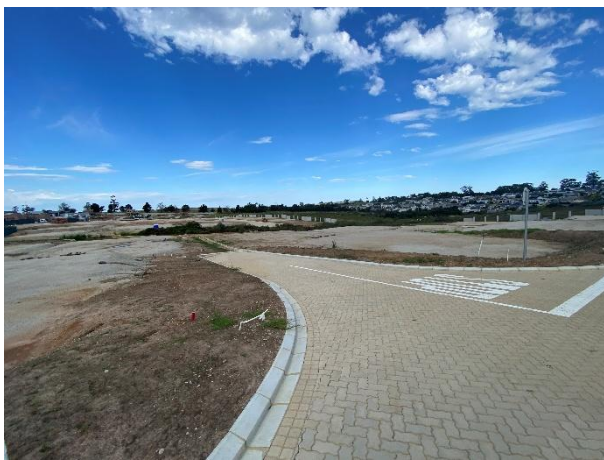
Phase 4A and 4B development area cleared for civil services installation and construction of top structures.
