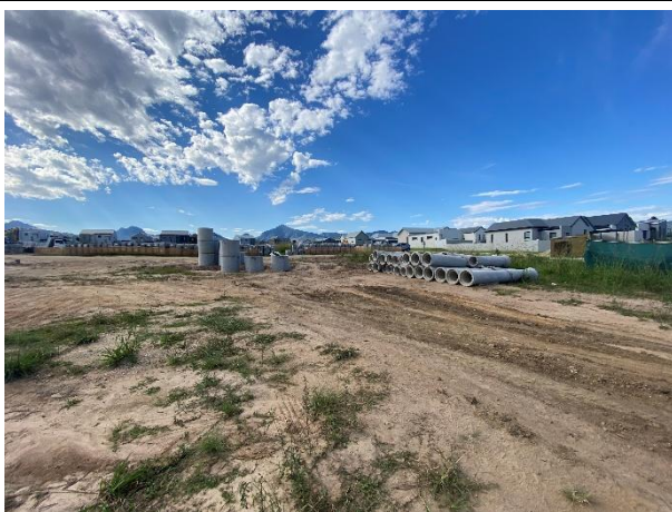
Material placed within the development footprint for civil services installation within the frail care and assisted living facility (associated with Phase 4).
