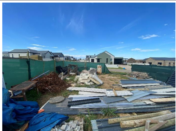
Temporary material laydown area and site camp on an existing erf within Phase 4 (frail care facility).
