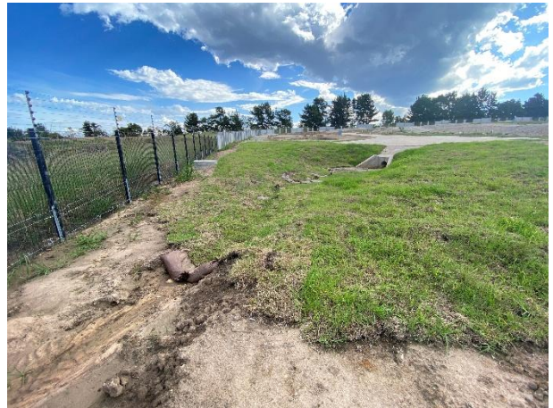
The sewer line and stormwater dissipator installed and rehabilitation of phase 4B is in process.
