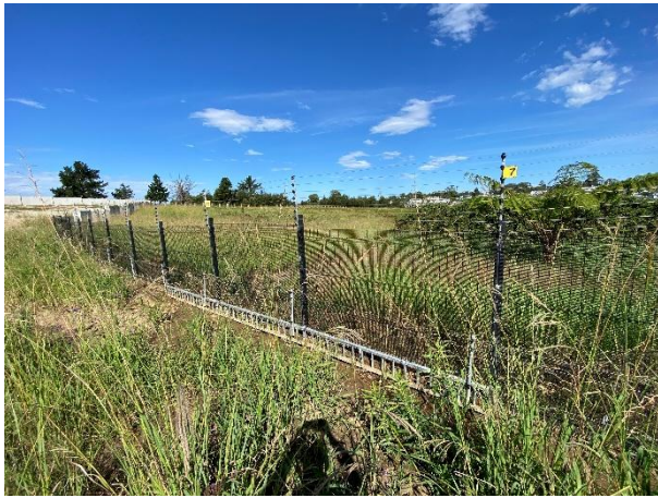
Wetland area fenced off with ClearVu fencing. Steel grid towards the southeast.
