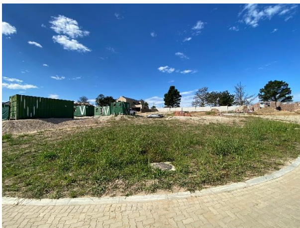
Construction site camp and available storage containers on an existing erf within Phase 4 of the frail care facility
