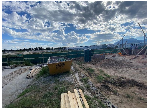
Construction of residences within Phase 3, with a skip and chemical toilet in place.
