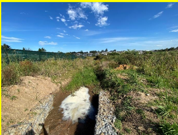
Paint were washed by contractors, resulting in paint residue entering the constructed stormwater outlet within the Phase 4B buffer area.
