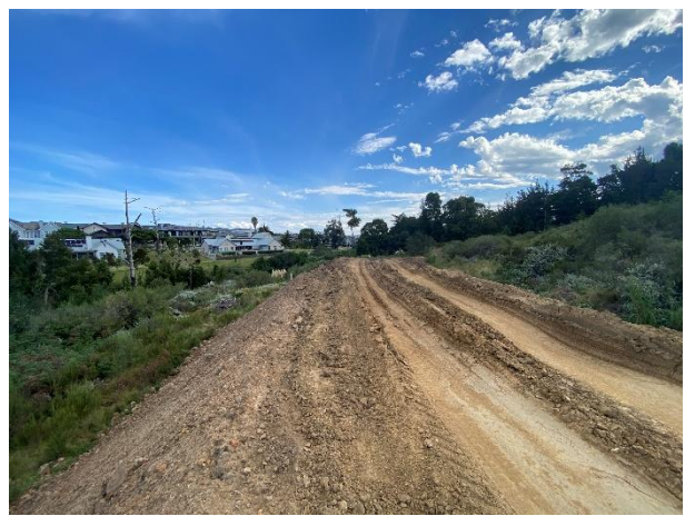
Swale created with rescued topsoil within Phase 5.
