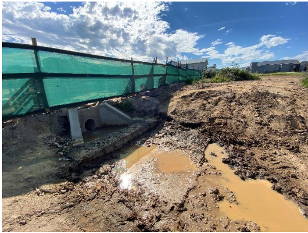
Constructed stormwater outlets within the buffer area of Phase 4B with energy dissipators (reno-matgrass).
