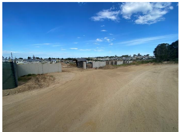
Current main access road being constructed.
