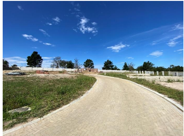
Condition of the frail care development area within phase 4 civil services installations and earthworks in progress
