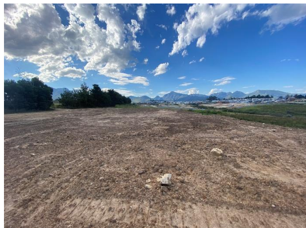
Dumped soil has been levelled at the northernmost section of the Phase 5 future development, as seen towards the north.
