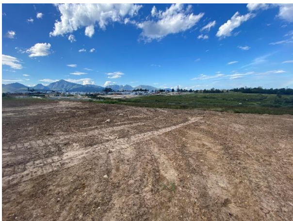
Dumped soil has been levelled at the northernmost section of the Phase 5 future development, as seen towards the northeast.
