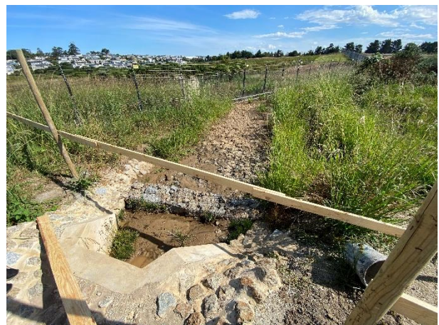
Constructed stormwater outlets within the buffer area of Phase 4B with energy dissipators (reno-matgrass) as seen towards the northeast.
