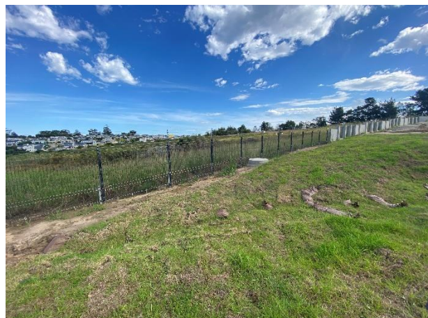
Wetland area fenced off with ClearVu fencing.
