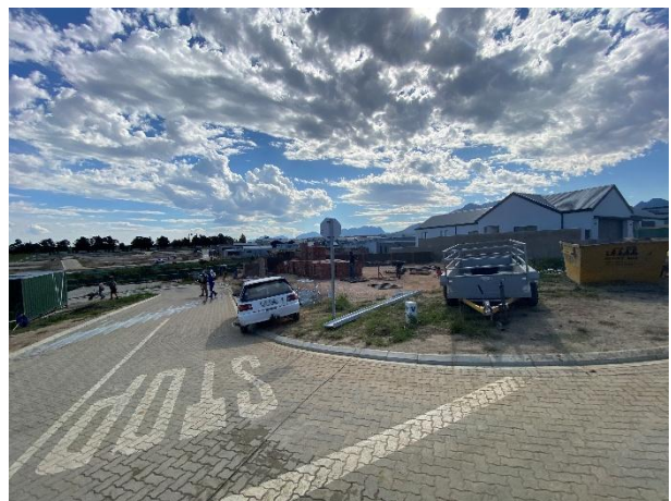
Construction of residences within Phase 3, with a skip available for waste disposal.
