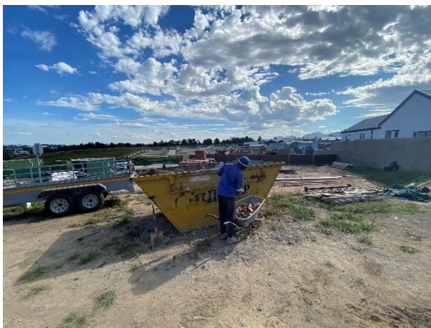
Construction of residences within Phase 3, with a skip available for waste disposal.
