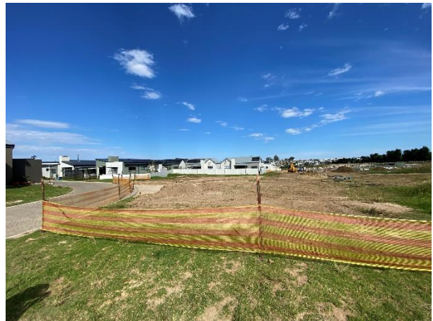
View towards the southeast looking onto the Phase 4 assisted living development area. Construction netting in place.
