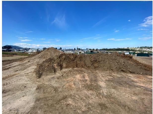
Condition of the frail care development area within phase 4, site clearance in progress.
