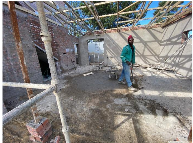
Construction of residences within Phase 3, cement batching on existing foundations.
