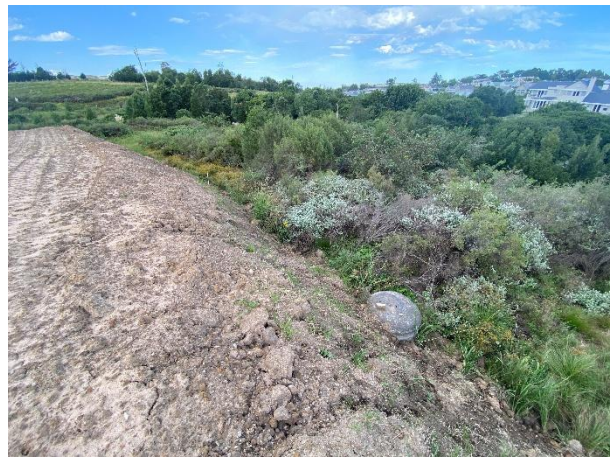
Swale created with rescued topsoil within Phase 5. Sewer manholes installed along the swale.
