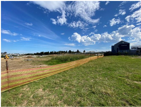
View towards the southwest looking onto the Phase 4 assisted living development area. Construction netting in place.
