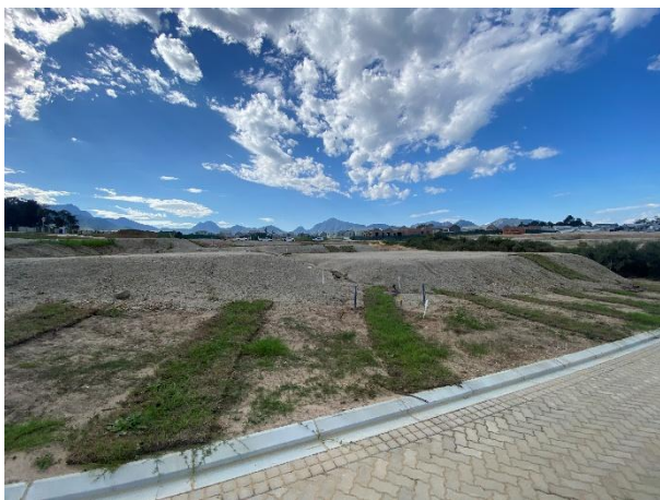
Kikuyu grass being planted towards the southeast of the wetland. Care must be taken to ensure encroachment is managed.
