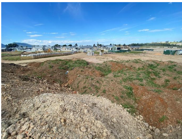
Topsoil and subsoil stockpile area within the Phase 4A and 4B development area. Stockpiles separated.
