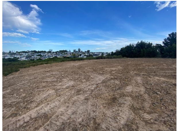
Dumped soil has been levelled at the northernmost section of the Phase 5 future development, as seen towards the southeast.
