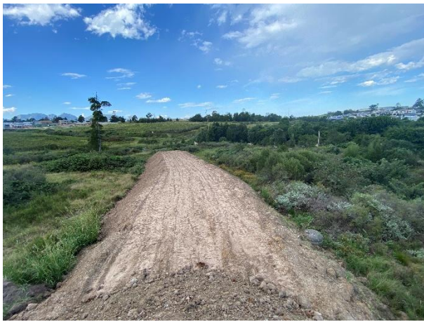
Swale created with rescued topsoil within Phase 5.
