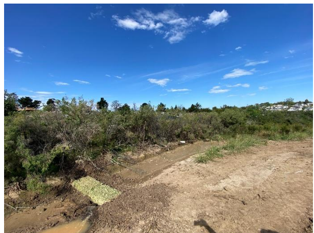
Additional silt protection (hay-bales) installed at the stormwater outlet area to prevent contaminated soil/silt from entering the wetland.
