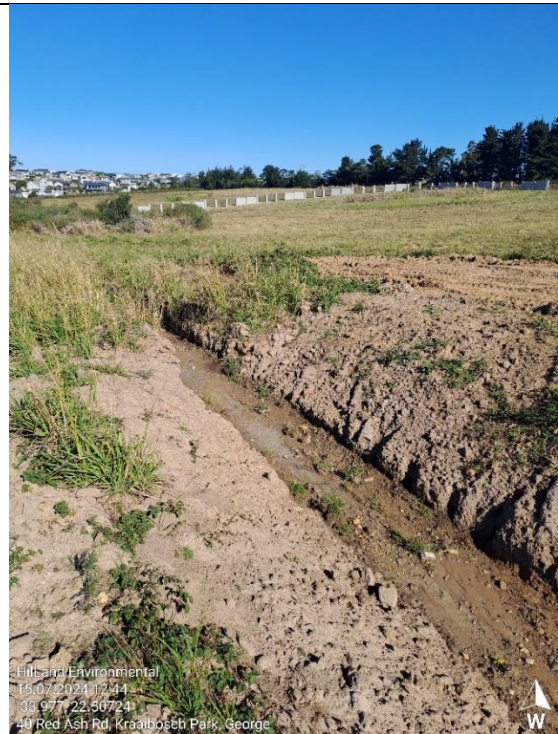
The sides of the stormwater outlets must be monitored for erosion while they are still revegetating.
