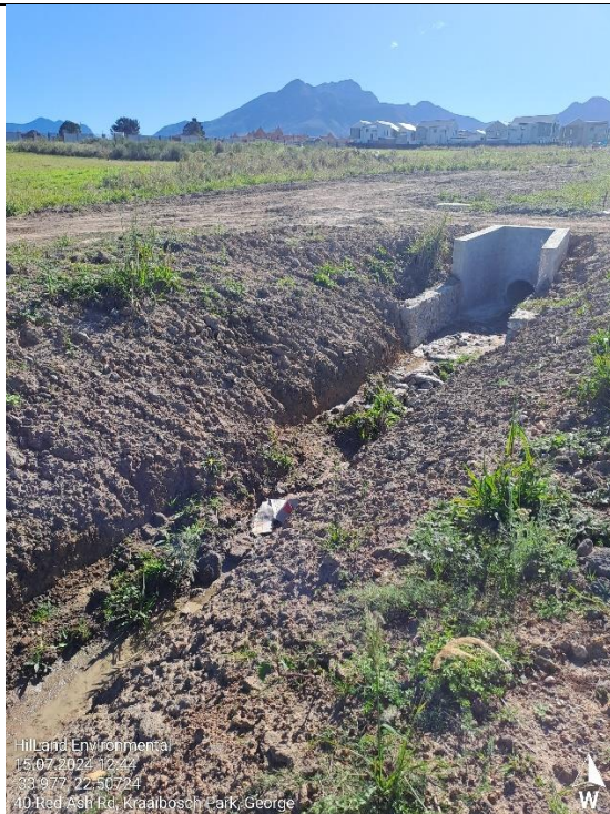
Sandbags must be continuously maintained in the stormwater outlet to reduce erosion.
