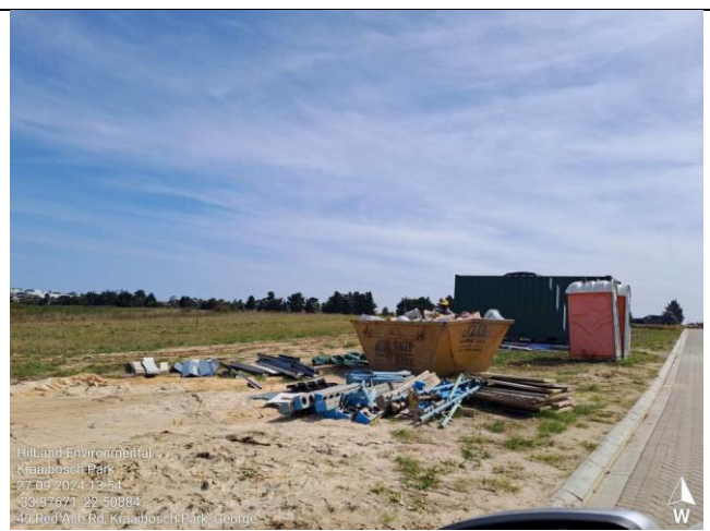
Contractors site camp – future development erf. Skips and toilets throughout construction site
