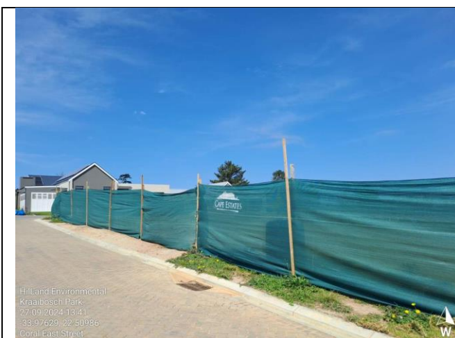
Demarcation of the construction sites.
