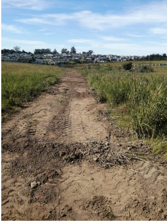
The sewer line – topsoil replaced, and small soil berms added for extra erosion protection.
