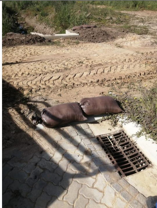
Sandbags have been placed in erosion prone areas and to divert water to the stormwater inlets.
