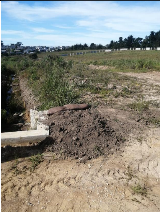
Erosion spots have been repaired and additional sandbags placed
