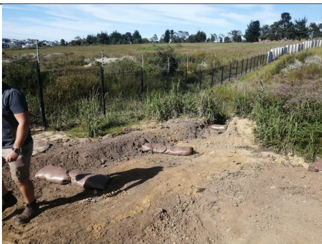
Eroded areas have been covered with topsoil and rows of sandbags/small soil berms have been installed.
