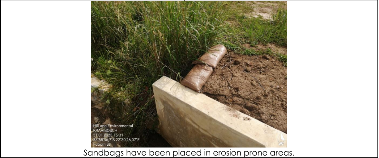
Eroded areas have been covered with topsoil and rows of sandbags/small soil berms have been installed.
