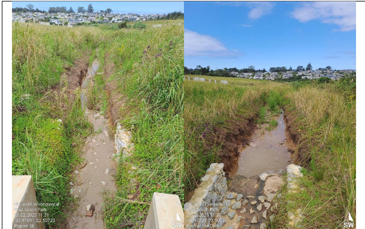
Sandbags within stormwater channels to be maintained
