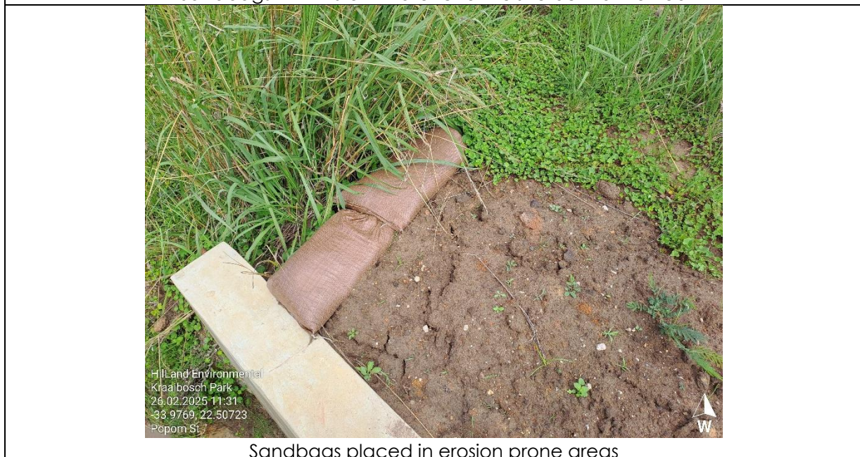
Sandbags within stormwater channels to be maintained
