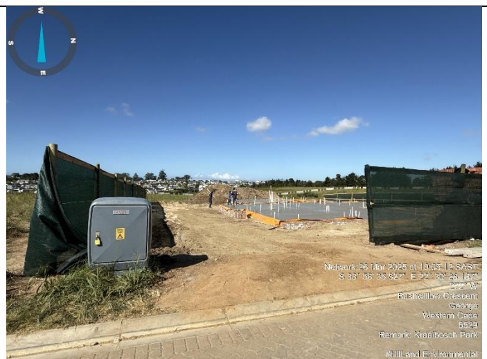
Construction in progress. Site is demarcated with green shade netting.
