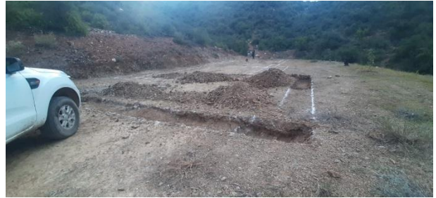
Platform/site layout demarcated with chalk.
