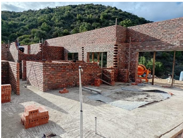
Brickwork progressing steadily.
