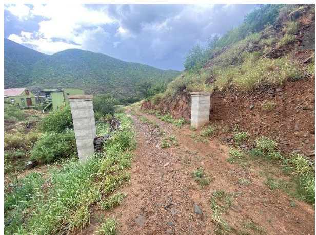
Condition of the access road at the entrance of the site.
