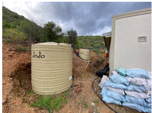
Jojo tank along the southern boundary of the main house.
