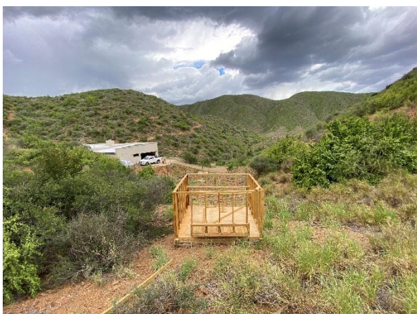
Chicken coop deck on stilts towards the northeast.
