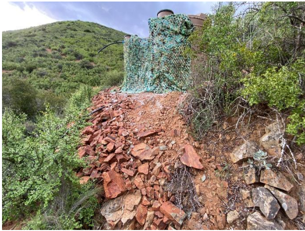
Condition of the water tank towards the northwest.
