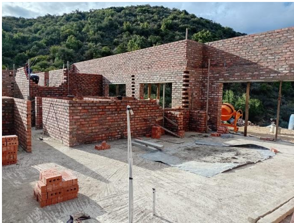
Brickwork progressing steadily.
