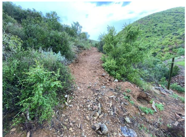
Condition of the footpaths towards the water tank.
