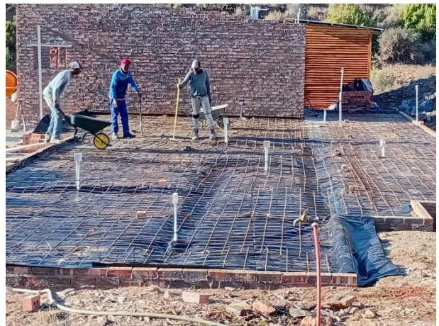
Prepared foundation with brick formwork and steel reinforcement grid.
