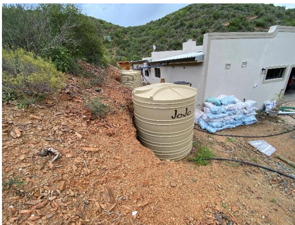
Jojo tank along the southwestern boundary of the main house.
