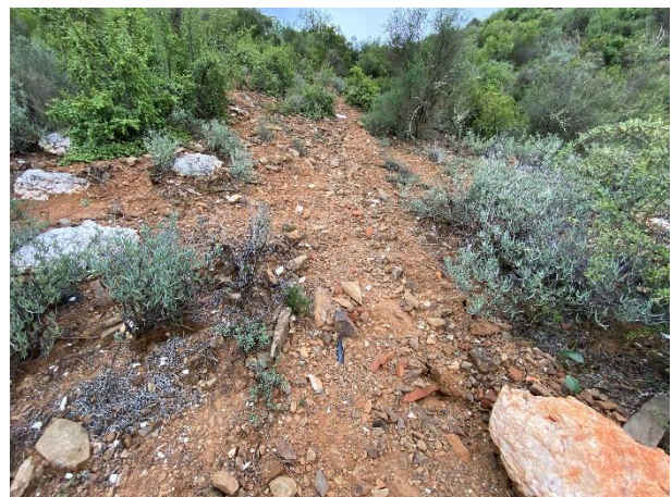
Condition of the footpaths towards and surrounding the water tank.
