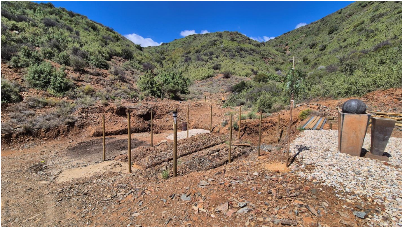
Image 7 – 8 indicating additional works adjacent to the house platform. Potential additional substrate / land clearing removed for construction
