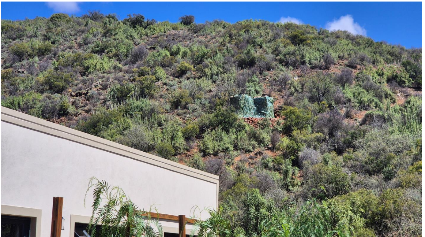
Image 10 water storage tank and platform
