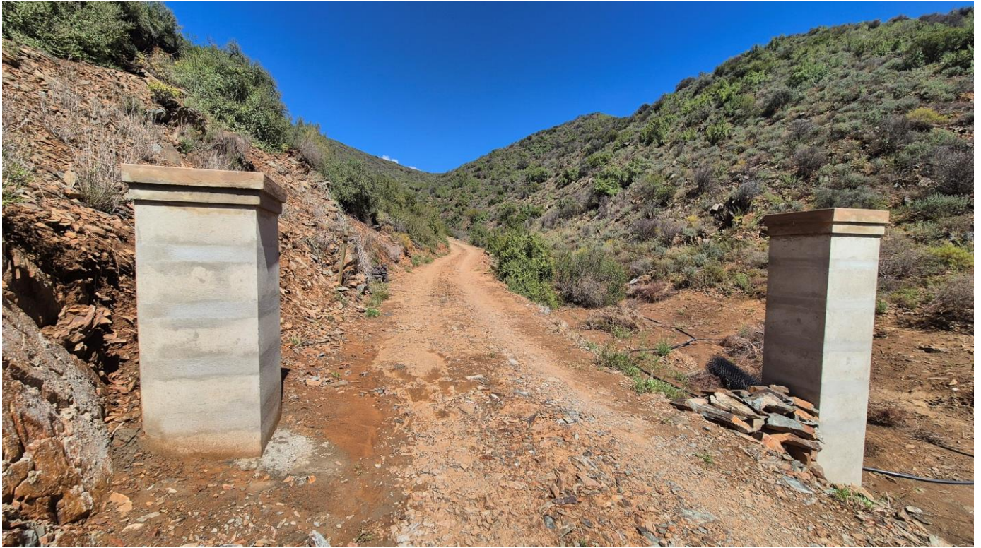
Image 1 – entrance to the site with approved road to dwelling
