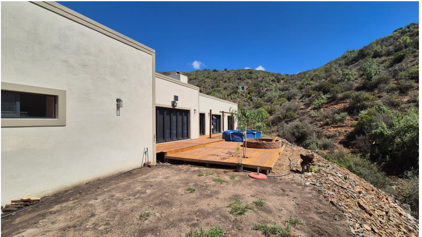
Image 3 – 6 showing the platform with constructed dwelling
