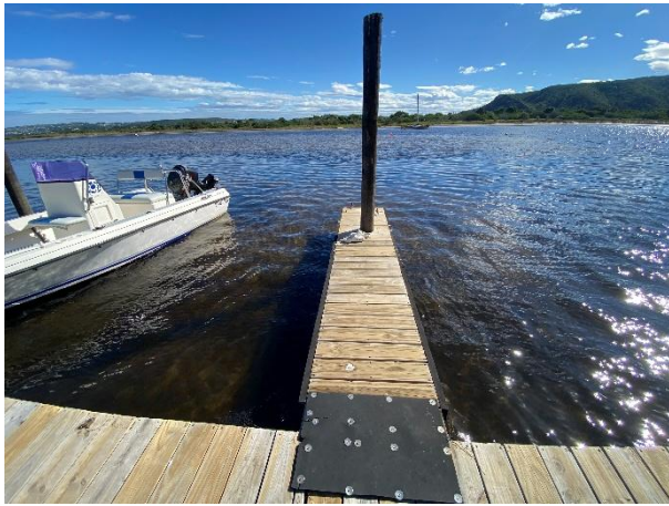
Attached floating jetty and the 4-meter-long by 0.7-meter-wide mooring finger.
