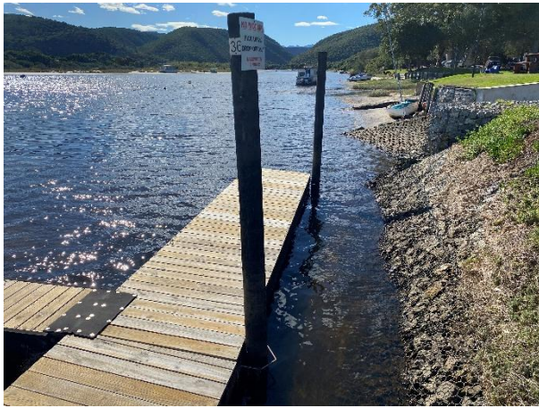
The northern end of the jetty showing the completed layers of the reno-matresses and established bank.
