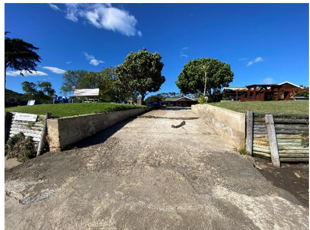
Condition of the slipway.
