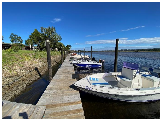
Completed and operational jetty as seen towards the south.
