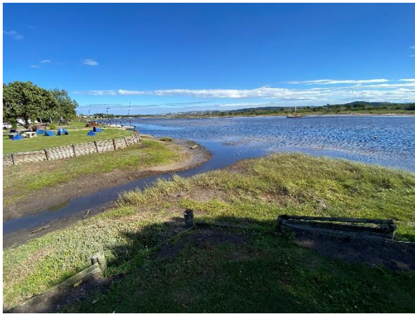
Stormwater outlet channel north of the slipway.
