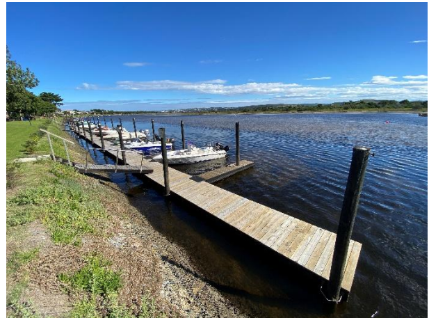
The banks and jetty as seen from the north.
