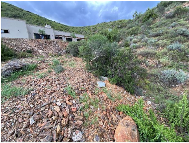
Property boundary at 33°29.6425' S; 21°36.9680' E.
