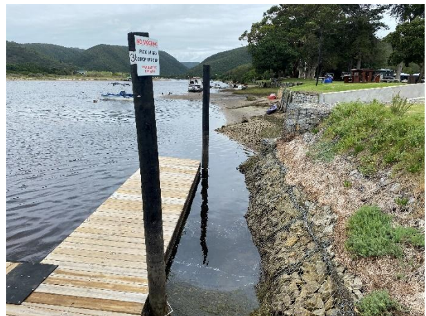
The mooring poles nearest to the slipway as seen towards the north.
