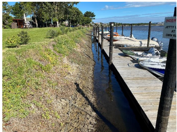
Rehabilitation of the riverbank.
