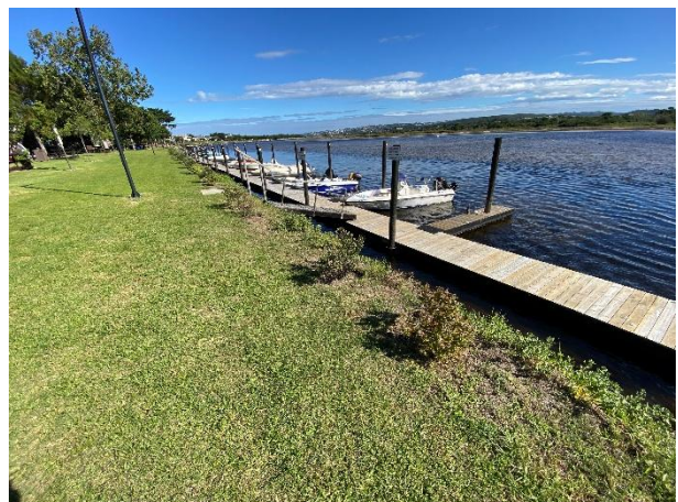
Current condition of the rehabilitation riverbank.
