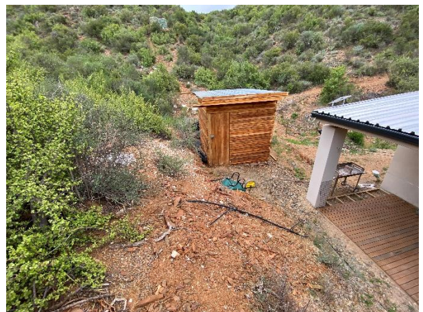
Condition surrounding the outhouse adjacent to the main house.
