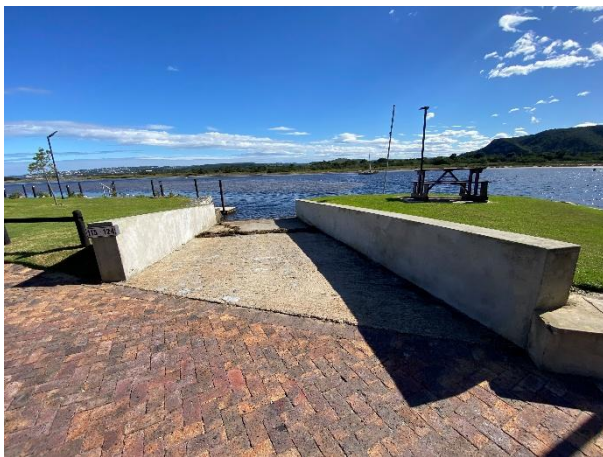
Condition of the slipway from the roadside.
