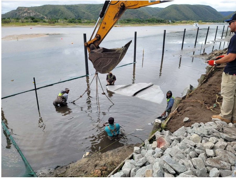
Geofabric being installed. Photograph showing curtain silt fencing in place around the working area and machine standing on the bank with guidance from below.
