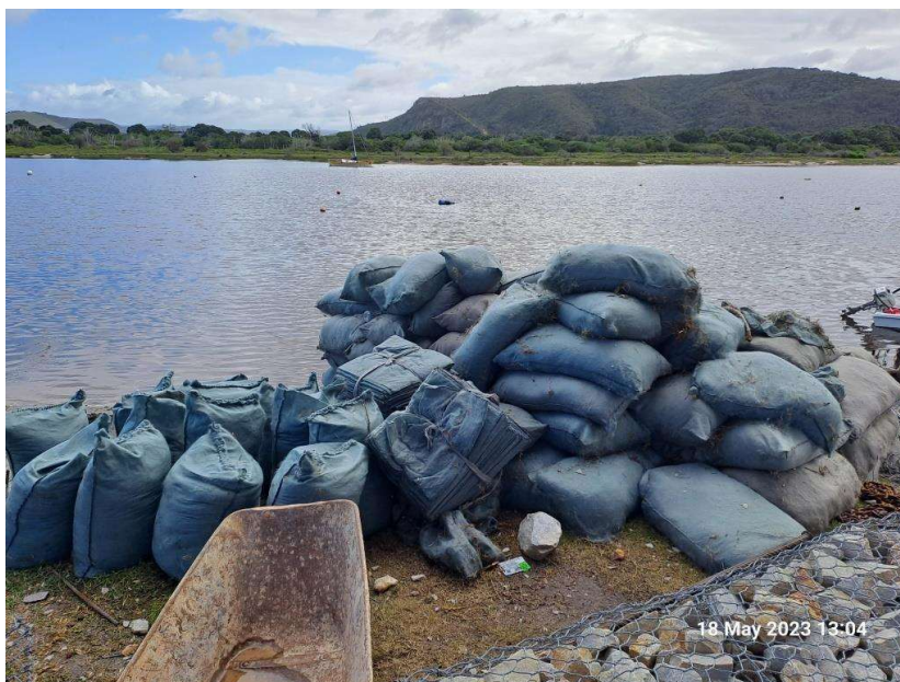
Sandbags being filled from the material which came out of the work area.
