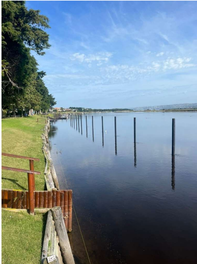
Installation of the 19 poles completed.
