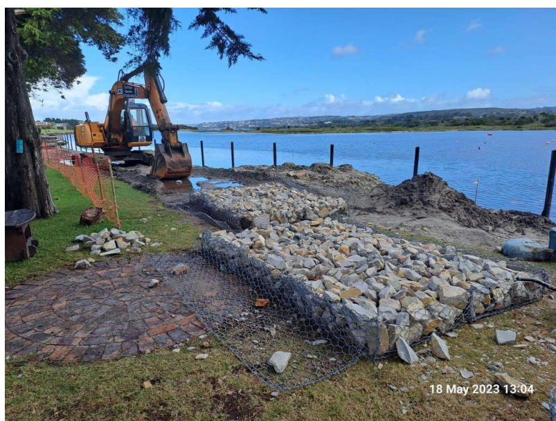
Preparation of reno mattresses
