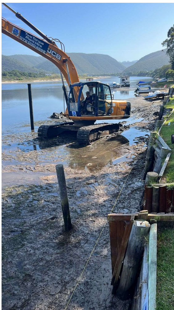
Machine planting the new mooring poles (photo 19 th April 2023)
