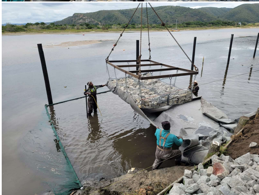
Note the silt curtain in the river on the downstream working edge
