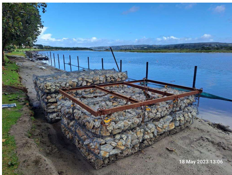
Reno mattresses packed on shore waiting to be lifted into position with the purpose made frame.
