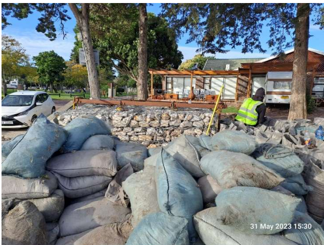
Sandbags being prepared to go onto the slope and be covered by the reno mattresses.
