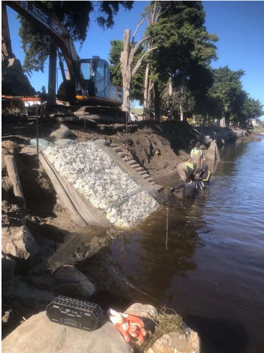
Test section showing the completed profile with the geofabric in place, the reno mattress on the bank with the sand bags behind.
