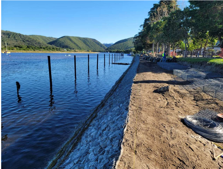
Current state o the site (13 September 2023)
