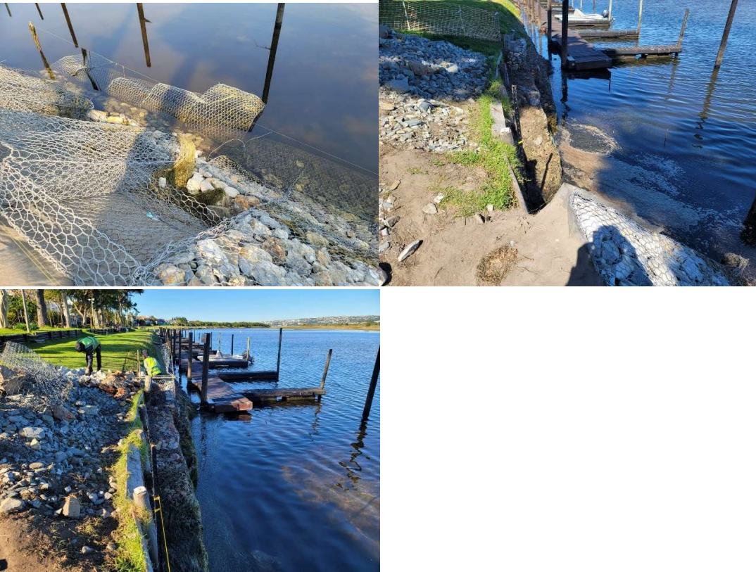
Tie-in with Blue Water in progress (30 August, 7 September and 13 September 2023)
