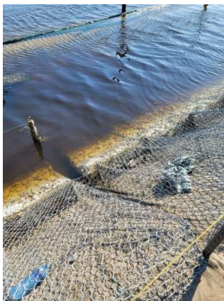
Mooring poles with curtain silt fencing in place when work was still undertaken in the water (11 August 2023)
