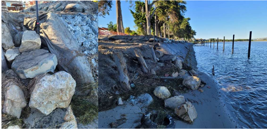
Tie-in progress with SANRAL slipway (13 September 2023)
