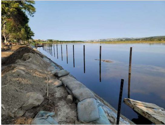
Silt curtain removed as work is restricted to the bank (30 August 2023)
