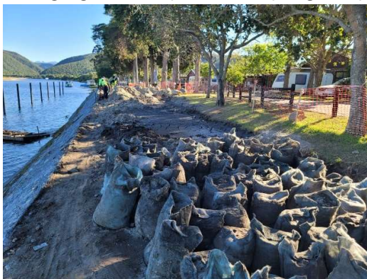
Sandbags being filled (13 September 2023)
