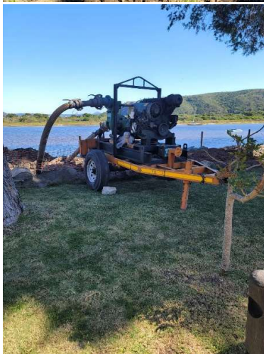
Dredging for compaction in progress (22 August & 7 September 2023)
