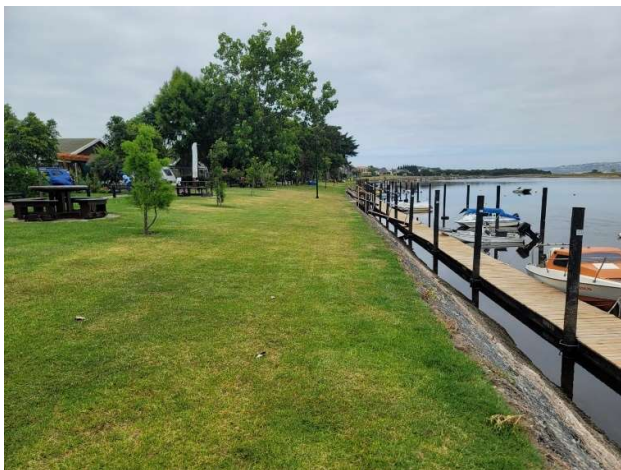
Installation of fingers in process
