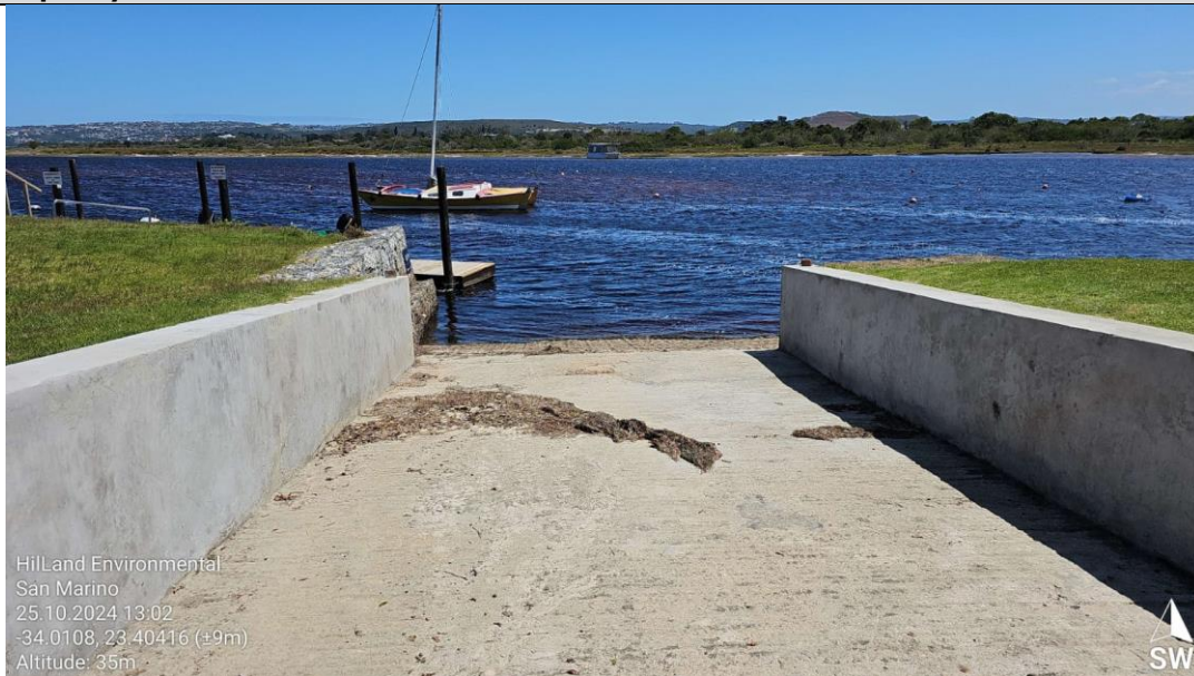
Riparian zone rehabilitation
