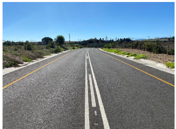
Condition of Protea Road, successfully resurfaced.
