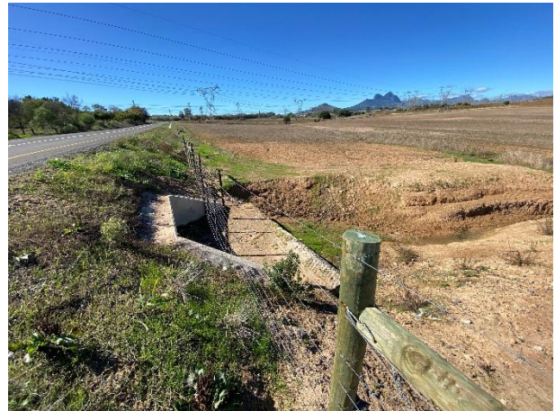
Stormwater outlet structure successfully installed.
