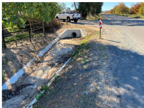
Installed stormwater side drains.
