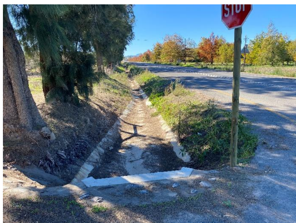
Installed stormwater side drains.
