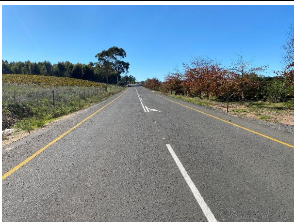
Condition of Protea Road, successfully resurfaced.
