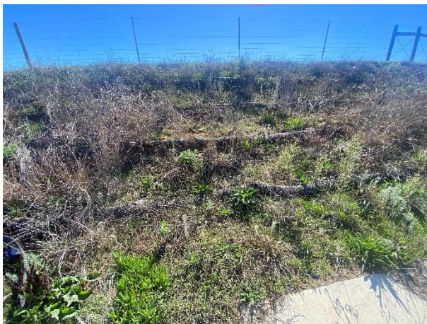
Revegetation established along rehabilitated roadside embankment slopes.
