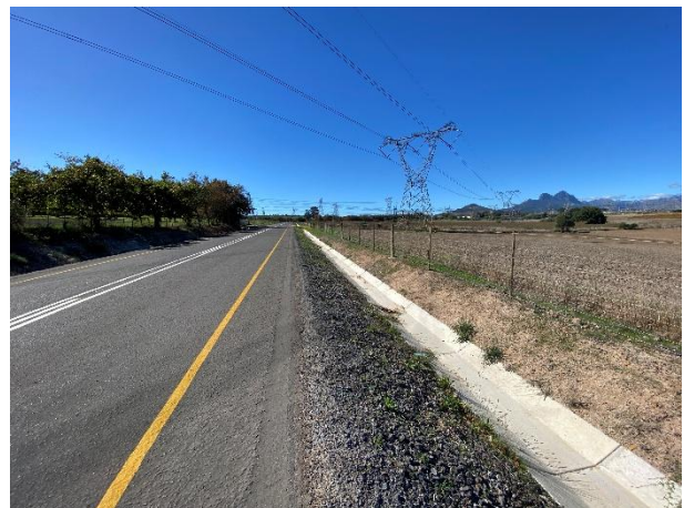
Stormwater side drains installed along the road reserve.
