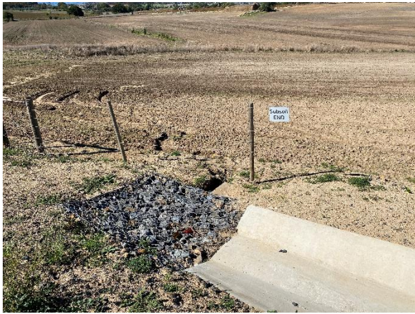
Gabion mattress installed.
