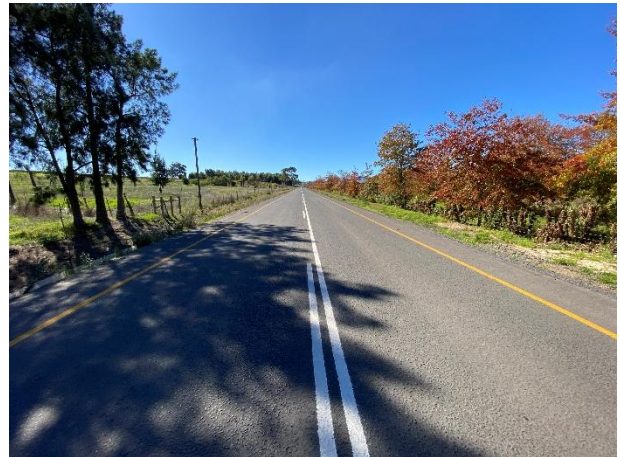
Condition of Protea Road, successfully resurfaced.
