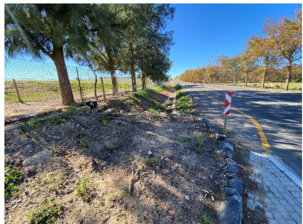
Rehabilitation of the road reserve in progress.
