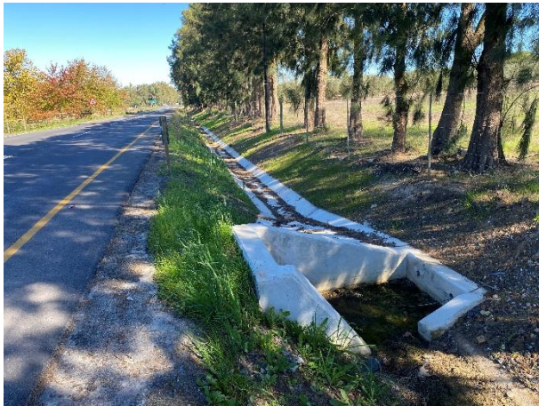
Installed stormwater side drains and inlet structure.
