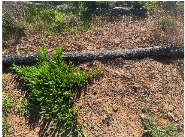
Revegetation established along rehabilitated roadside embankment slopes.
