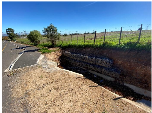
Excavated stormwater side drain channels successfully installed with gabion retaining walls.
