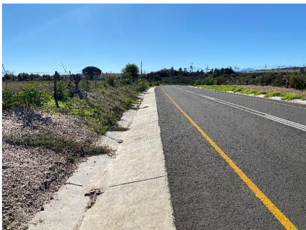
Installed stormwater side drains.
