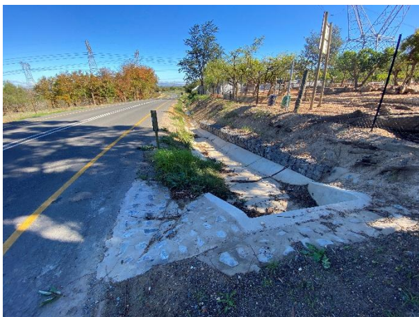
Stormwater side drains installed along the road reserve as seen towards the west.
