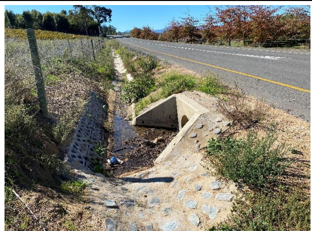
Stormwater outlet structure successfully installed.
