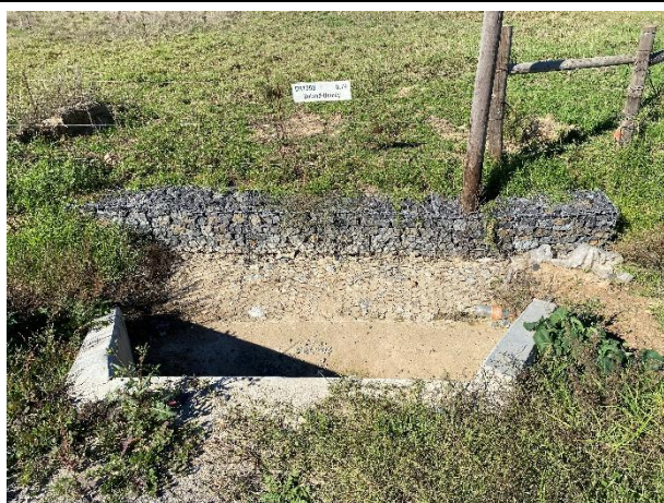
Newly upgraded stormwater culvert.
