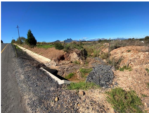
Upgraded stormwater outlet structure with installed gabion mattresses.
