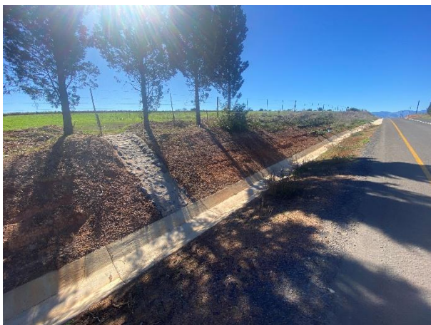
Recently constructed concrete-lined roadside stormwater drainage channel and slope stabilisation.
