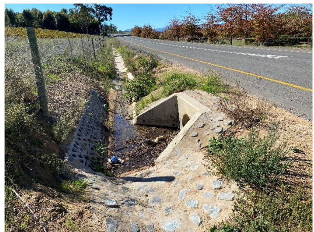
Stormwater outlet structure successfully installed.
