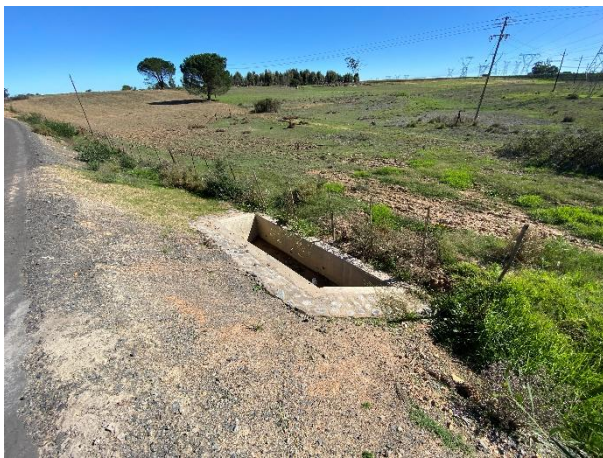
Stormwater inlet structure successfully installed.
