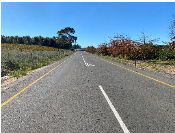
Condition of Protea Road, successfully resurfaced.
