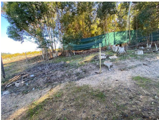
Reinstated fencing along the development route.
