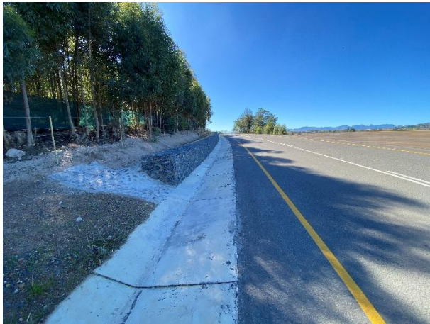
Installed gabion retention wall along the previous cuttings along the Protea Road.
