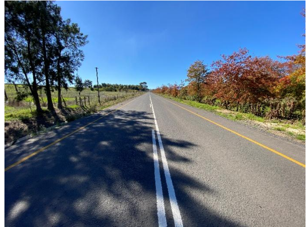
Condition of Protea Road, successfully resurfaced.
