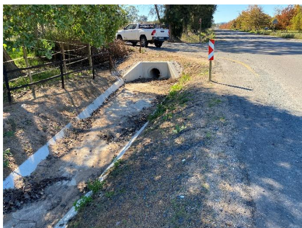
Installed stormwater side drains.
