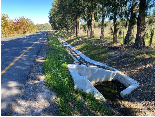
Installed stormwater side drains and inlet structure.
