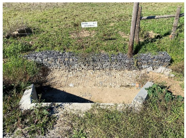
Newly upgraded stormwater culvert.
