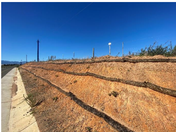
Hessian sausage erosion controls installed for roadside slope rehabilitation.
