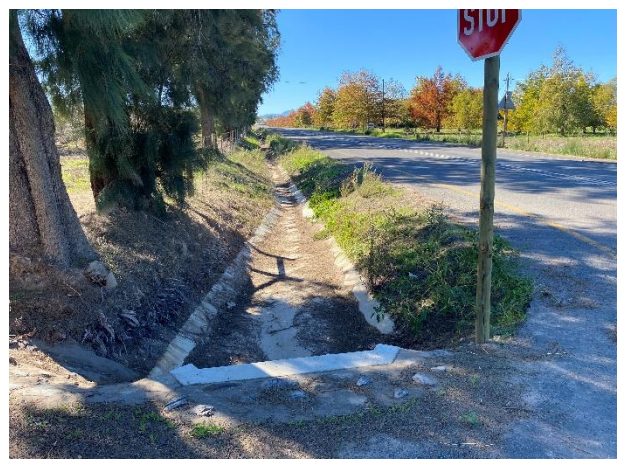
Installed stormwater side drains.
