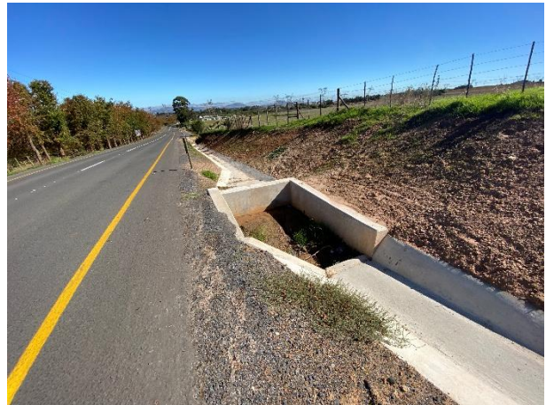
Upgraded stormwater inlet structure.
