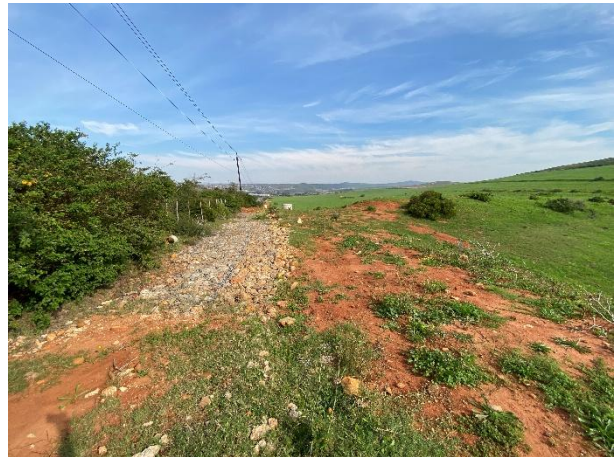
Installation of gabion mattresses along the pipeline route.
