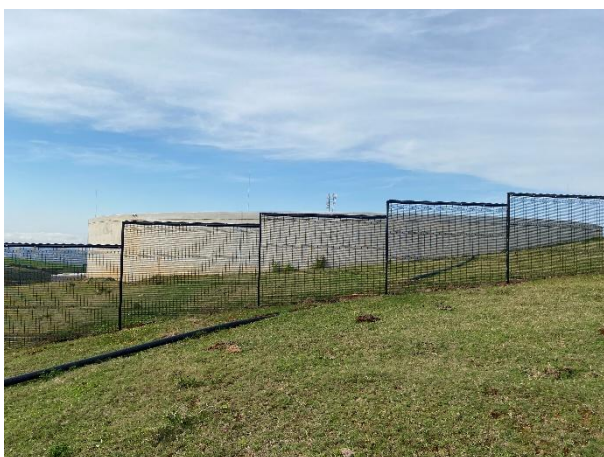
Existing 7 Ml reservoir fully fenced with ClearVu fencing as seen towards the southeast.
