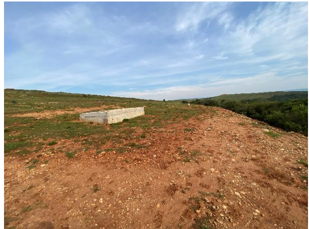
Installed gravity pipeline network and associated infrastructure towards the southwest.
