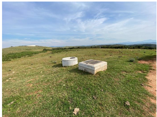
Installed gravity pipeline network and associated manhole infrastructure towards the northwest.
