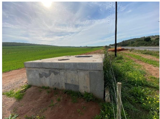
Installed gravity pipeline network and associated infrastructure along the R102 towards the southeast.
