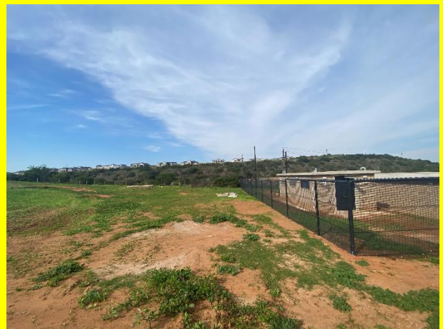
Hydroseeding surrounding the pump station in progress, minor builders' rubble to be removed.
