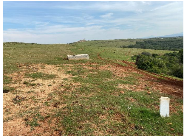
Installed gravity pipeline network and associated infrastructure towards the 1 Ml reservoir servicing Monte Christo Retirement Village.
