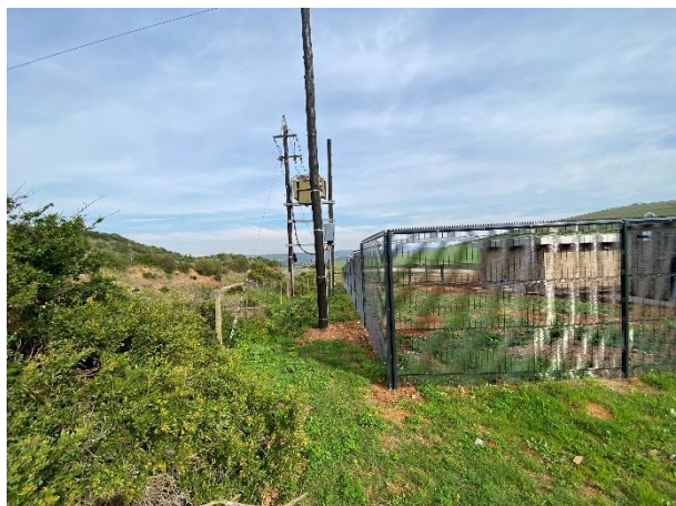
Condition of the constructed pump station along the R102 towards the south
