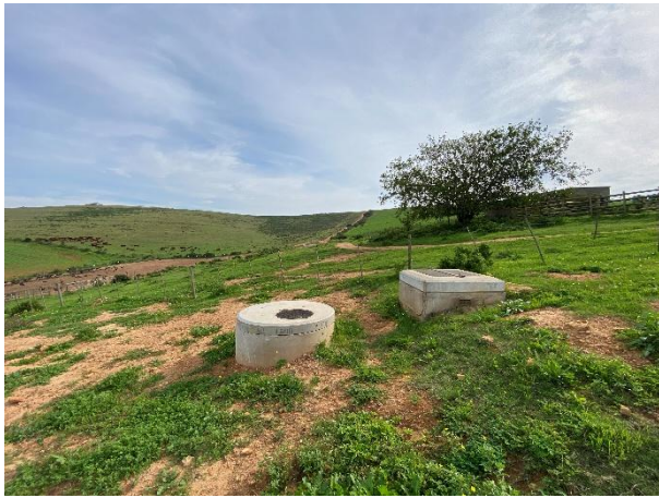
Installed gravity pipeline network and associated manhole infrastructure adjacent to the farm shed.
