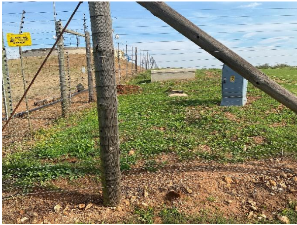
Fencing in place surrounding the 1 Mℓ reservoir servicing Monte Christo Retirement Village.
