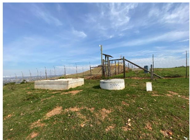
Installed gravity pipeline network and associated infrastructure towards the 1 Ml reservoir.
