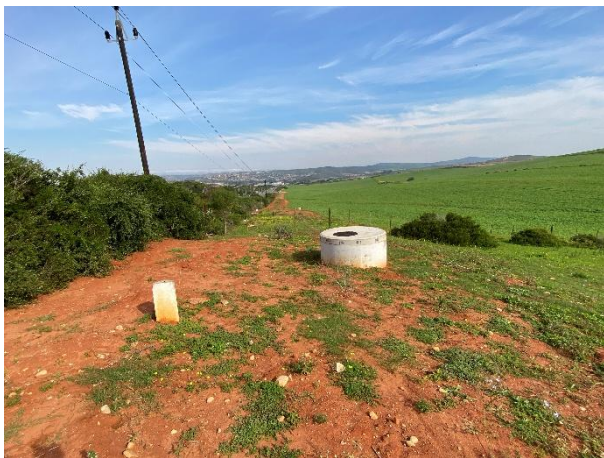
Installed gravity pipeline network and associated manhole infrastructure along the R102 towards the southwest.
