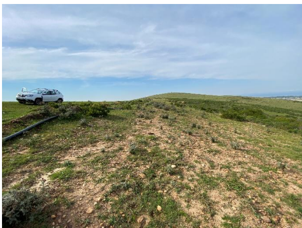
Installed gravity pipeline network and associated infrastructure towards the southeast.
