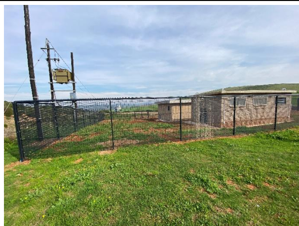
Condition of the constructed pump station and fencing along the R102 towards the south.
