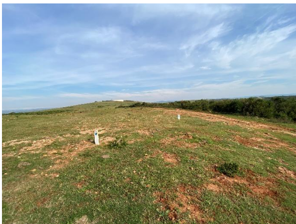
Installed gravity pipeline network towards the southwest, natural vegetation along the western boundary intact.
