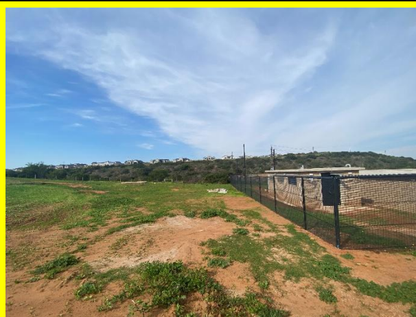
Hydroseeding surrounding the pump station in progress, minor builders' rubble to be removed.
