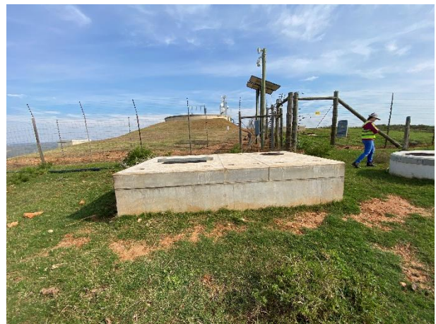
Installed gravity pipeline network and associated infrastructure towards the 1 Mℓ reservoir.
