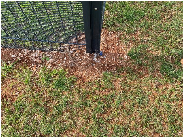
Surveyor peg for the fence installation.
