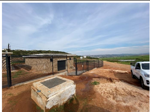
Pump station has been fully fenced in with ClearVu fencing.
