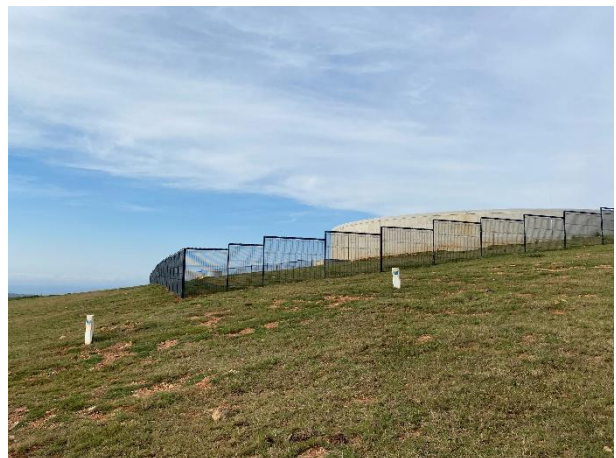
Connection of the gravity-fed pipeline network to the existing 7 Ml reservoir as seen towards the southwest.
