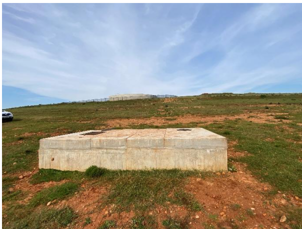
Condition of the associated potable water network infrastructure towards the southwest.
