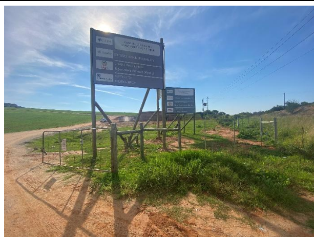
Signage in place at the entrance of the site off the R102.
