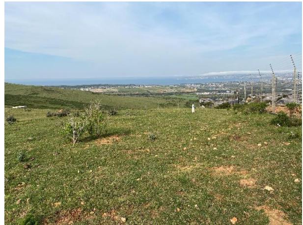
Installed gravity pipeline network connection from the 1 Mℓ reservoir towards the southeast.
