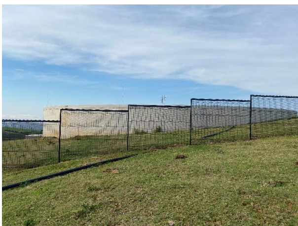
Existing 7 Ml reservoir fully fenced with ClearVu fencing as seen towards the southeast.
