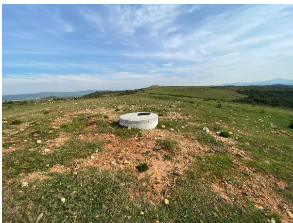
Installed gravity pipeline network and associated infrastructure towards the 1 Ml reservoir
