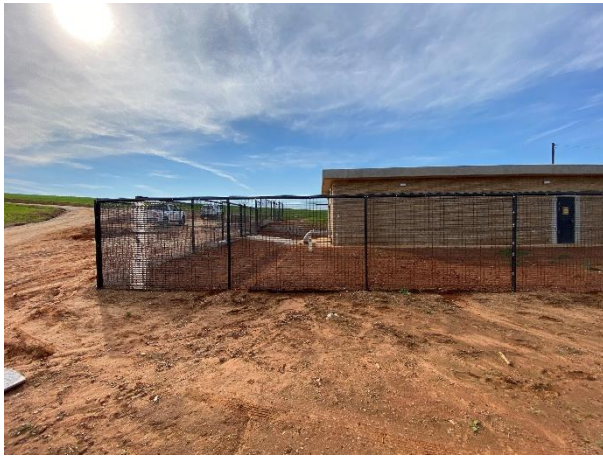
Condition of the constructed pump station and fencing as seen towards the northeast.
