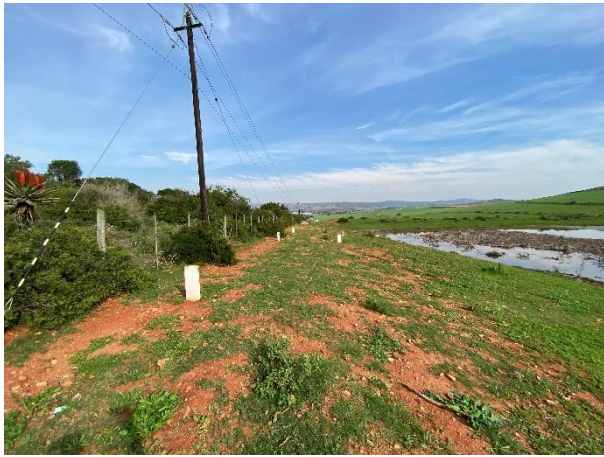
Installed gravity pipeline network along the R102 towards the southwest. Adequate vegetation regrowth.
