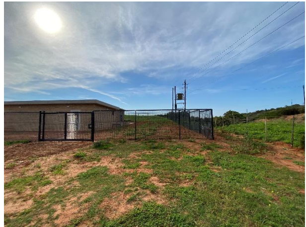
Condition of the constructed pump station and fencing along the R102 towards the north.
