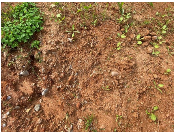
Hydroseeding within the pump station completed.
