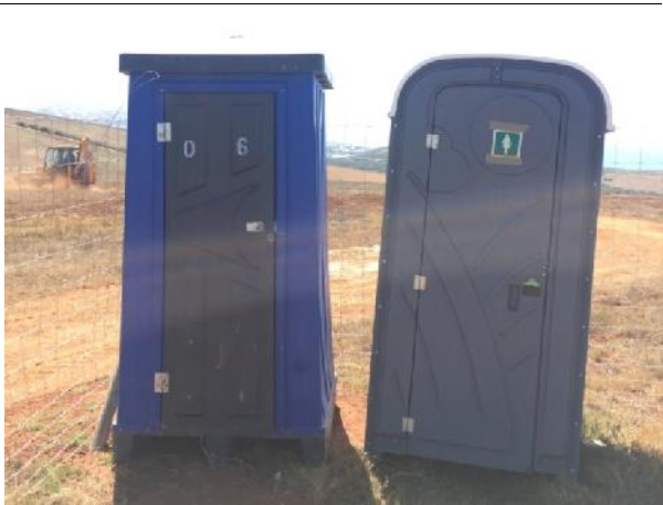
2021.02.10 – On-site ablution facilities
