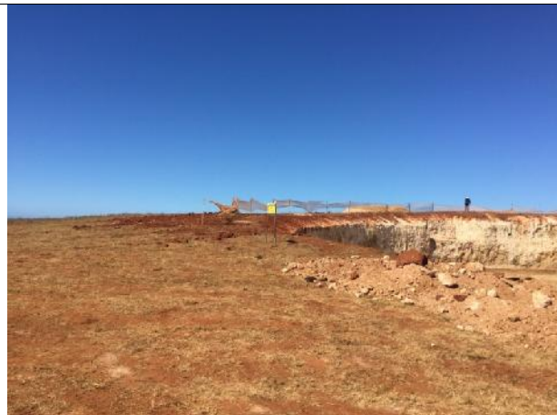
2021.02.10 – The orange netting is only installed on the southern edge, where the deepest excavated area is.
