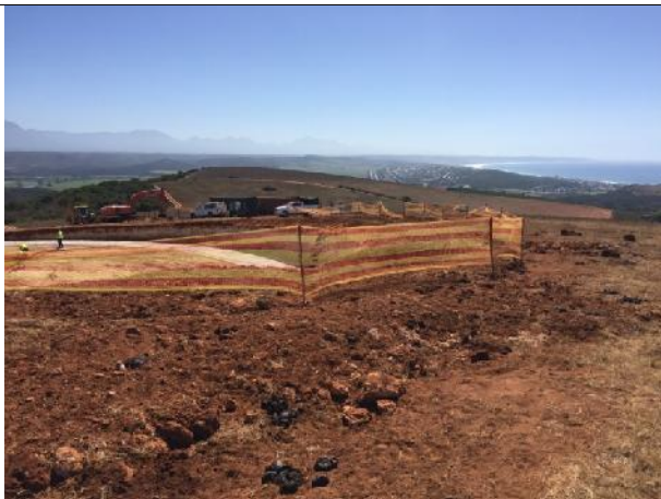
2021.02.10 – The No-Go demarcation at the top of the excavation area on the Southern edge of the reservoir.
