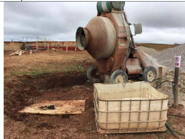
2021.03.17 – Concrete mixing area
