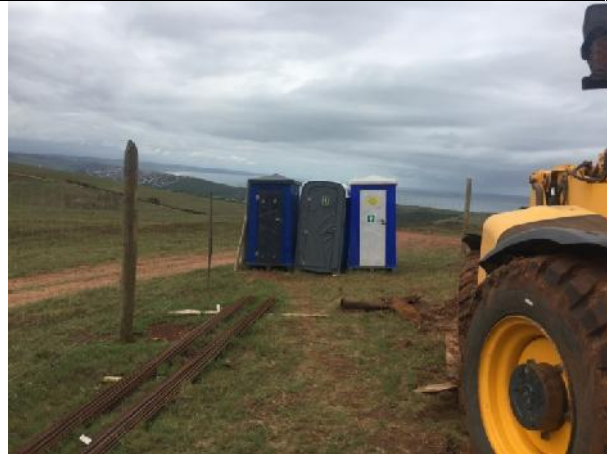
2021.03.17 – On-site ablution facilities
