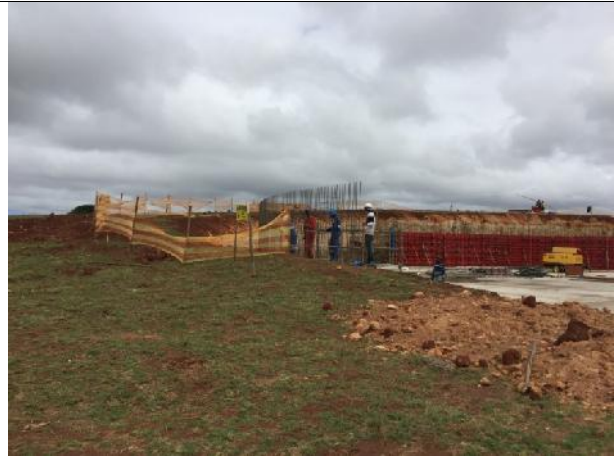
2021.03.17 – The orange netting is only installed on the southern edge, where the deepest excavated area is.
