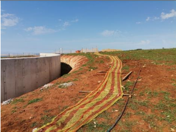
2021.04.21 – The No-Go demarcation around the excavation area is removed during the day. The fence MUST be in place during inactive construction periods.
