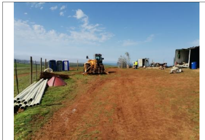
2021.04.21 – Site camp is kept neat and tidy
