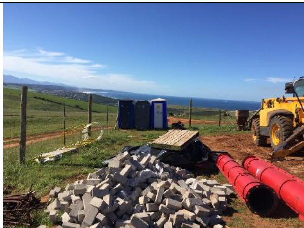
2021.05.12 – Site camp is kept neat and tidy.
