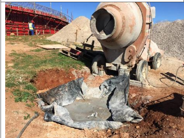
2021.05.12 – The concrete mixing area is contained.
