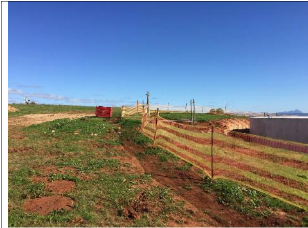
2021.05.12 – The demarcation around the excavation area is in place. The fence MUST be in place during inactive construction periods.
