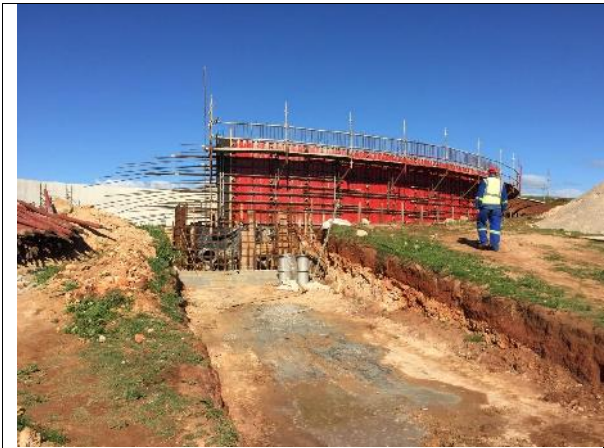
2021.05.12 – cement run-off water catch pit.
