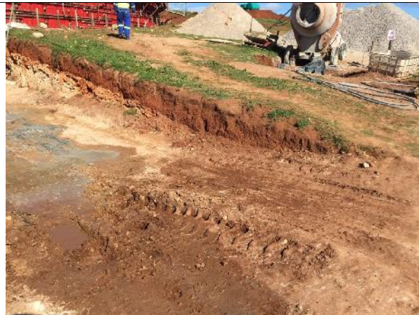
2021.05.12 – cement run-off water catch pit.
