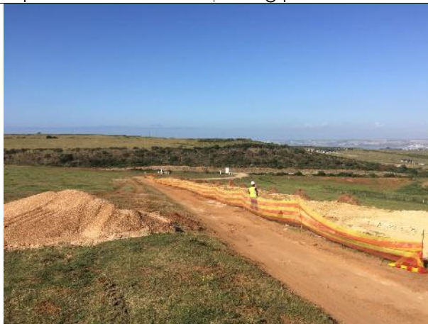
2021.06.09 – No-Go demarcation in place – it is recommended that both side of the trench must be demarcated to prevent the farm animals from entering the site.
