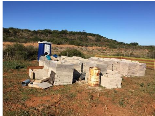
2021.06.17 – Ablution facilities located at the pump station construction area.
