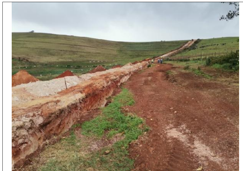
2021.06.23 – The subsoil is stockpiled to the left of the trench and the topsoil is stockpiled further left, next to the subsoil stockpile.
