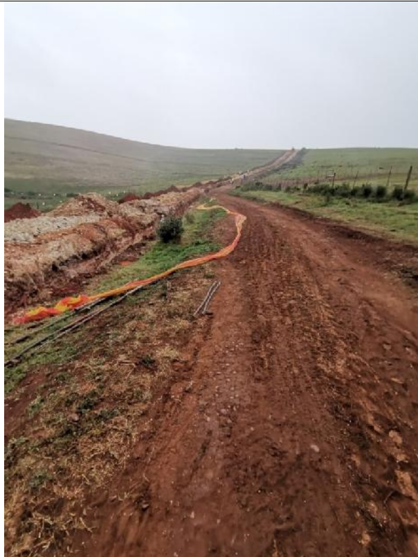
2021.06.23 – The access road on the right-hand side of the trench.
