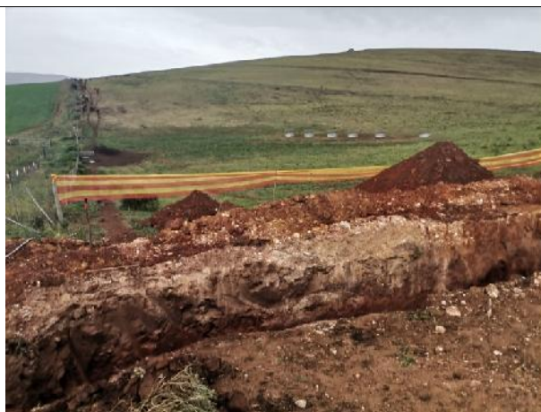
2021.06.23 – The orange netting is installed along parts of the western side of the trench.
