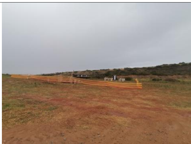
2021.06.23 – The No-Go demarcation around the construction of the pump station.
