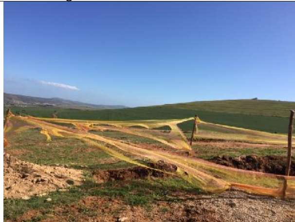
2021.08.11 – The orange netting must be fully upright – especially when there are cattle in the same camp.
