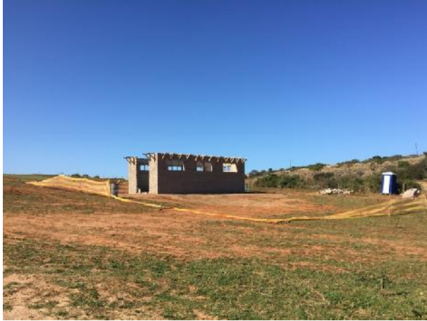
2021.08.11 – The contractor is reminded that the orange netting must be fully upright when not working in that area.
