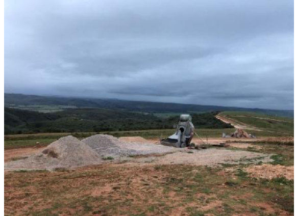
2021.09.27 – Concrete mixing areas is bunded to prevent cement water run-off.
