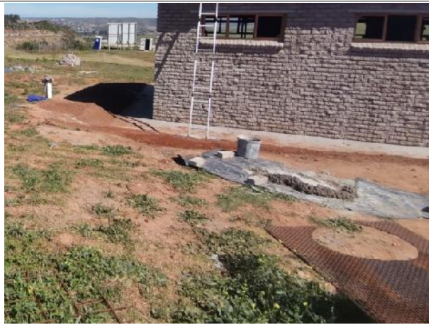
2021.09.08 – Cement is mixed on a non-permeable plastic layer.
