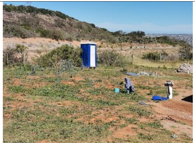
2021.09.09 – Ablution facilities for the staff at the pumpstation.
