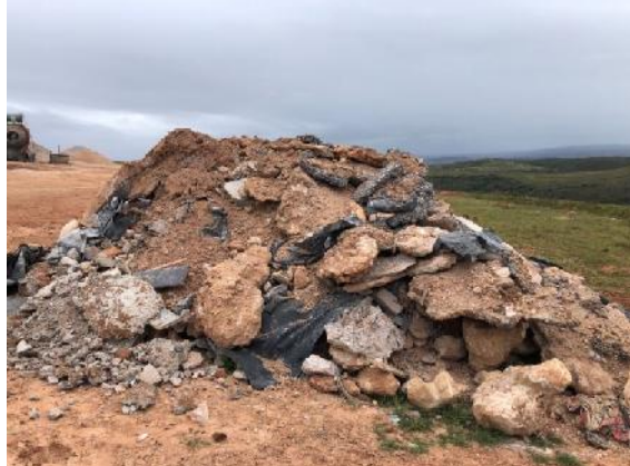
2021.09.27 – The contractor is reminded that paper/plastic must be kept separate from construction rubble.
