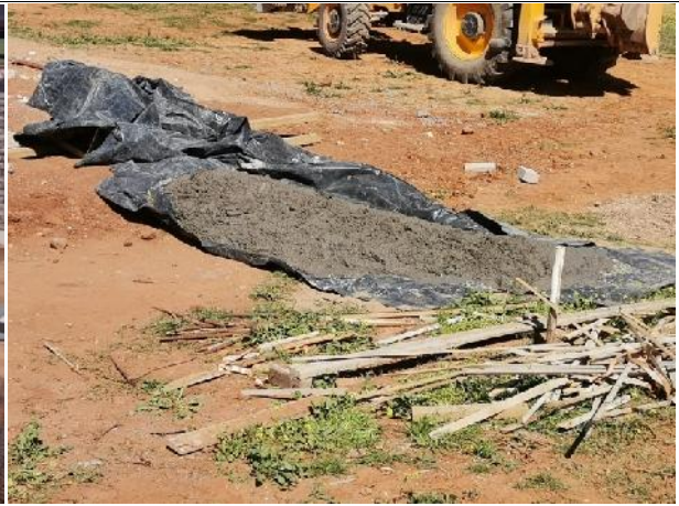
2021.09.08 – Cement is mixed on a non-permeable plastic layer.
