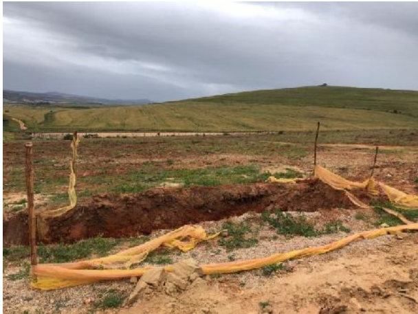
2021.09.27 - Demarcation must be always maintained and in good condition.
