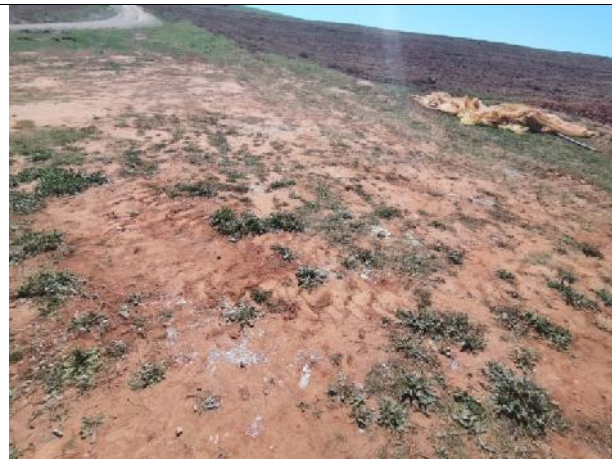
2021.09.08 – Cement spills must be cleaned up daily.
