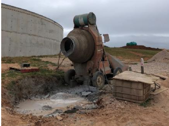
2021.09.27 – Concrete mixing areas is bunded to prevent cement water run-off.
