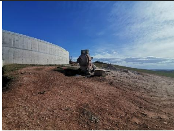
2021.10.22 – Concrete mixing areas is bunded to prevent cement water run-off.
