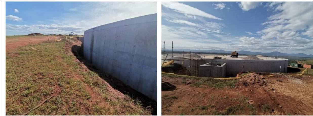
2021.10.22 – The demarcation netting is in place. The contractor must ensure that it is maintained and fully upright before leaving the site each day.
