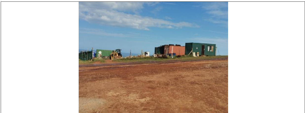
2021.10.22 – Adequate litter bins and ablution facilities are available at the site camp.
