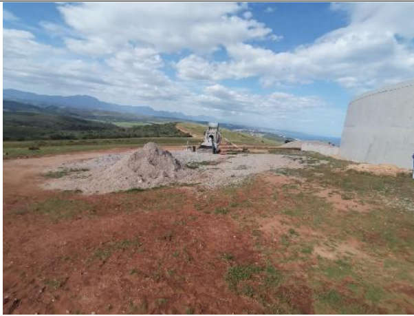
2021.10.22 – Concrete mixing areas is bunded to prevent cement water run-off.
