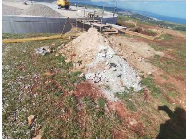
2021.10.22 – The contractor is reminded that paper/plastic must be kept separate from construction rubble.
